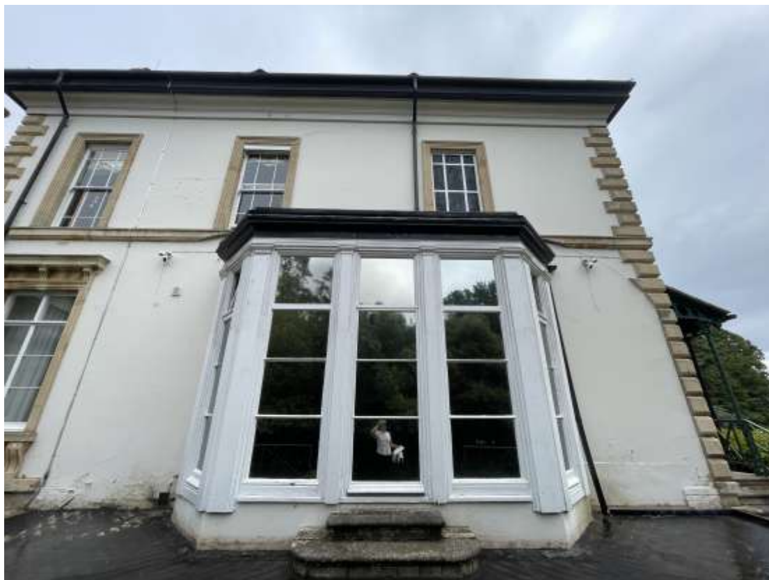
Stone quoins and string to rear elevation of ground floor evidently scribed around the now demolished conservatory.
