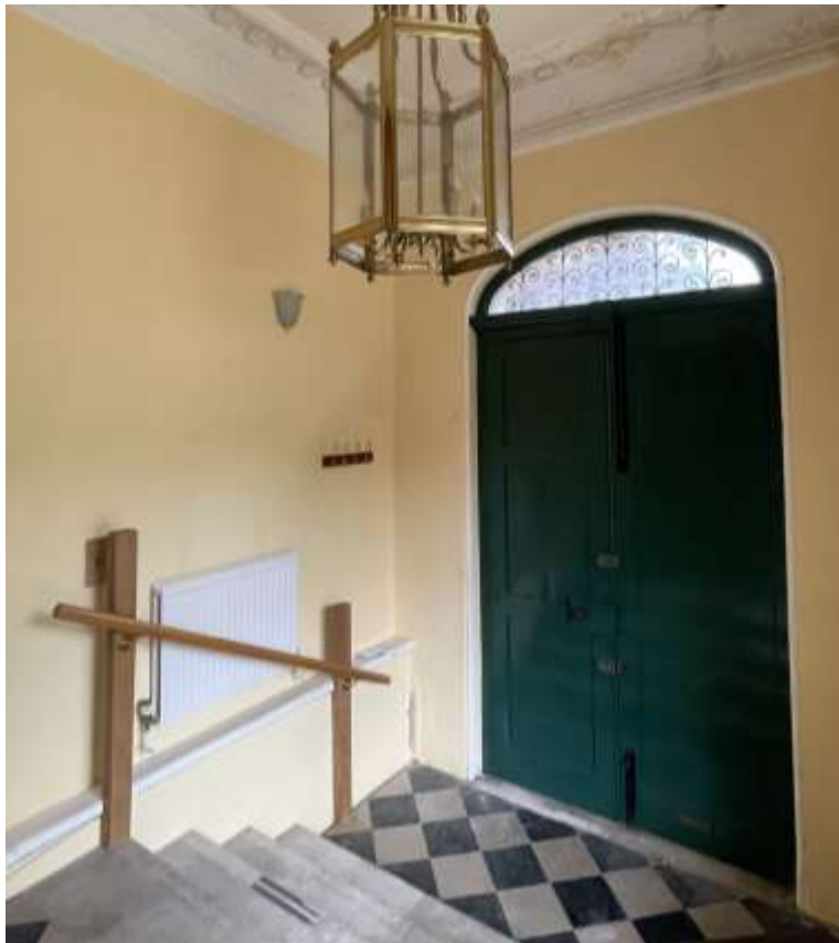
Existing entrance lobby on other side of kitchen.
