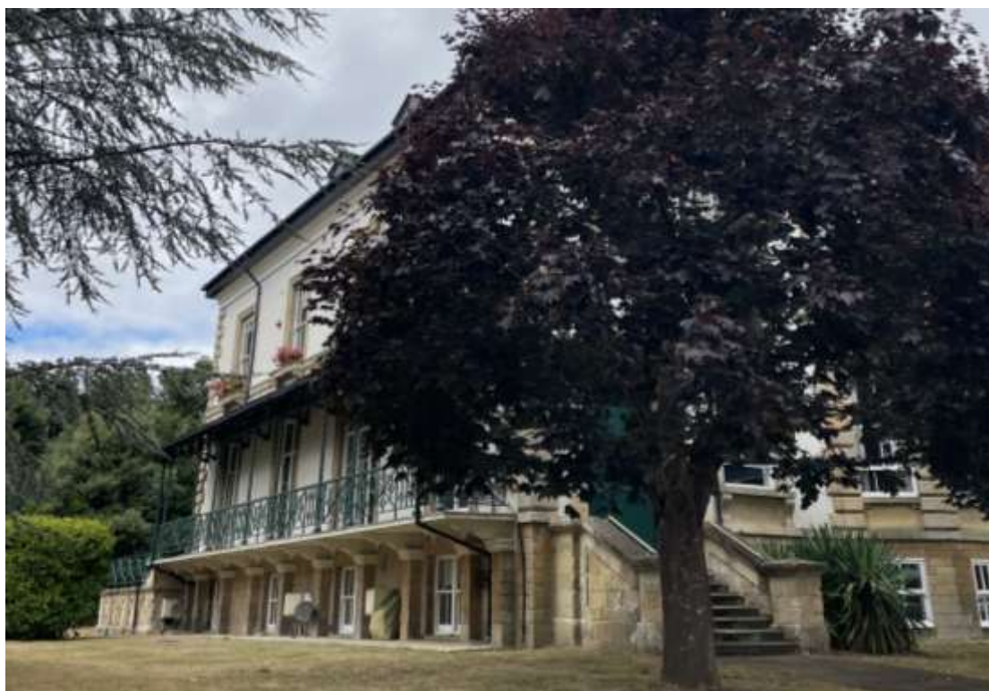
Verandah staircase removed and cast iron balustrade repaired.
