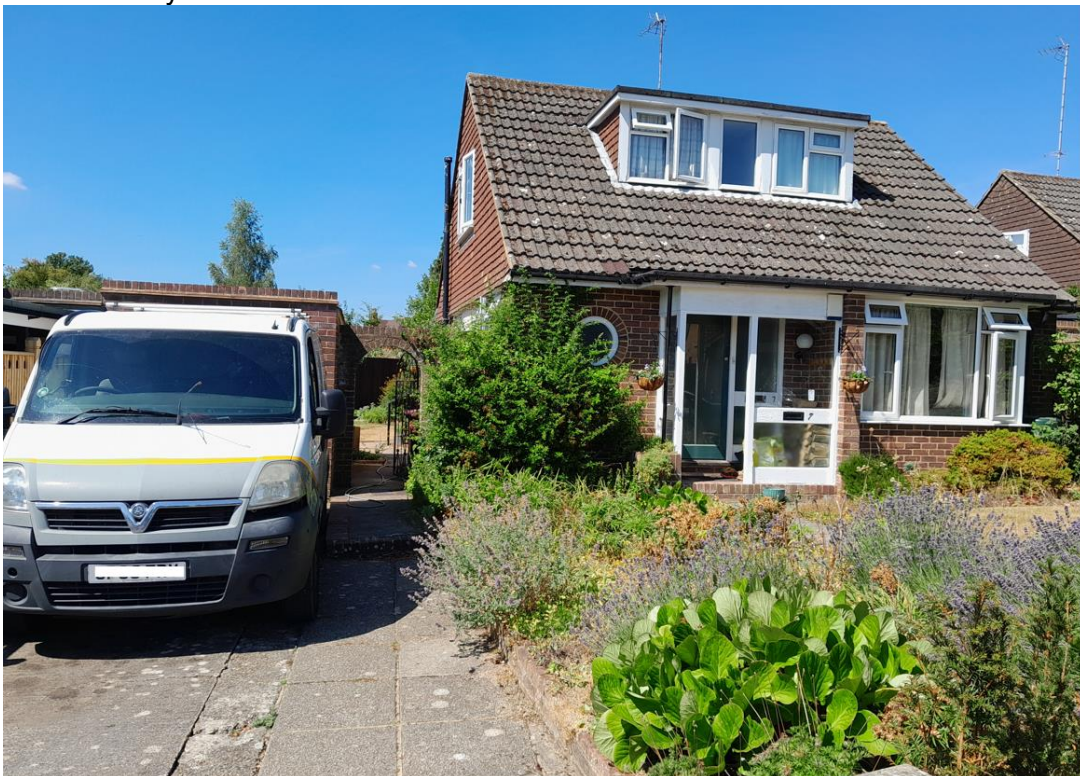
Existing front elevation, with front garden, driveway parking and garage to side (behind van).
