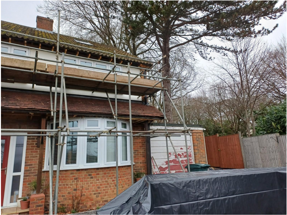
Site Visit Photos taken on 11 December 2024
