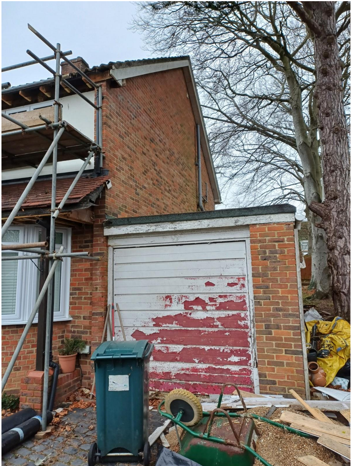
Site Visit Photos taken on 11 December 2024
