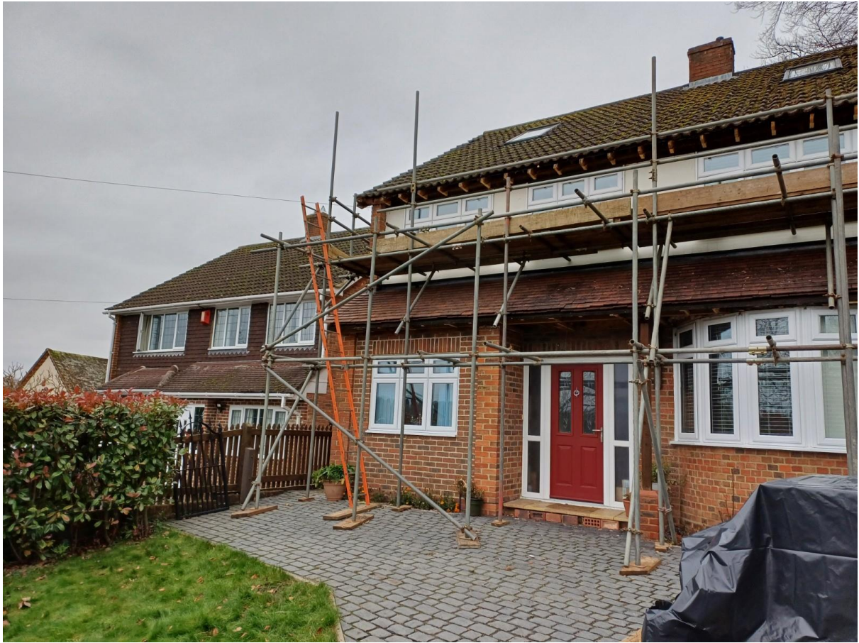
Site Visit Photos taken on 11 December 2024
