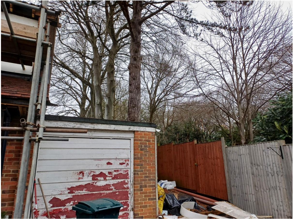
Site Visit Photos taken on 11 December 2024
