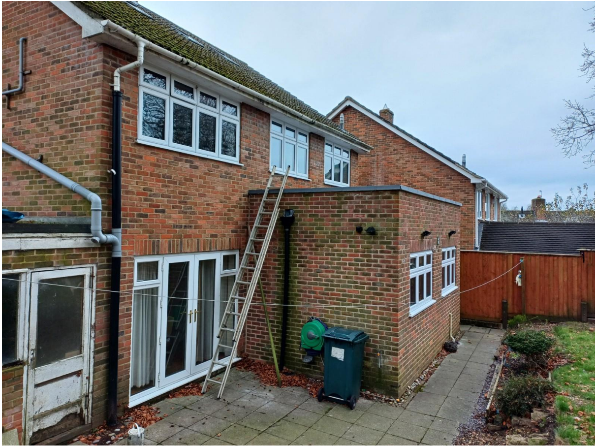
Site Visit Photos taken on 11 December 2024
