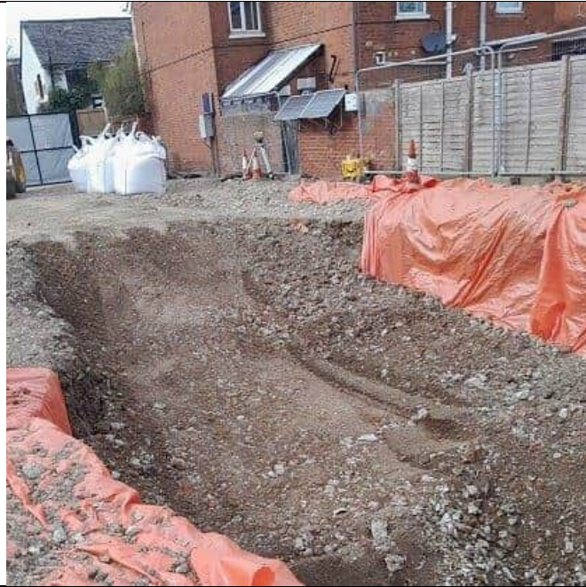
Photograph 4: membrane being implemented within the service corridors.
