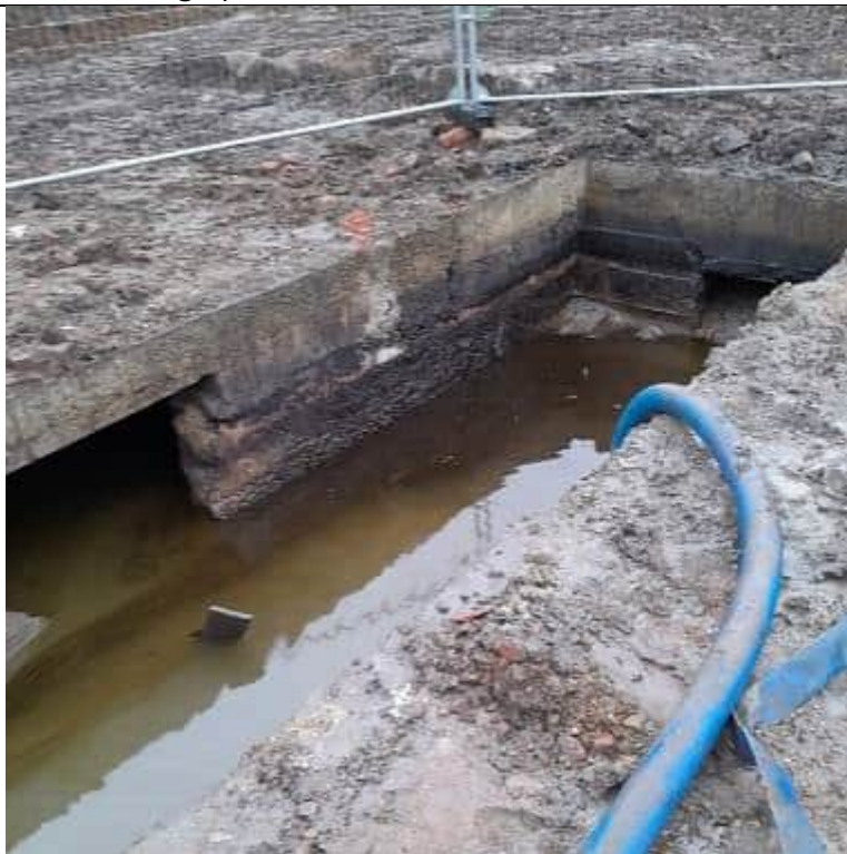
Photograph 2: Pumping of waste water on site
