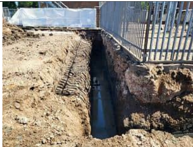
Photograph 5: Cut off trench, dug out.
