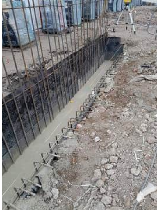
Photograph 6: Trench installed with membrane and backfilled with concrete.
