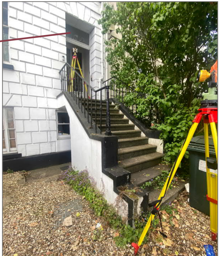
Image 17: View of entrance steps and balustrade 109 Castle Hill, Reading
