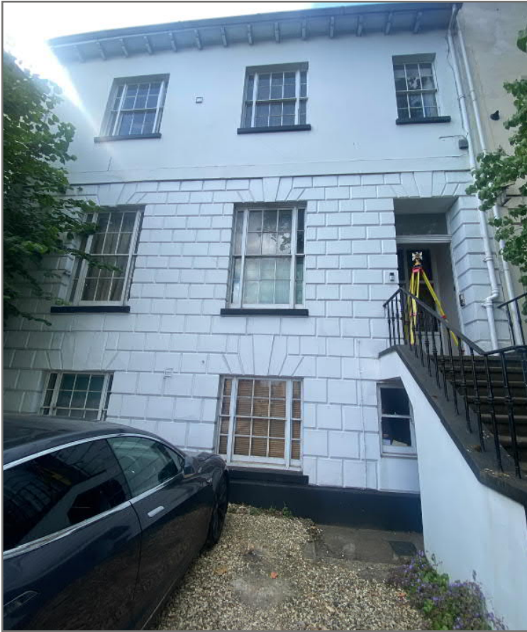
Image 14: View of north elevation with rusticated 'base' (Semi-Basement and raised Ground Floor)
