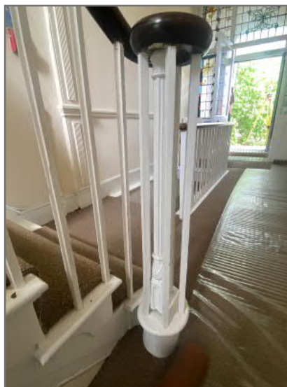
Image 19: Curtil step with a cluster of square profile balusters supporting it; open-string staircase
