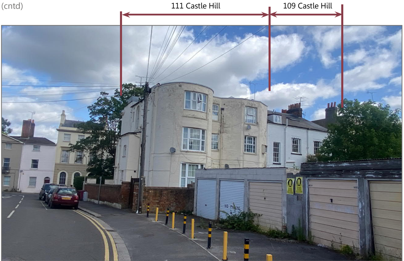
Image 16: View from Field Road
