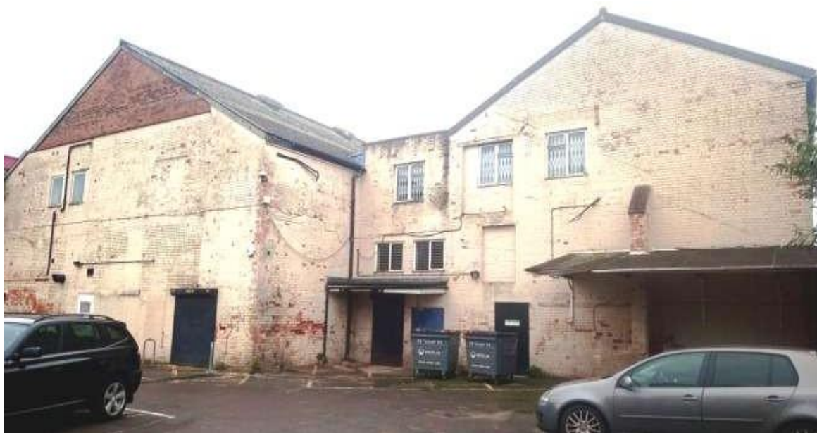
Fig 2.2.4: West end of building from the southwest (71 right)
