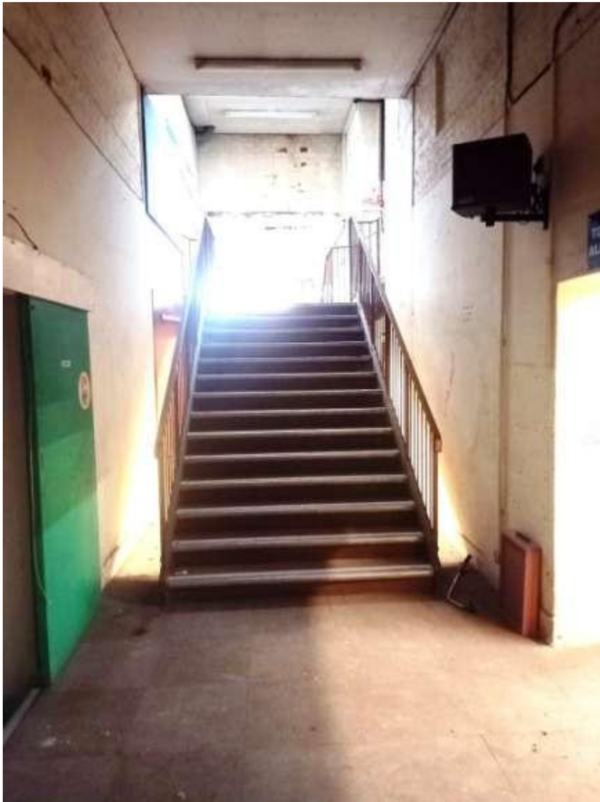
Fig 4.2: Front stairs from ground floor to mezzanine landing in infill block
