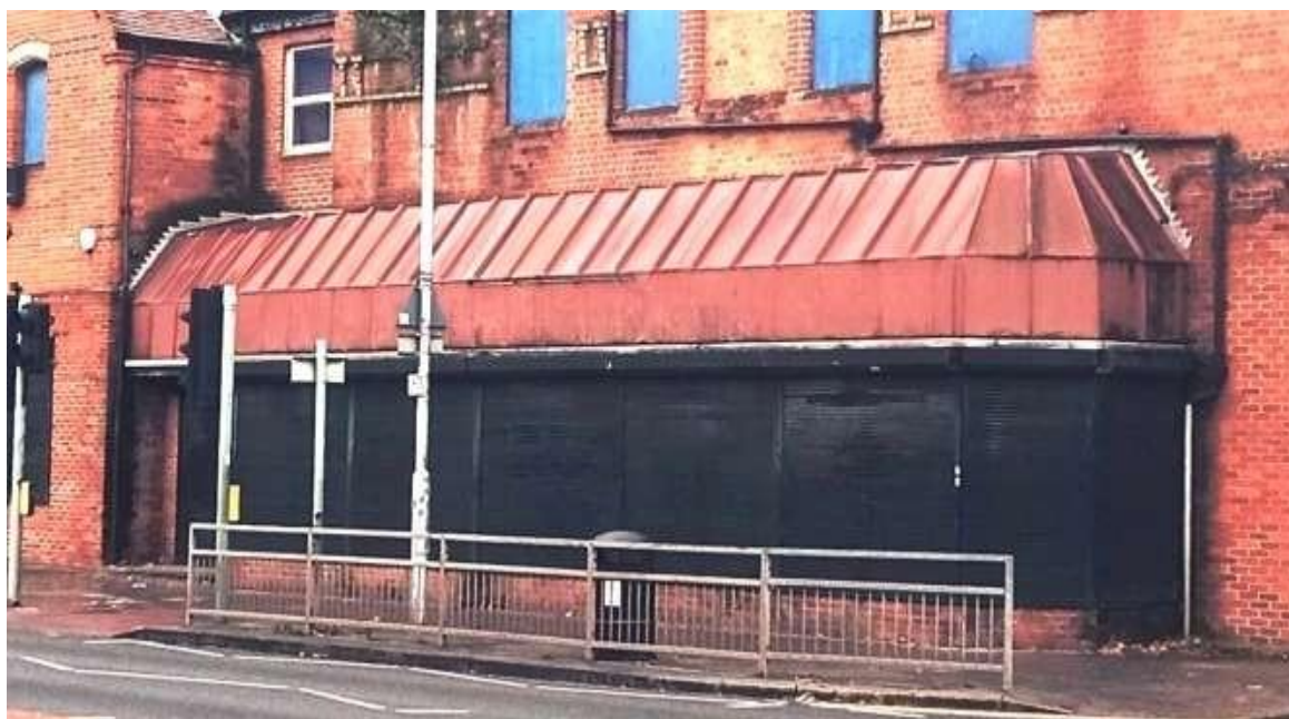
Fig 3.1.8: Shop front canopy
