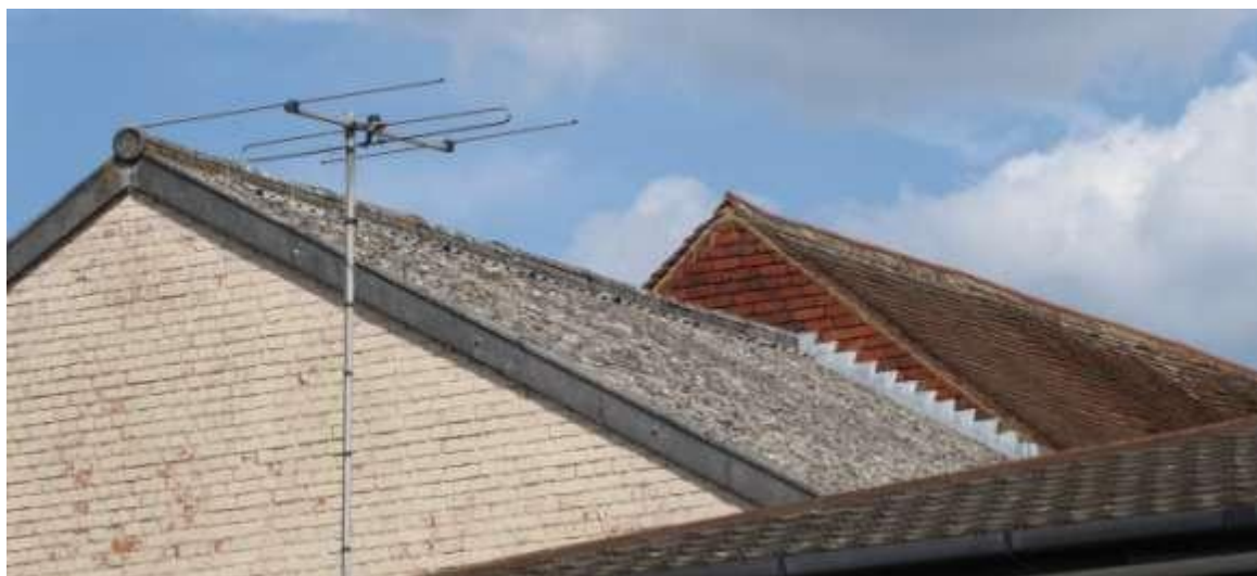
Fig 3.1.7: Rear south block roof
