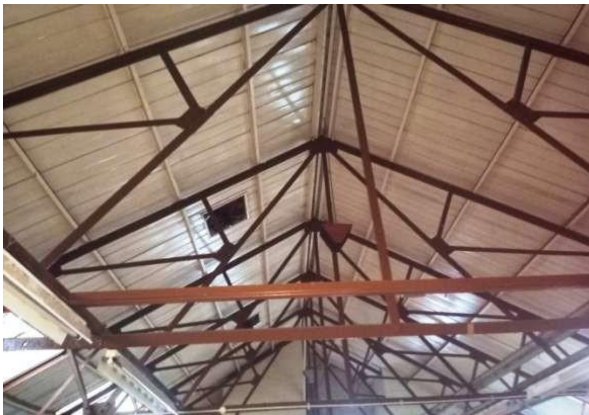
Fig 4.5.4: Roof trusses to north block man roof
