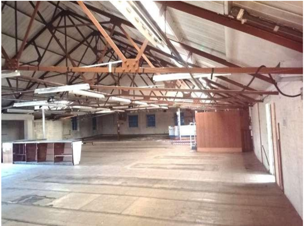
Fig 4.5: North block first floor looking towards the front
