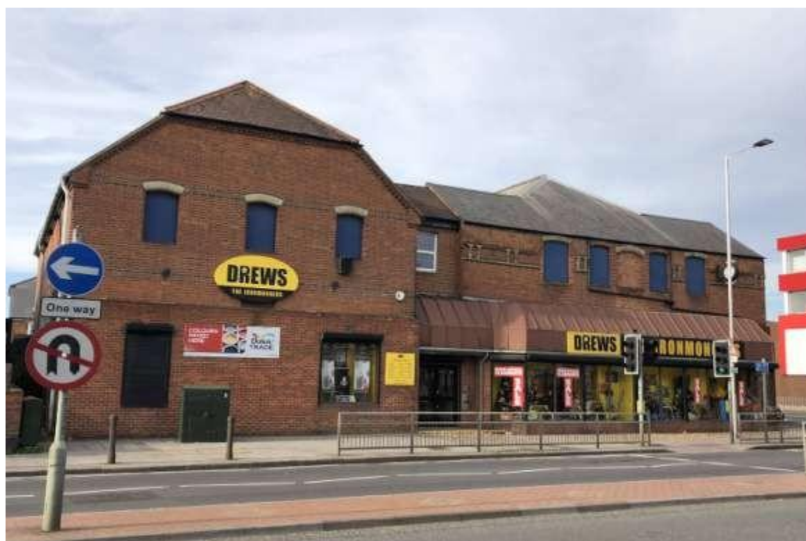
Fig 6.2.8: Frontage to Caversham Road at the time of Drews" closure
