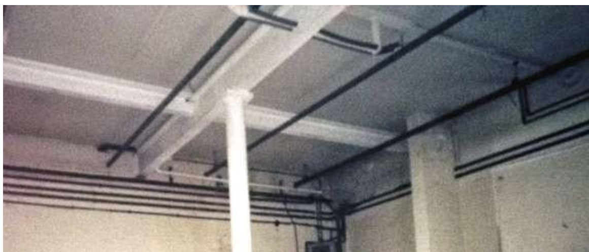
Fig 4.4.3: Support to underside of upper floor
