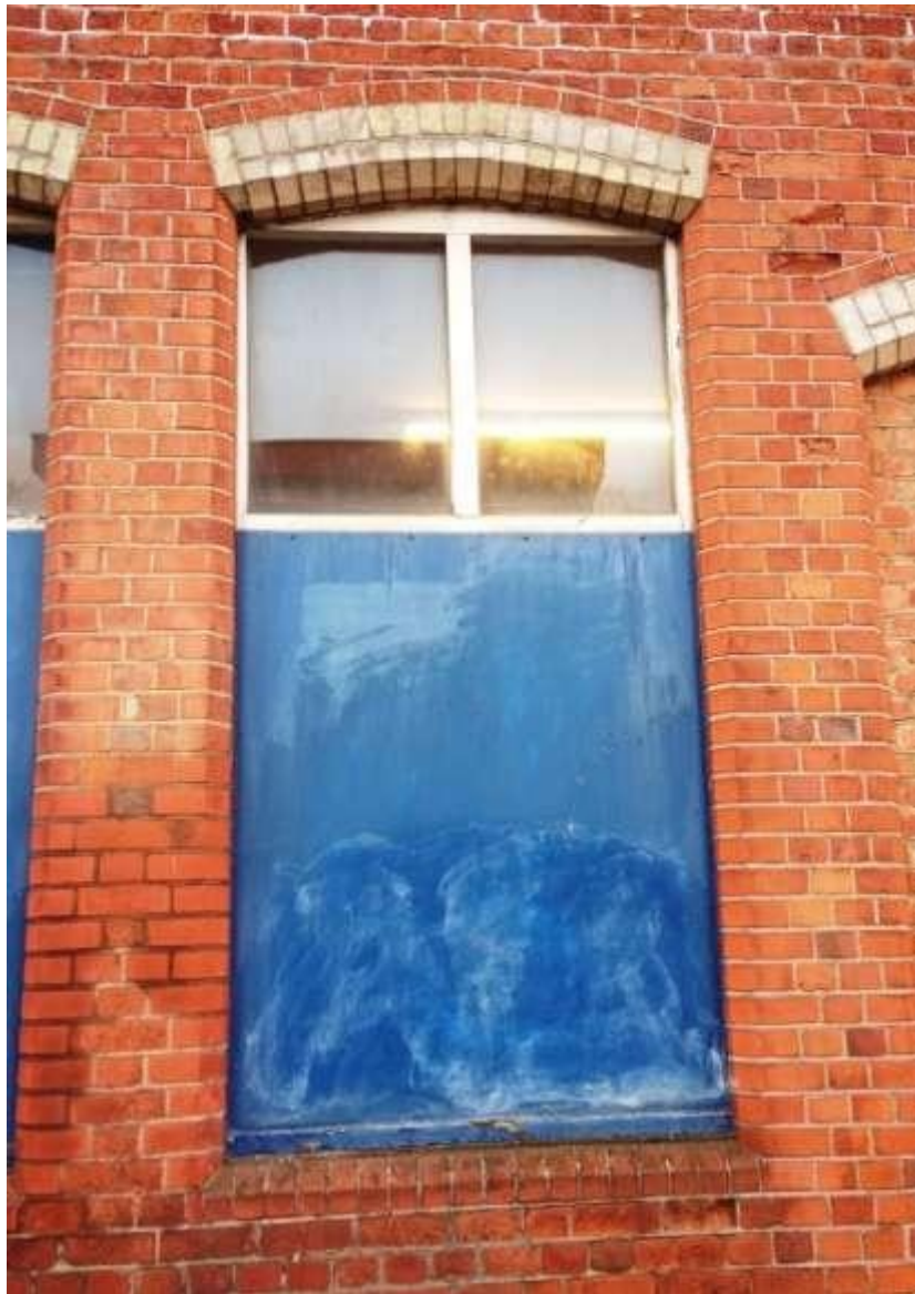
Fig 3.3.2: Ground floor window
