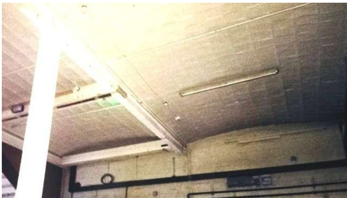
Fig 4.3.4: Underside of brick upper floor
