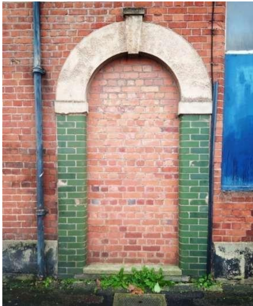
Fig 3.3.4: Closed-up door opening
