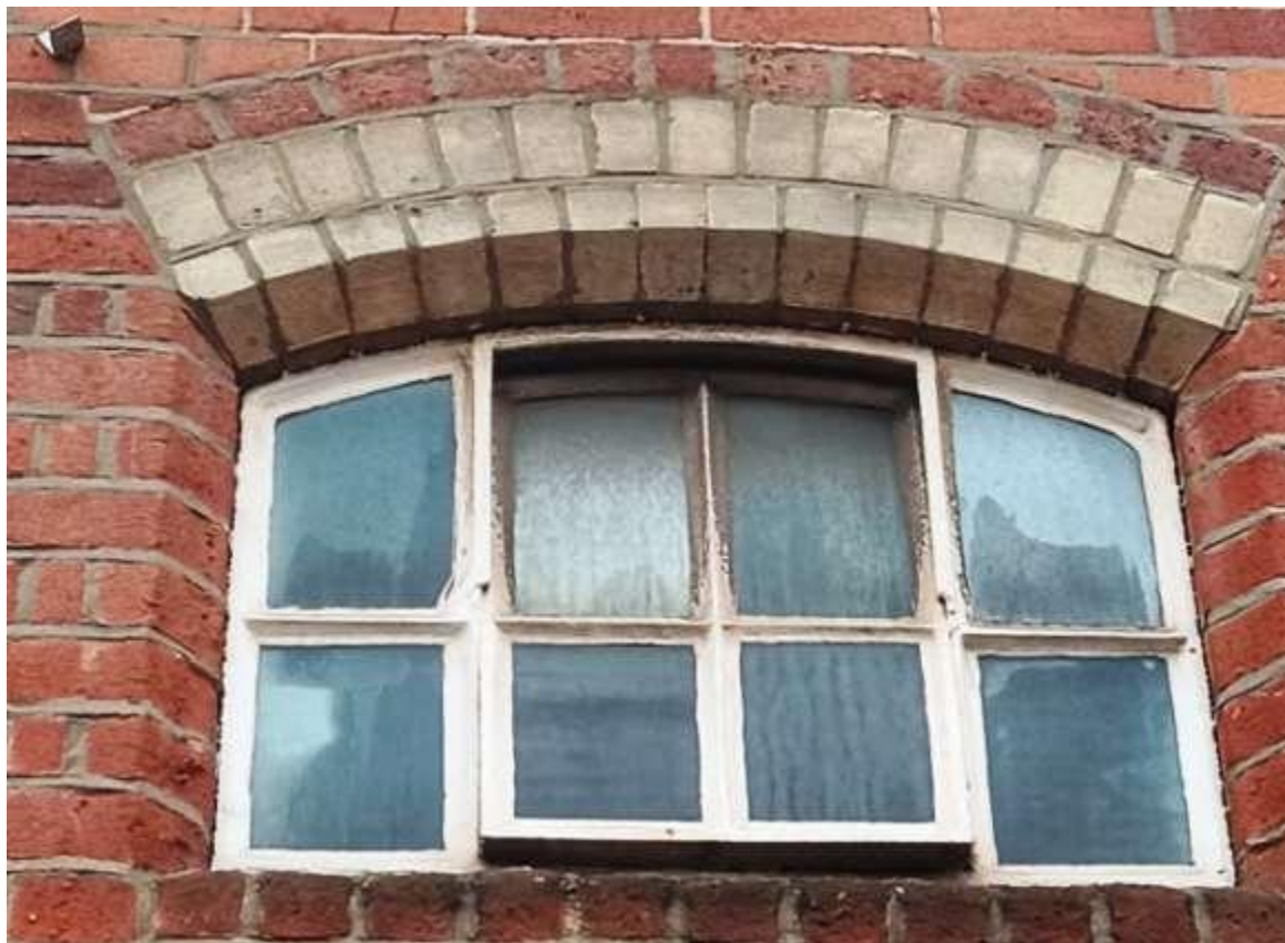
Fig 3.4.2: Cast iron window
