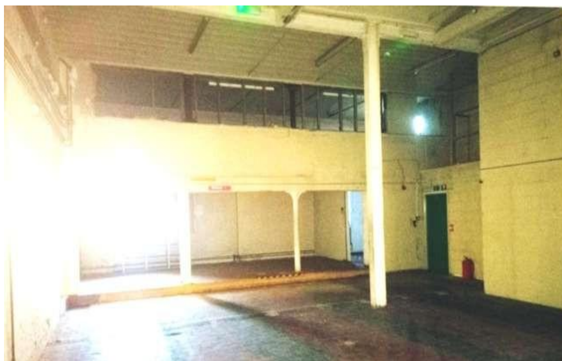
Fig 4.3: South block looking towards first floor offices to front
