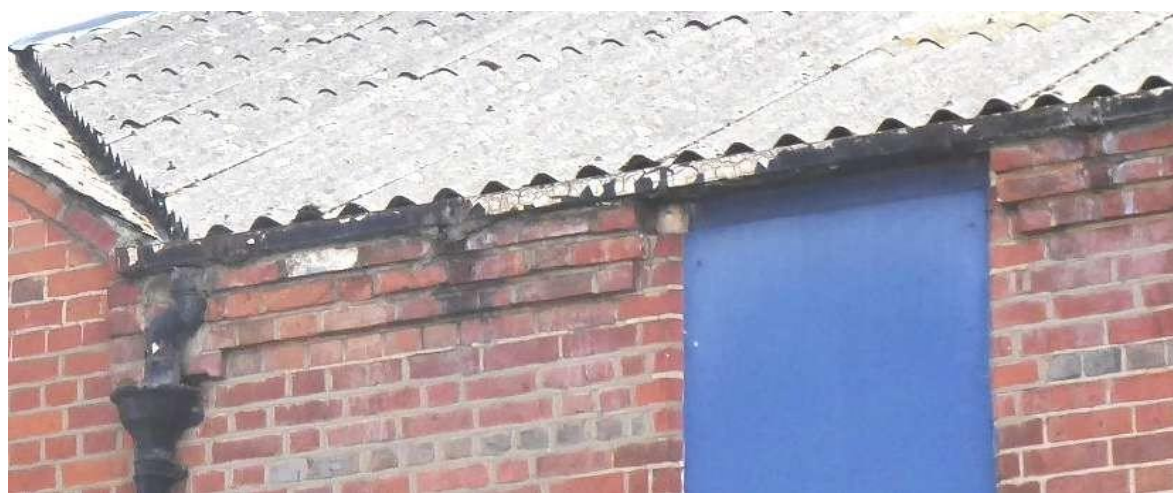
Fig 3.2.6: Eaves to north side of north block (73)
