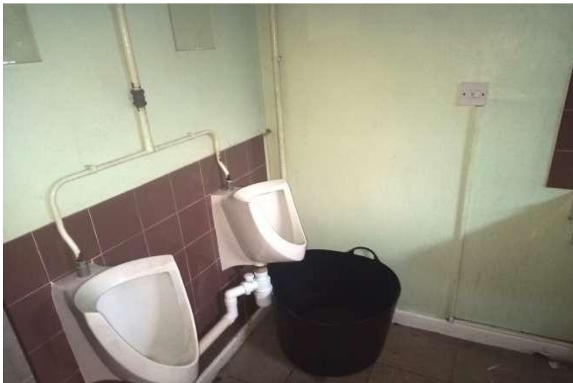
Fig 4.6.4: Toilets to rear section
