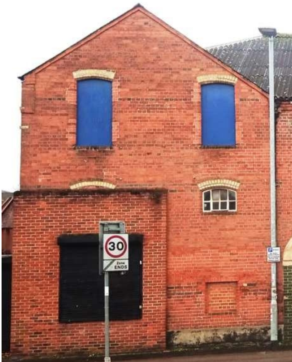
Fig 3.3.5: North gable to end of front cross wing
