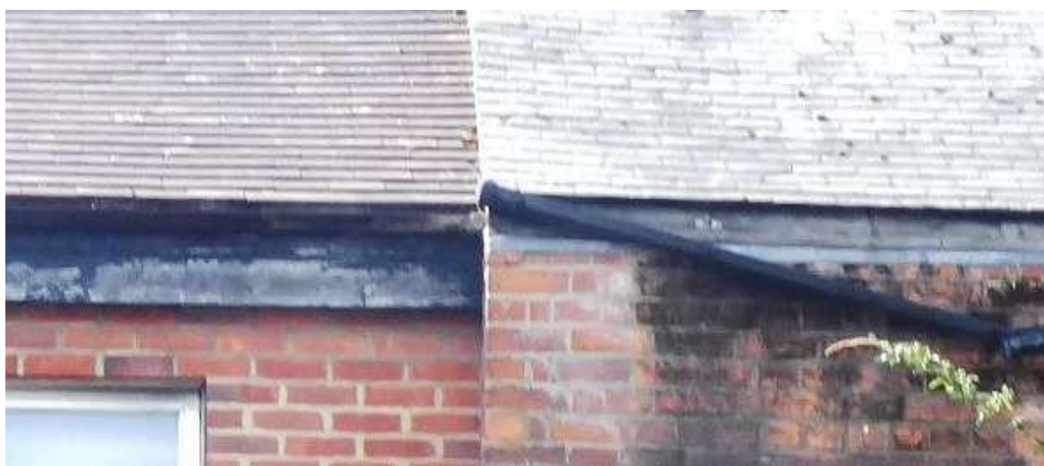
Fig 3.2.4: Eaves to front infill block (left) and main front (right)
