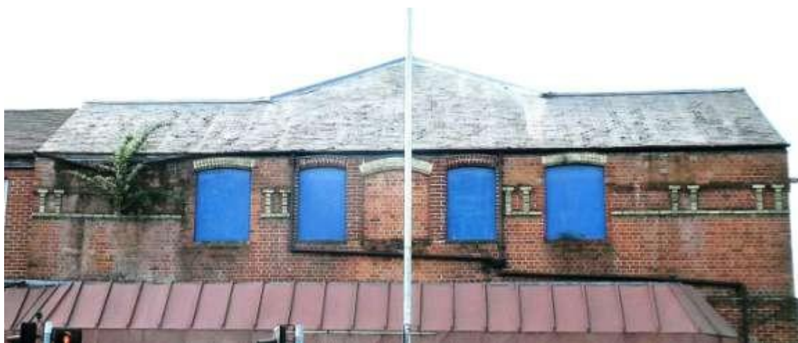
Fig 3.1.2: Front roof of north block (73)
