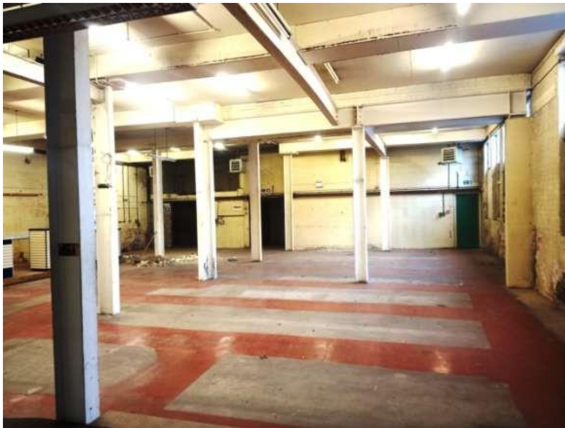
Fig 4.1: North block ground floor looking from front to back
