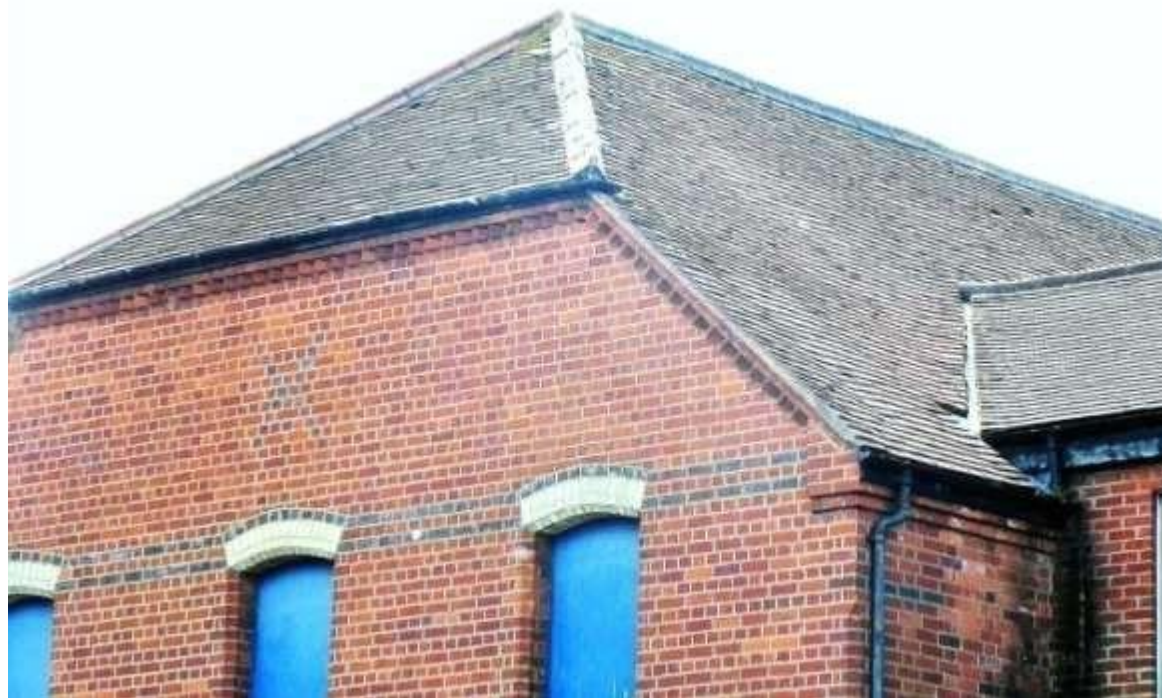
Fig 3.1.6: Front section of south block (71) roof
