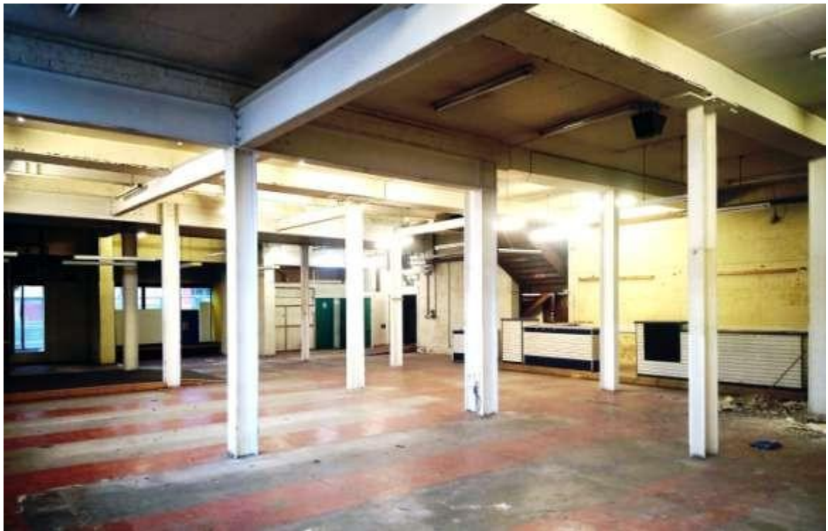
Fig 2.2.12: Ground floor to north block (73) looking to the front
