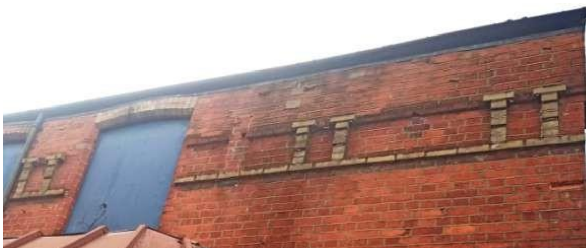
Fig 3.3.13: Decorative brickwork to front of N° 73
