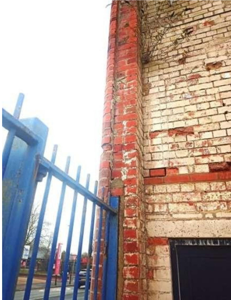
Fig 3.3.25: Link nib on northwest corner to removed building
