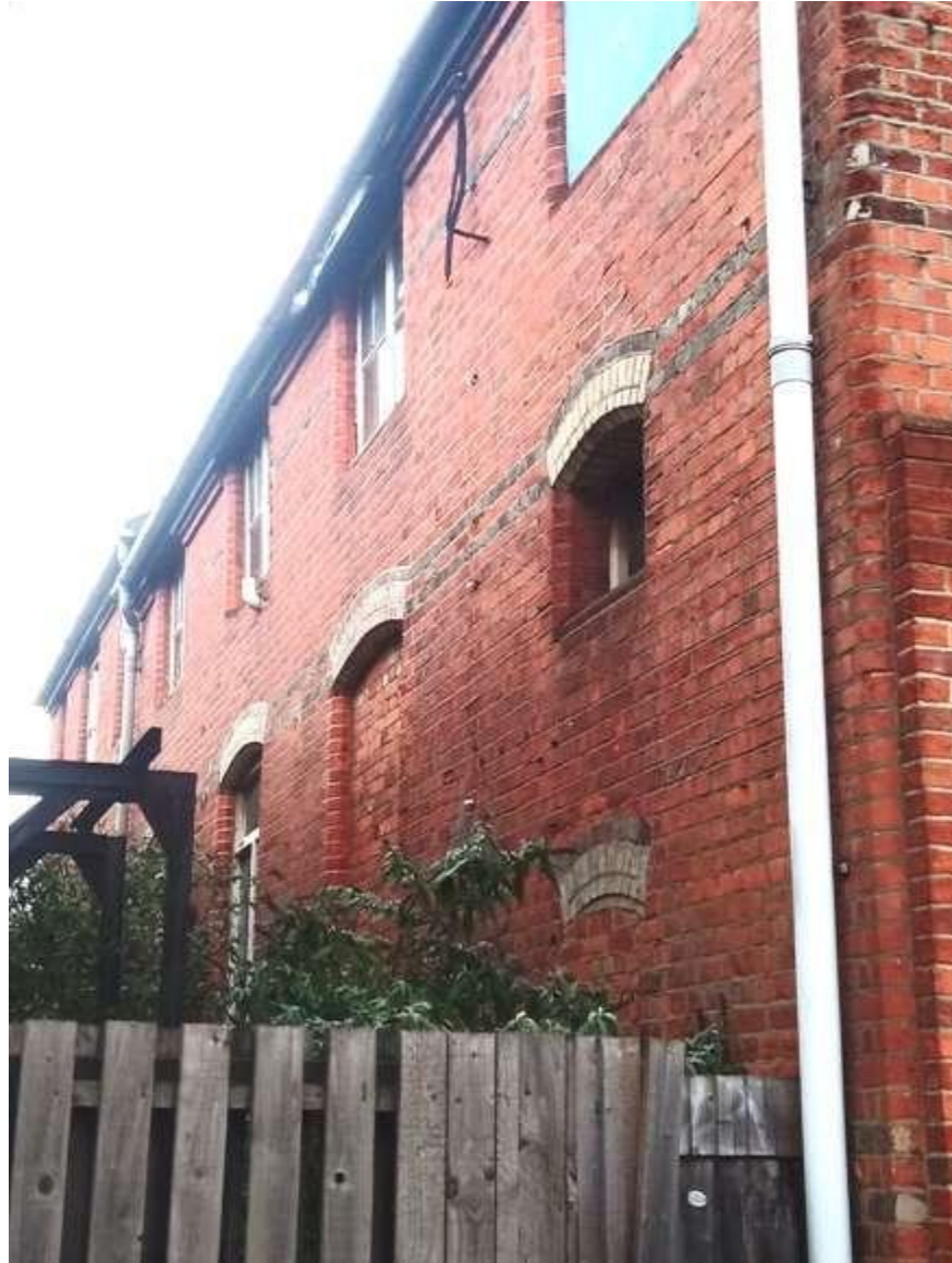
Fig 3.3.17: View of south elevation, showing fenestration pattern
