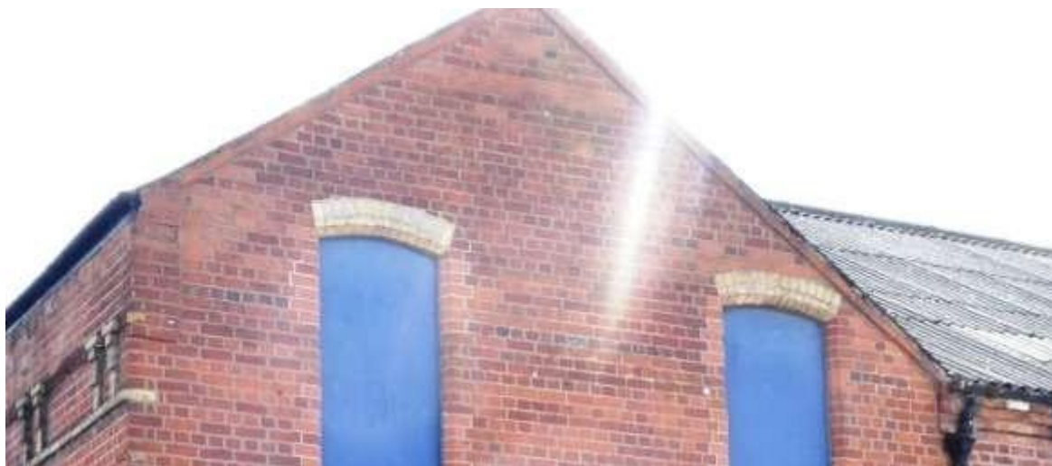
Fig 3.1.3: Eccentric eaves height to the north gable of front wing
