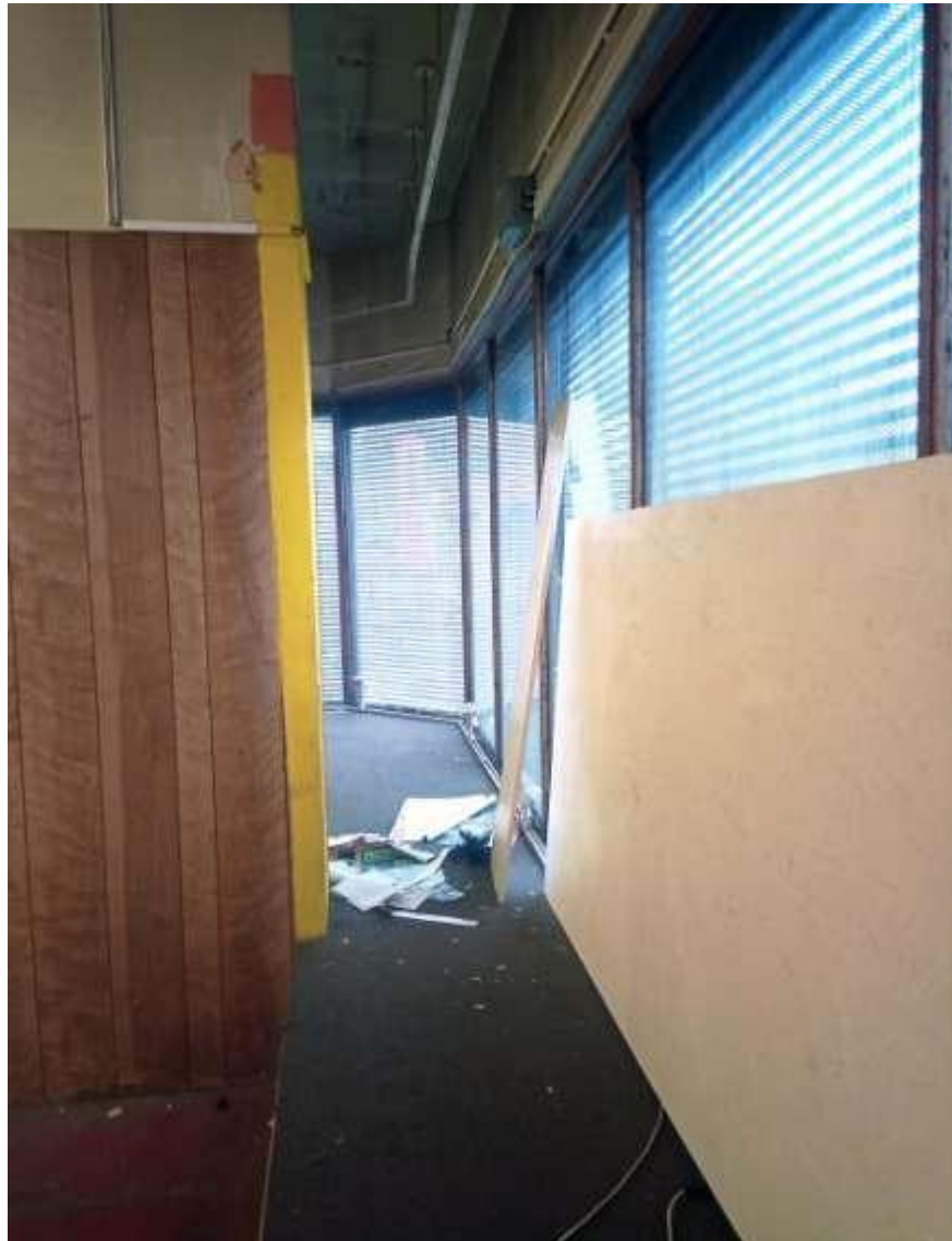
Fig 4.1.8: Interior of frontage retail display area.
