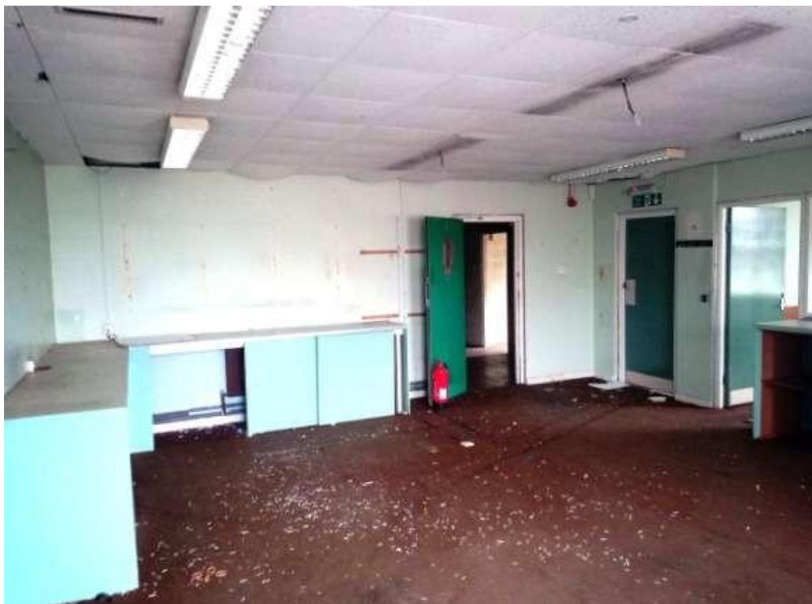
Fig 4.8: South block first floor west end office
