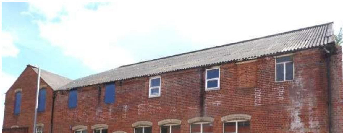
Fig 3.1.1: Roof to north block (73) from west gable
