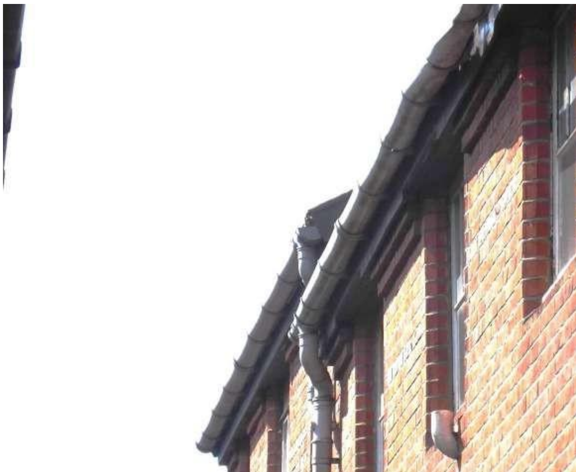
Fig 3.2.2: South wall eaves to south block (71) at east and west part junction
