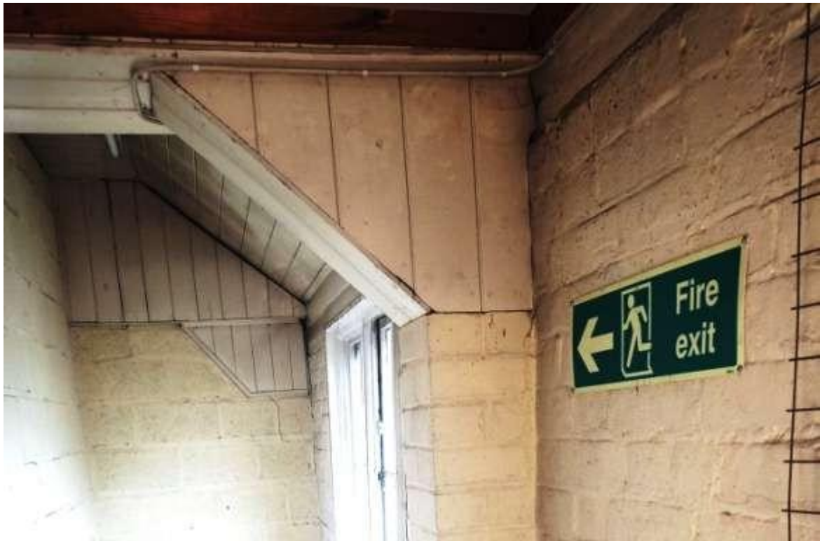
Fig 4.7.3: Boxed truss end on brick nib
