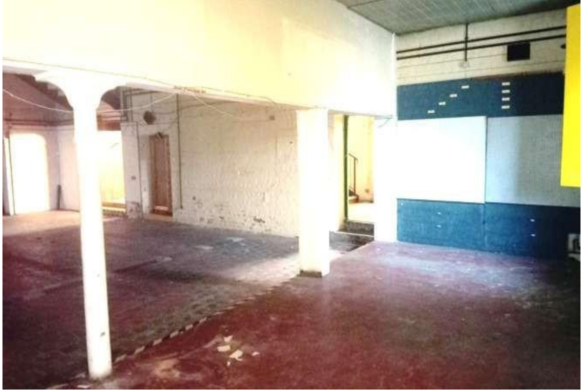
Fig 4.3.1: Front of south block, under office section
