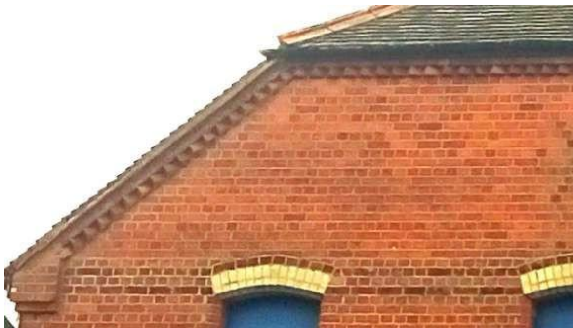
Fig 3.2.1: South block east gable
