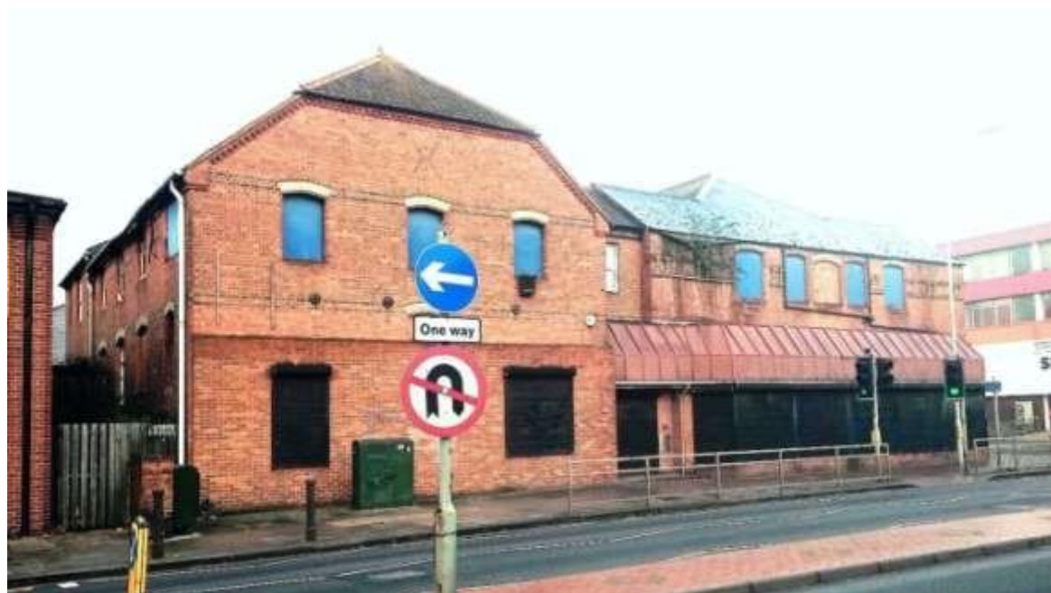
Fig 2.1.2: 71 - 73 Caversham Road from the southeast (71 left)
