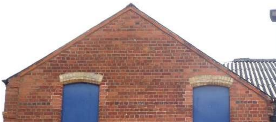
Fig 3.2.5: North gable to front cross roof to N° 73
