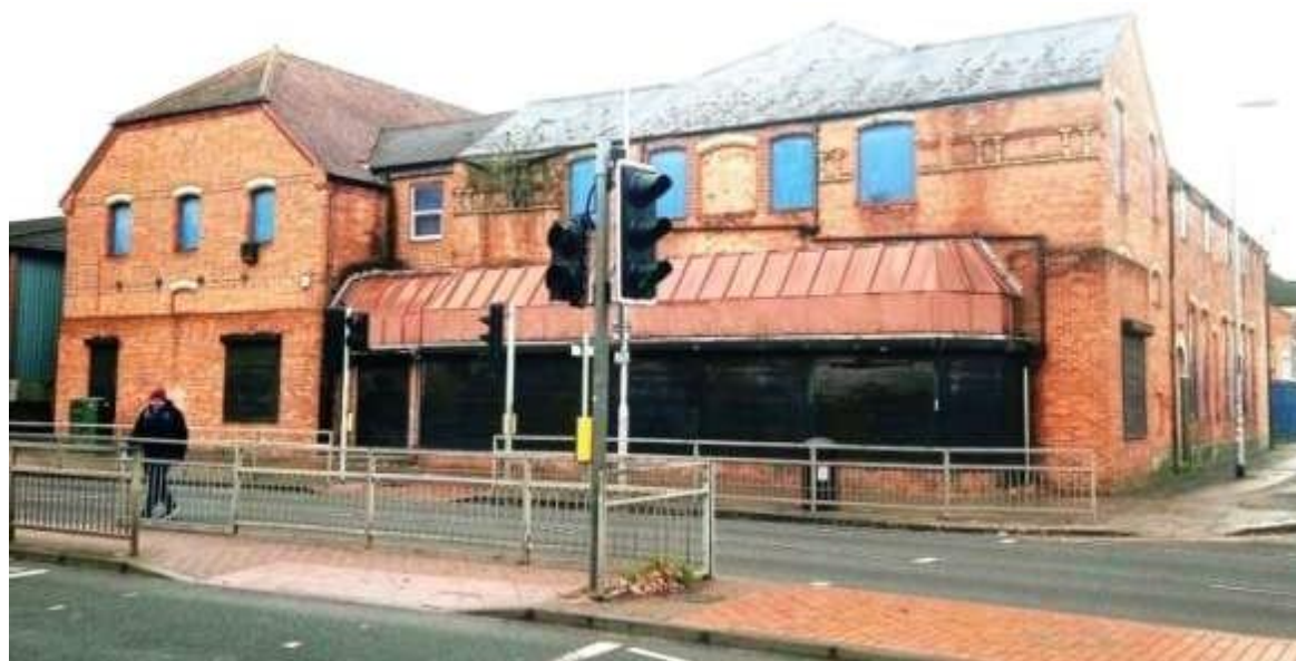
Fig 2.1.2: 71 - 73 Caversham Road from the northeast (71 left)
