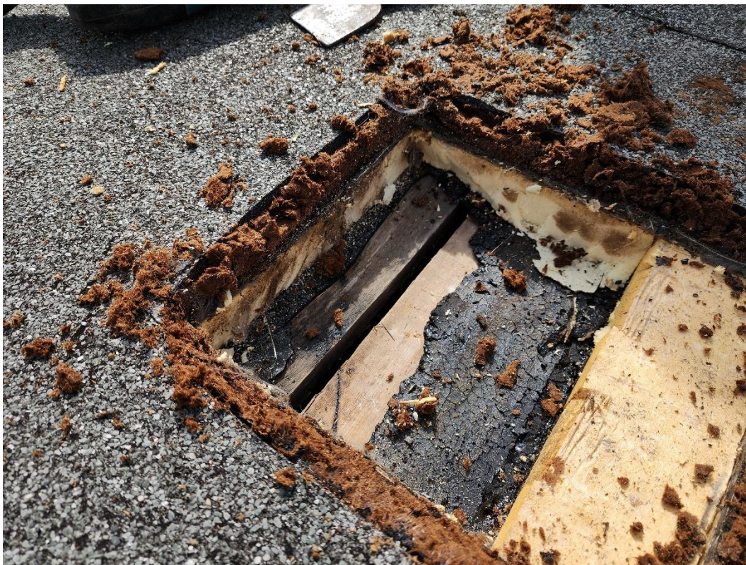
Photo 7 - Core 4 - Note insulation and softwood boards with ventilation gaps.
