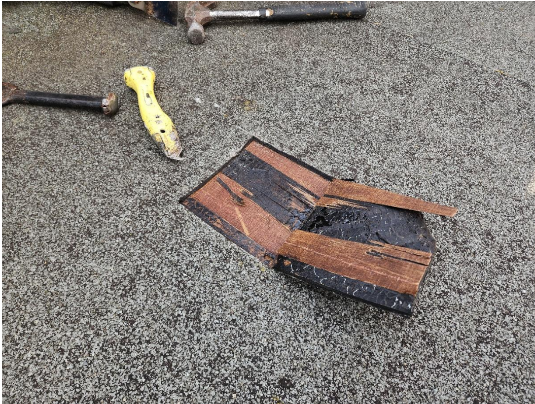
Photo 16 - Core sample 6 – (Lower section of roof area 4)
