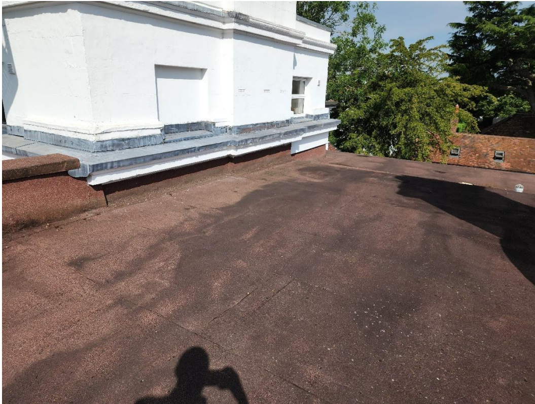
Photo 3 - General view of Roof 1
