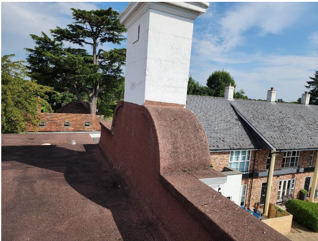
Photo 4 - Chimney to Roof 1
