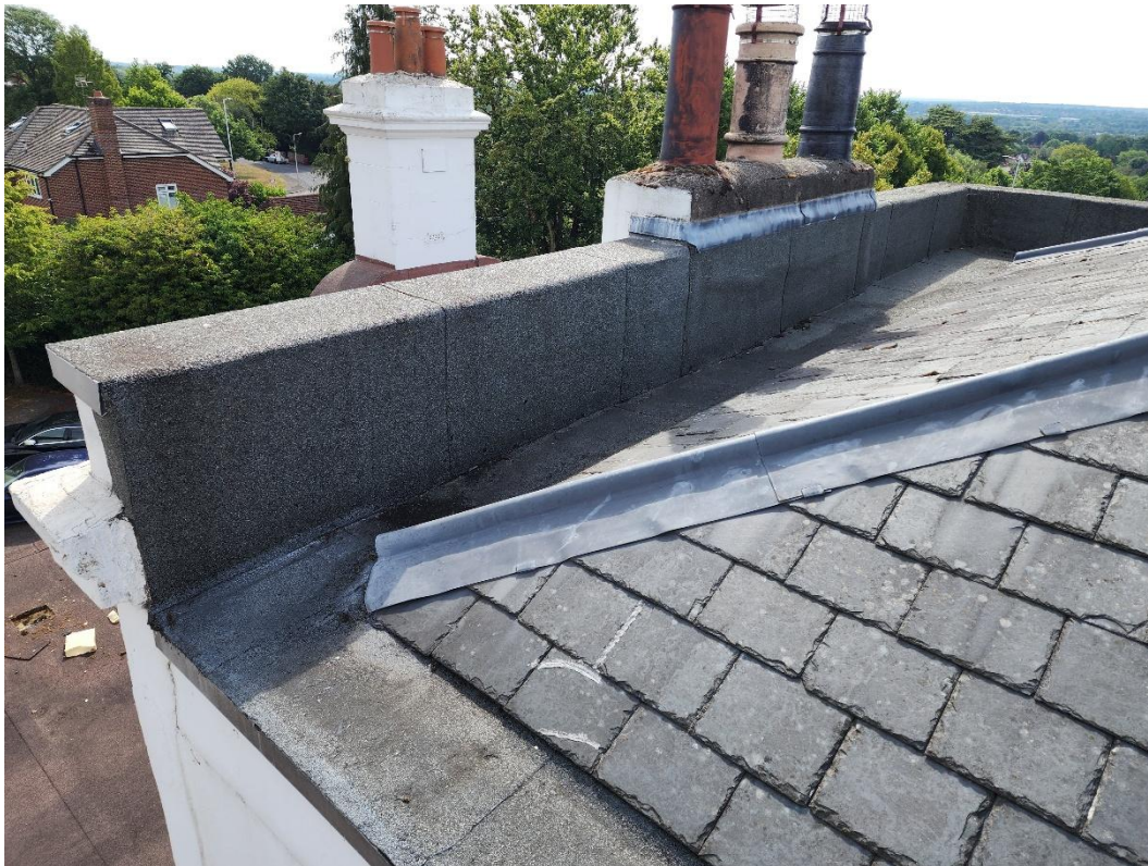
Photo 9 - Perimeter detail to Roof 3
