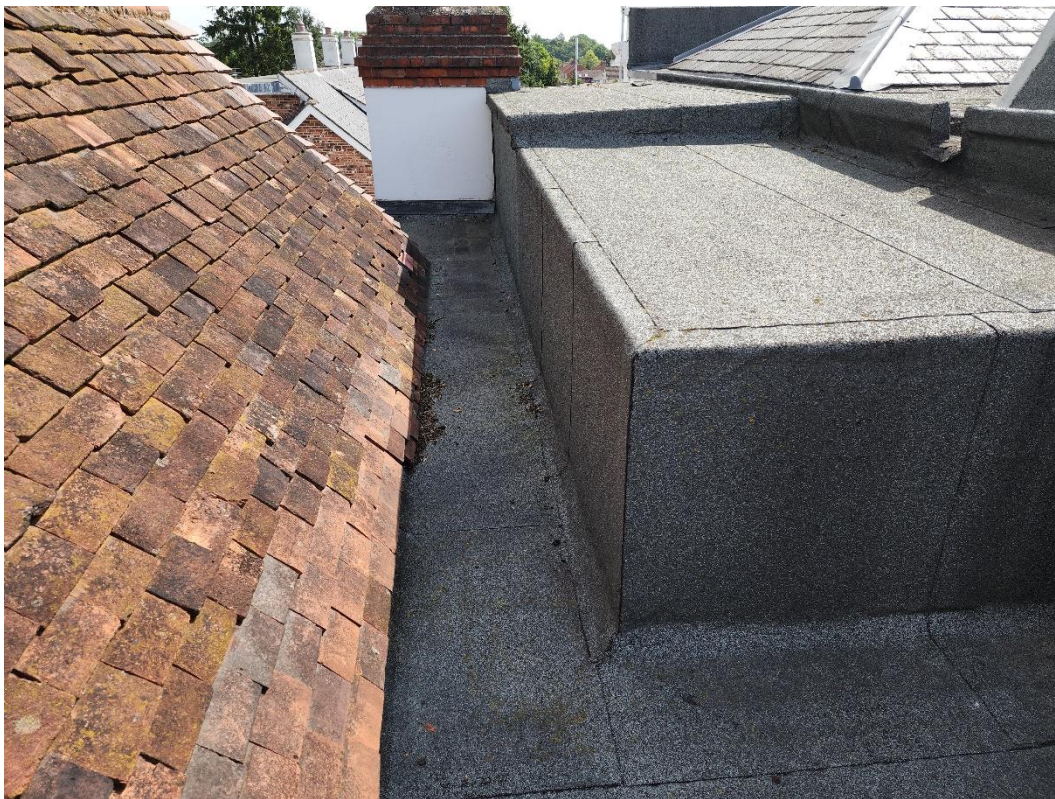
Photo 17 - View looking towards upper section of roof area 4.
