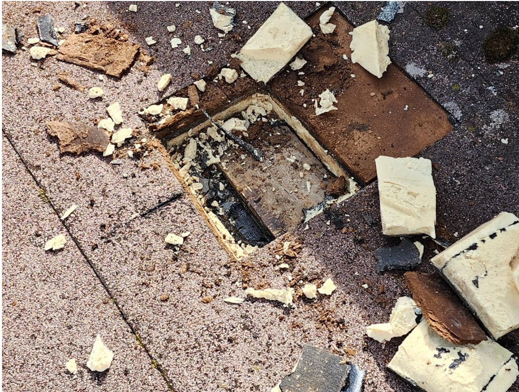
Photo 1 - Core 1 – Note plywood to perimeter.
