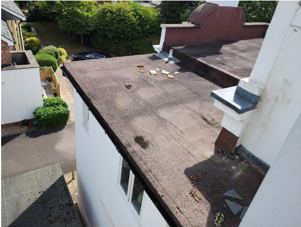
Photo 5 - General view of roof 2 from above
