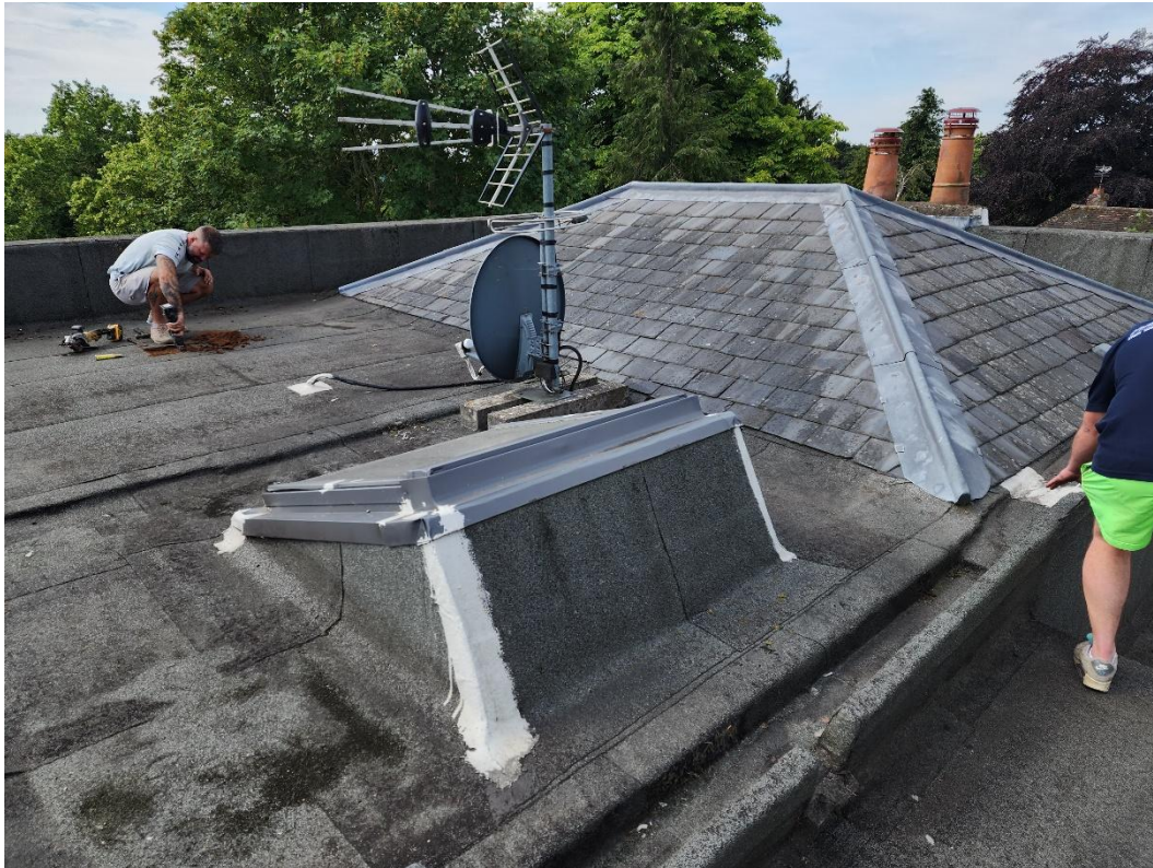
Photo 12 – Roof 3 – Note liquid applied coating to rooflight.
