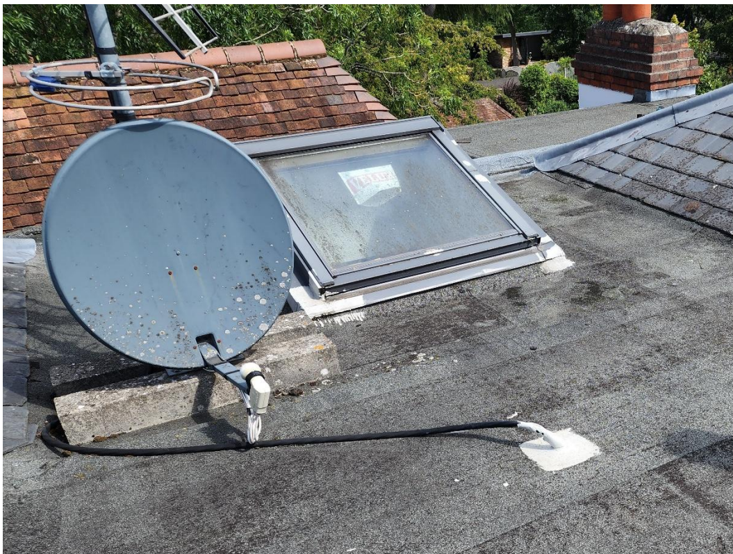
Photo 13 - Roof 3 - Liquid applied coating to cable outlet
