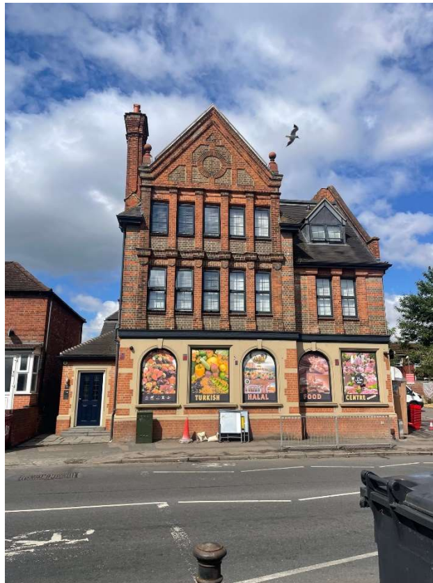
Existing façade of the BTM facing Whitley Street
