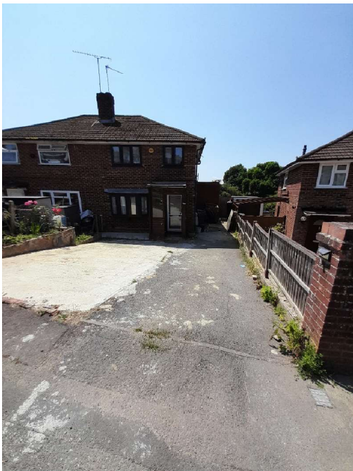
Looking towards front elevation.
