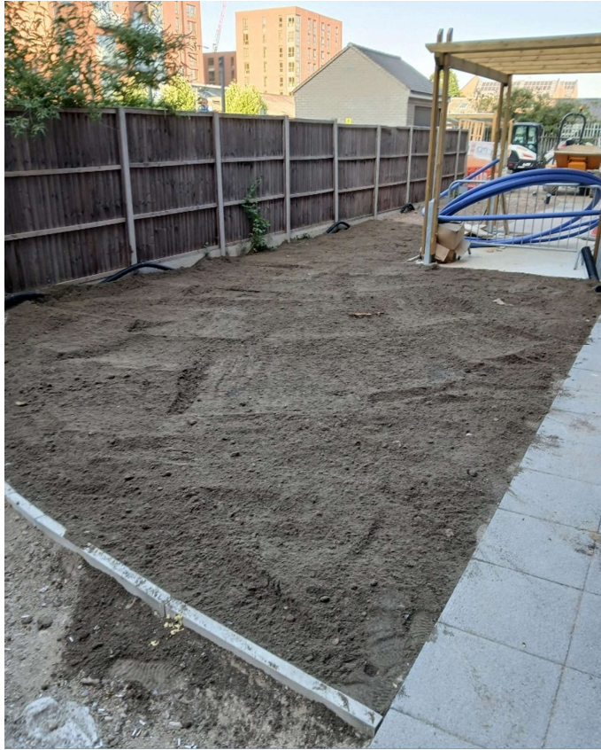
Figure 17: Photos received from the client on 16/06/25, showing final levels of topsoil.
