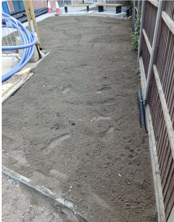
Figure 15: Photos received from the client on 16/06/25, showing final levels of topsoil.
