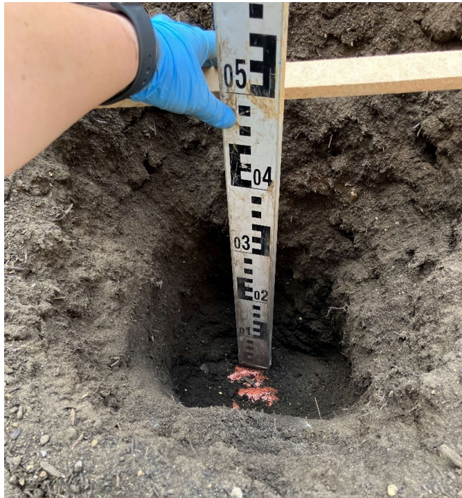
Figure 9: HP4 noted with 480mm of soil. Final soil levels will be topped up to 500mm to finished curb level. Orange marker membrane noted at base.
