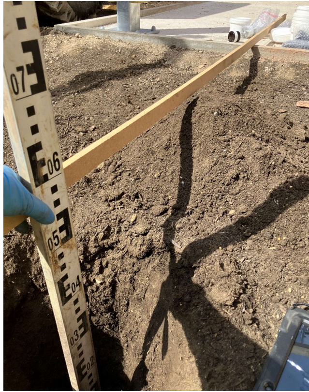
Figure 5: HP2 levels noted to be approximately 580mm once topsoil has been placed to final finishing level.
