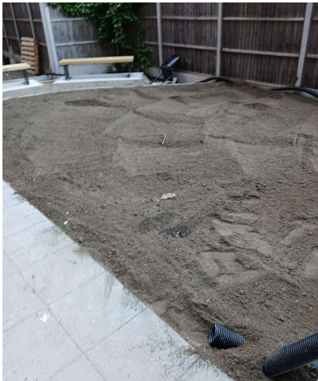
Figure 16: Photos received from the client on 16/06/25, showing final levels of topsoil.
