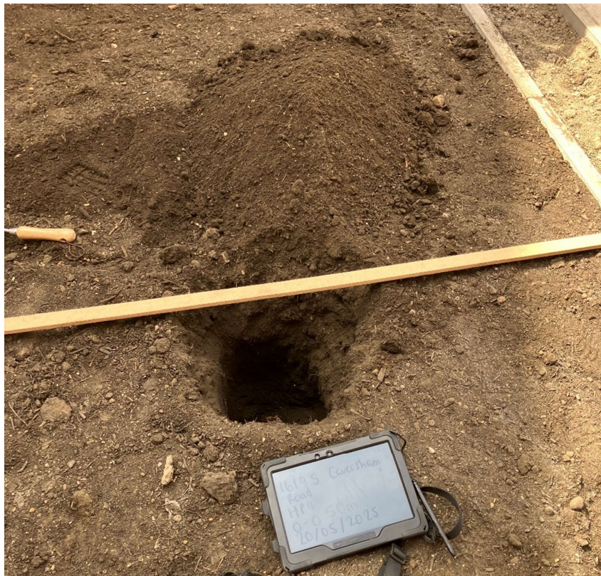
Figure 10: HP4 topsoil arisings and levelled with finished curb level.
