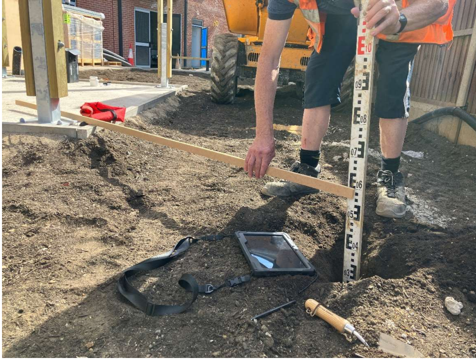
Figure 1: Hand Pit 1 (HP1) dug with 400mm thickness of soil noted. Final soil level once topped up to finished levels will be approximately 580mm.
