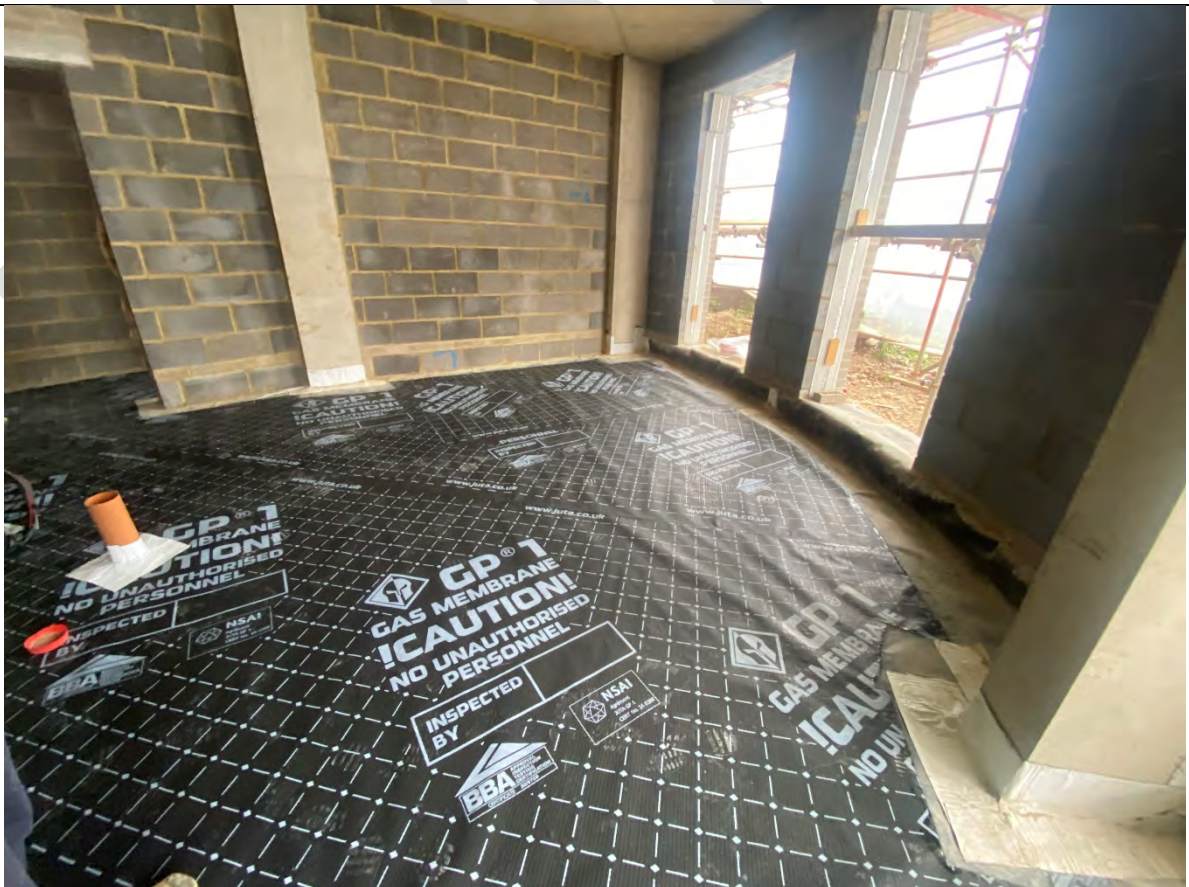
Photograph 2: General condition of membrane.
