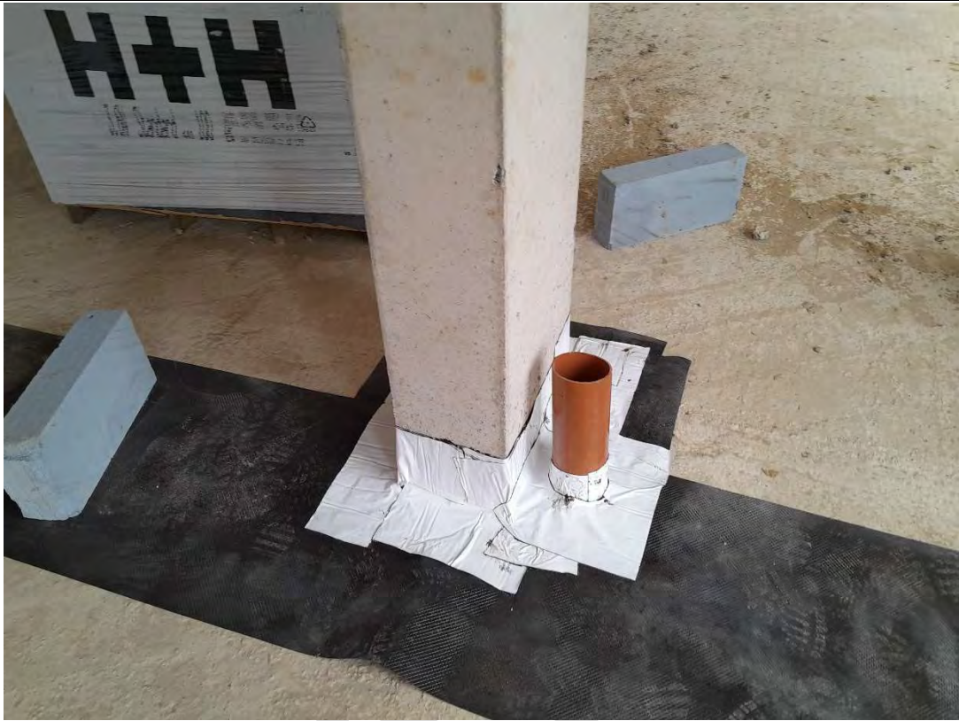
Photograph 7: Non-proprietary top hat service detailing
