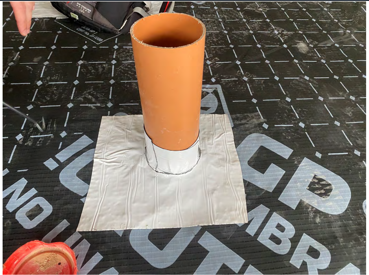
Photograph 5: Non-proprietary top hat service detailing.
