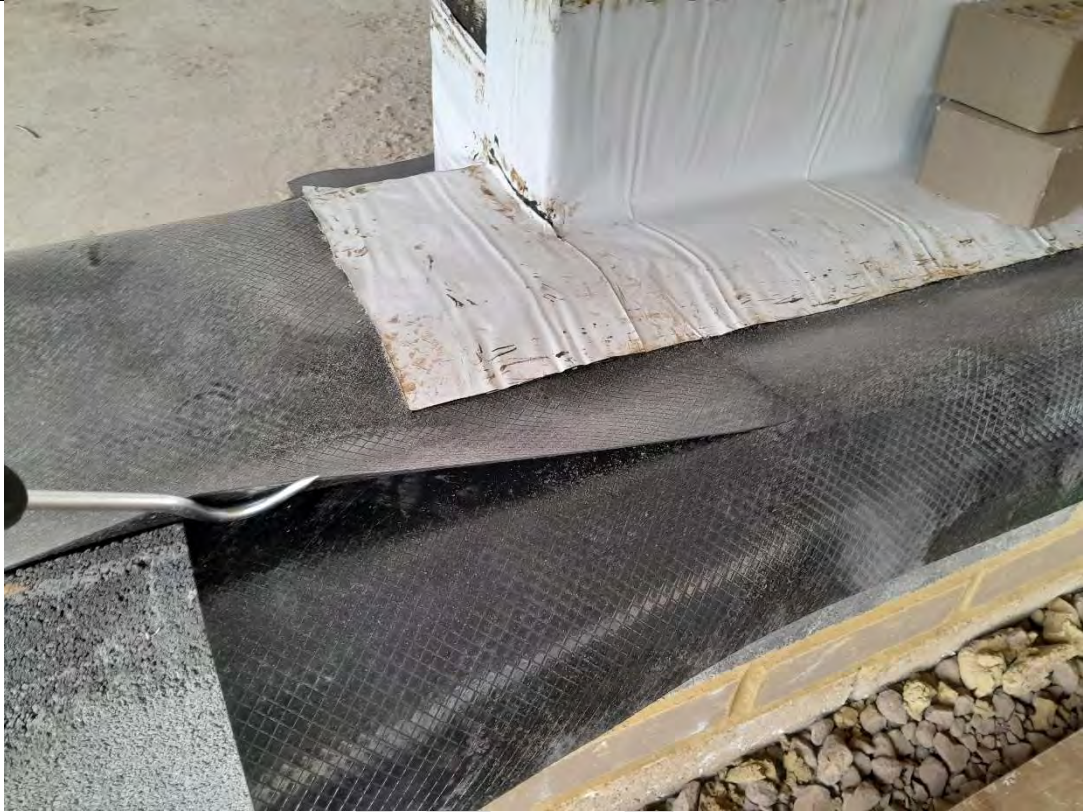
Photograph 5: sufficient overlap
