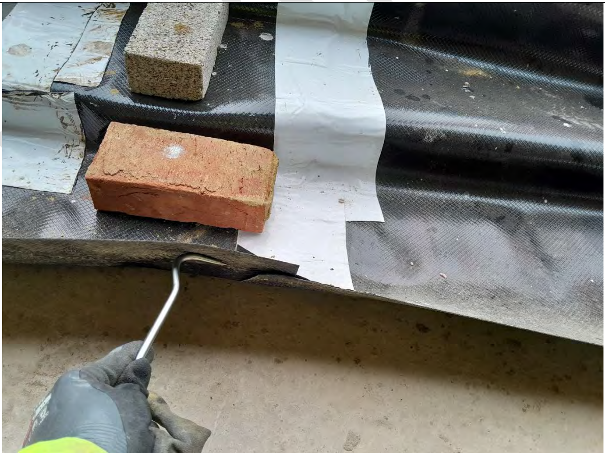
Photograph 6: Overlap <150mm with additional tape
