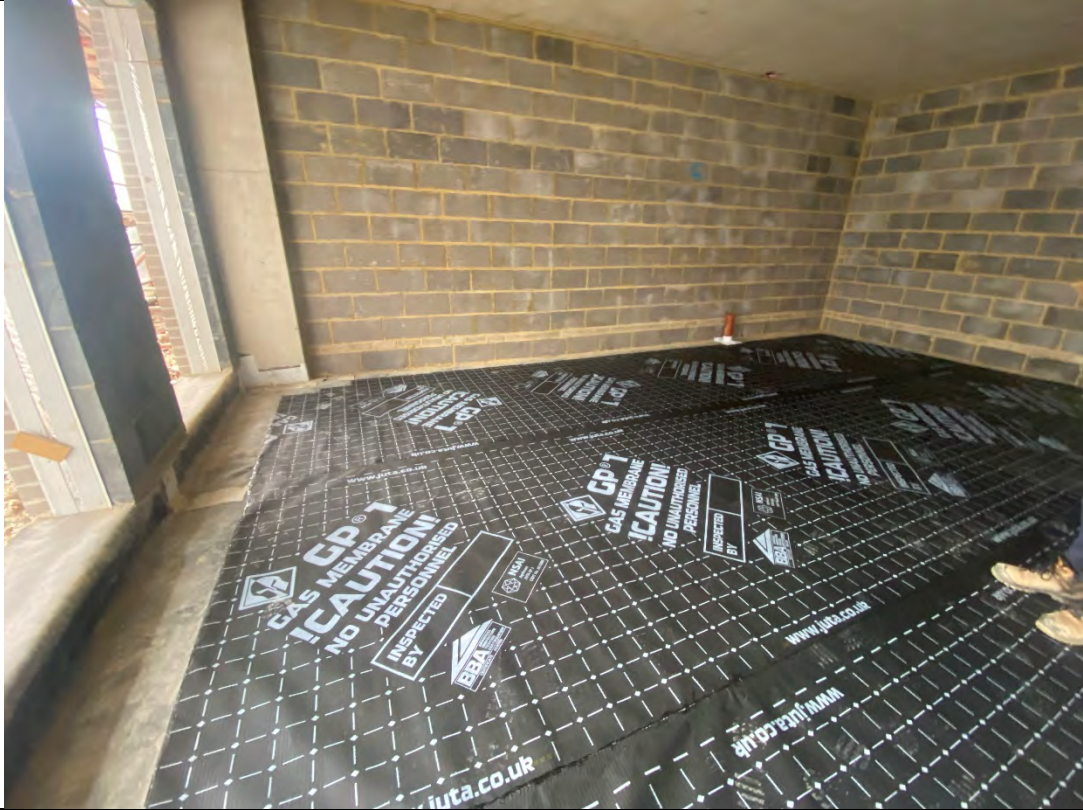
Photograph 1: General condition of membrane.
