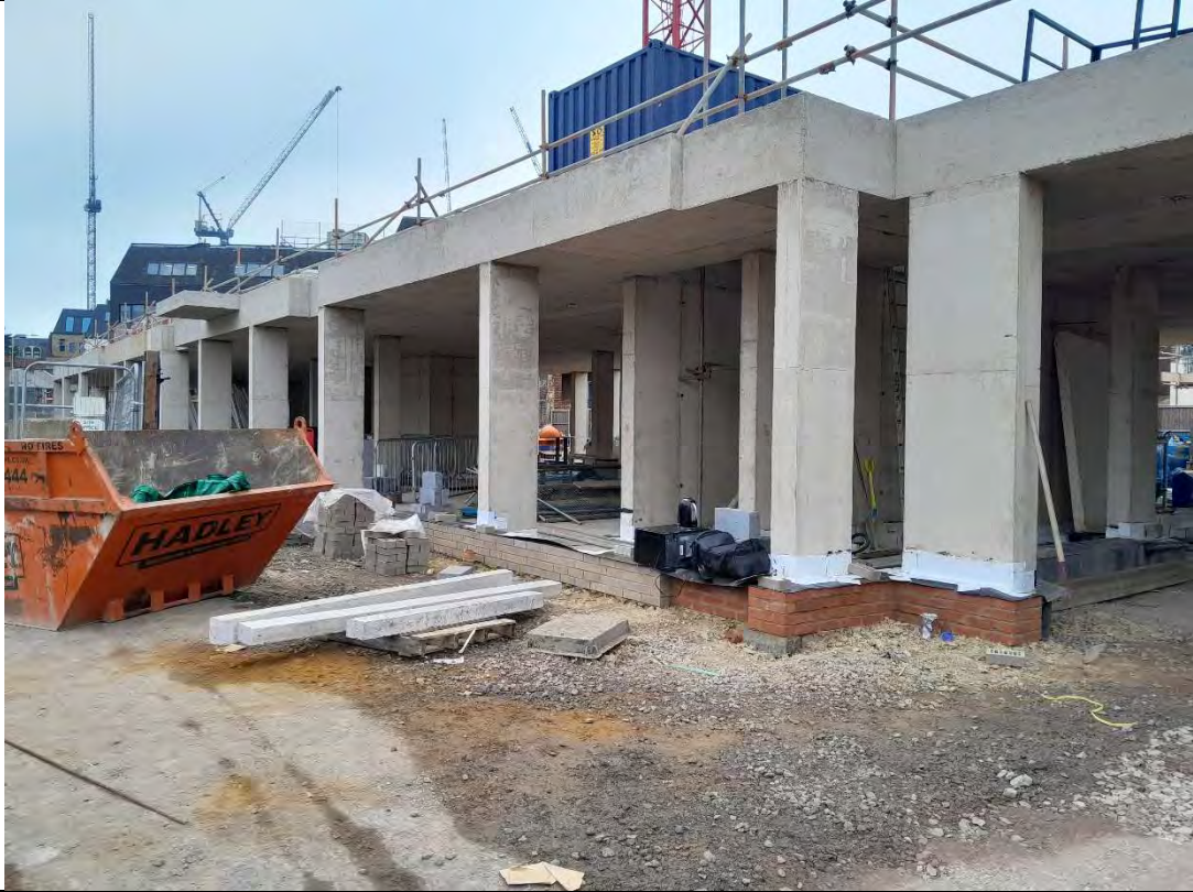
Photograph 1: General site condition
