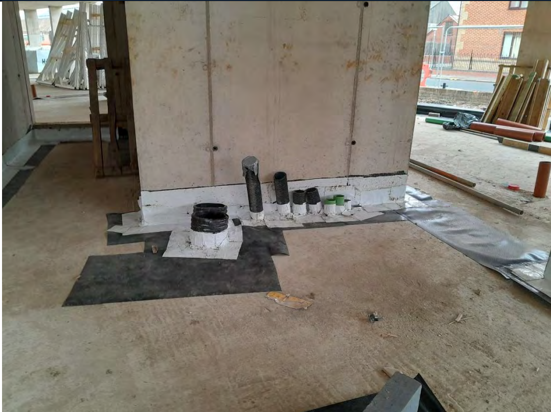
Photograph 3: DPC and detailing around internal walls and nearby services
