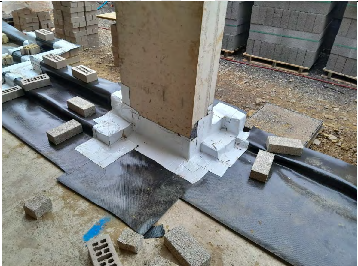
Photograph 2: DPC and detailing around external walls
