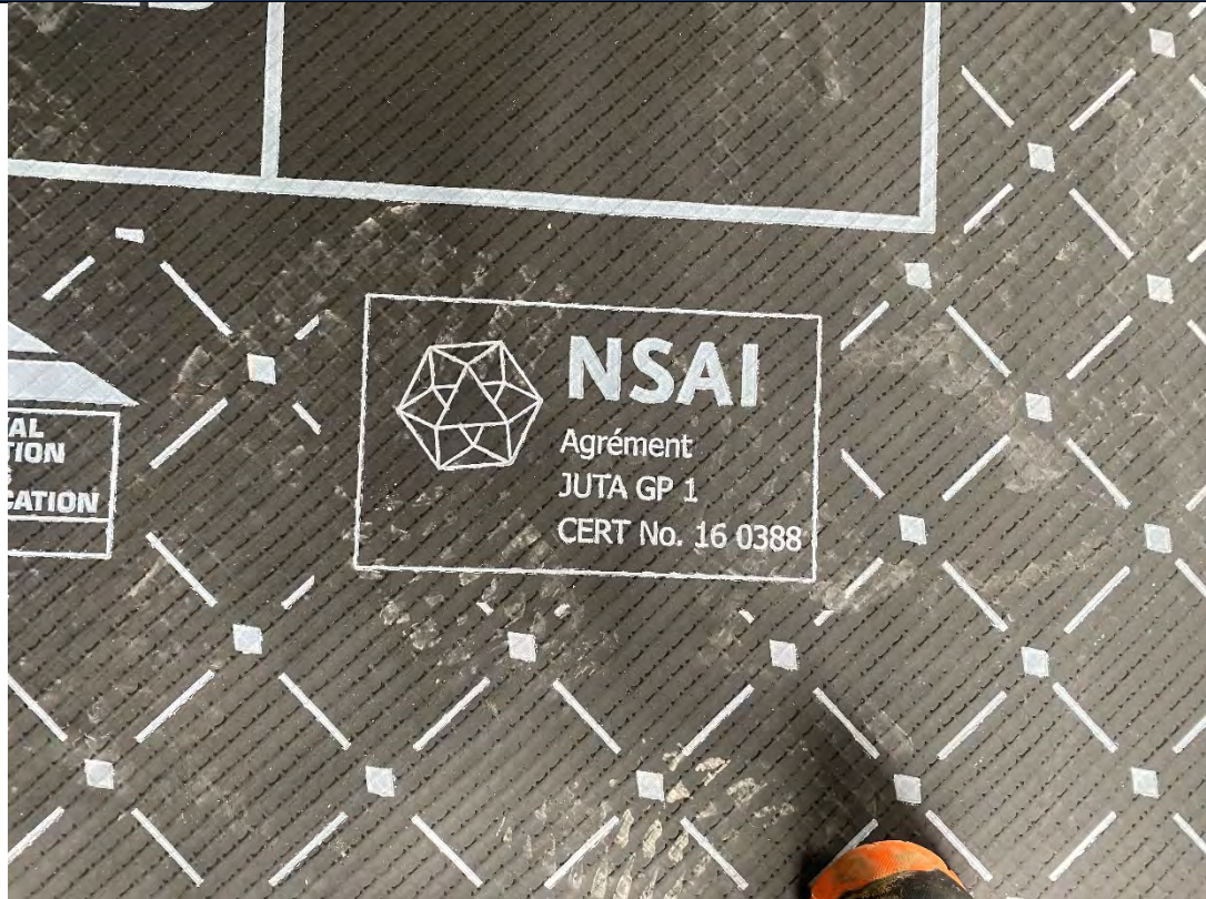
Photograph 3: Type of membrane used shown.
