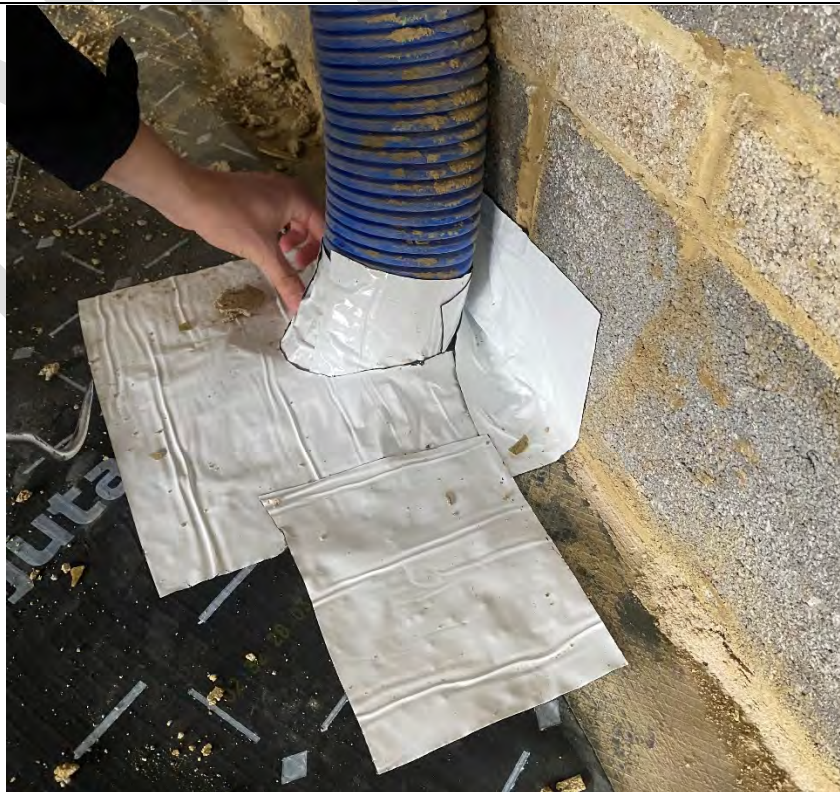
Photograph 6: Non-proprietary top hat service detailing.
