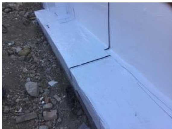
The SAGM has been adhered to the previously installed membrane.
