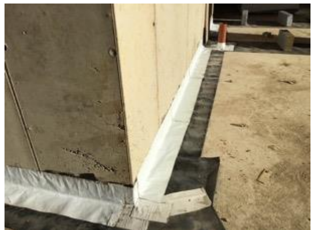
Retro fit detail using SAGM.
