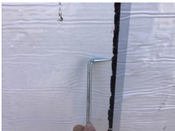
Pick testing all SAGM detailing.
