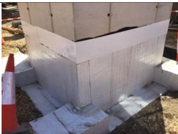
Overview of wrapped SAGM to lift pit 2.
