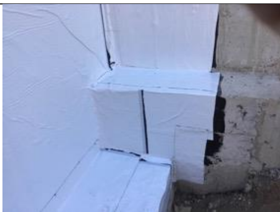
Corner seal using SAGM.
