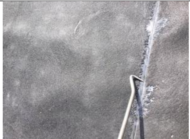
Pick testing to the welded lap joint.
