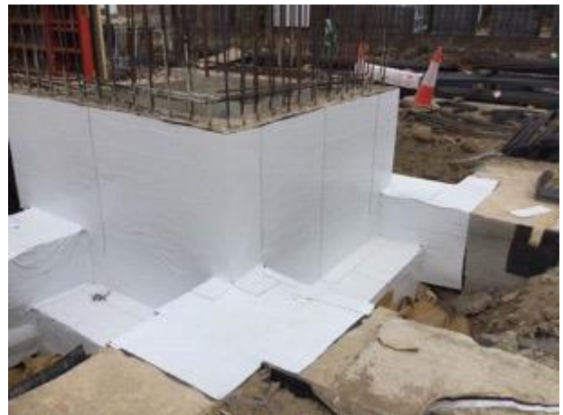
SAGM tanking applied to the lift pit wrap.
