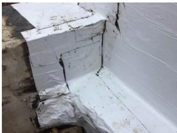
Corner seal using SAGM.
