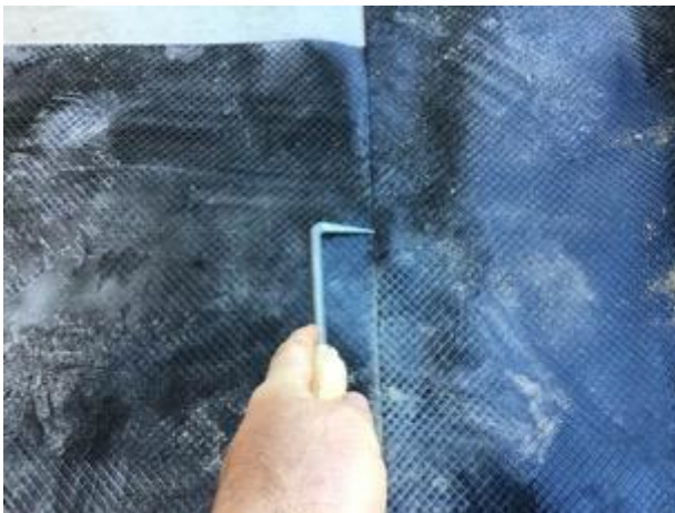
Pick testing all welded membrane laps.
