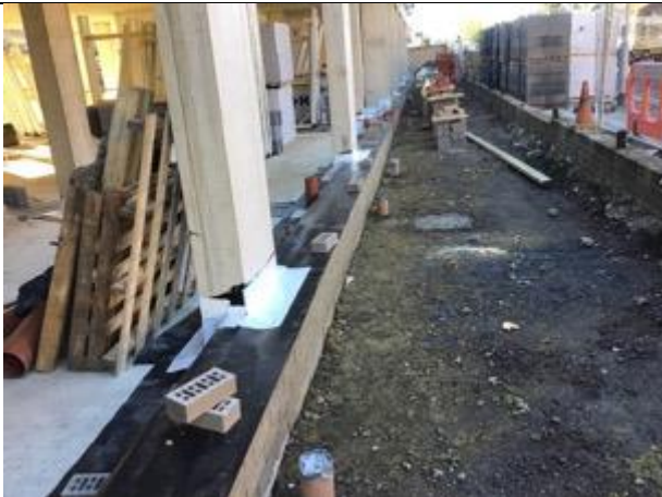
Overview of installed Juta GR DPC to the perimeter of Apartment Block A.
