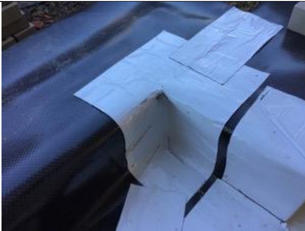
Typical corner seal using SAGM.
