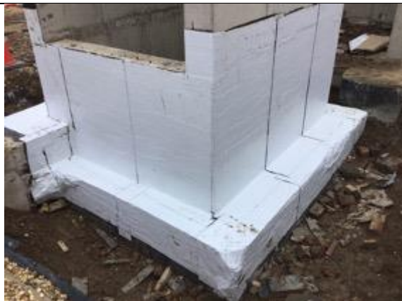
Overview of installed SAGM as a wrap to lift pit 3.
