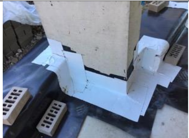
Sealed concrete column using SAGM.
