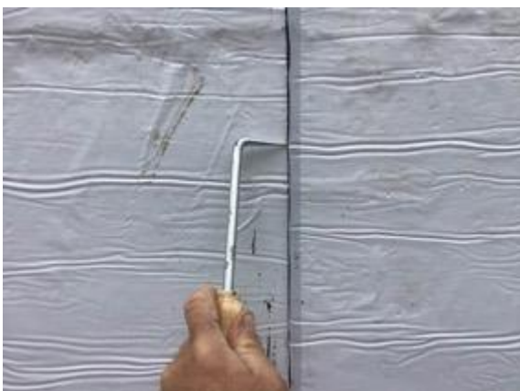
Pick testing all SAGM detailing.
