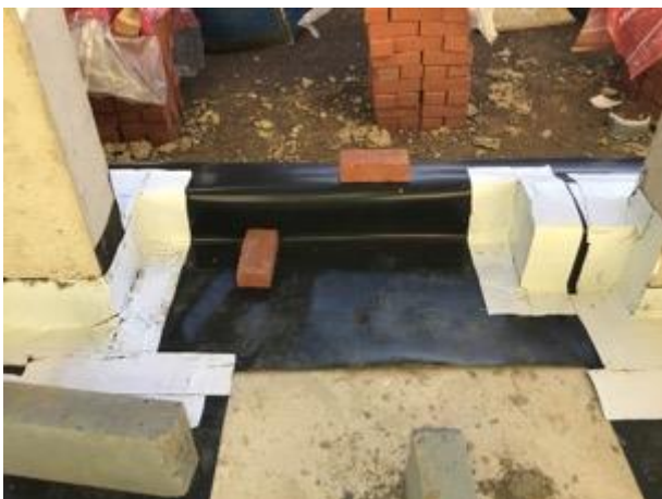
Typical door threshold seal using SAGM.
