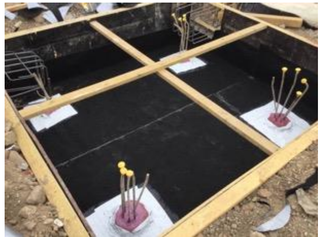
Overview to the completed lift pit base.
