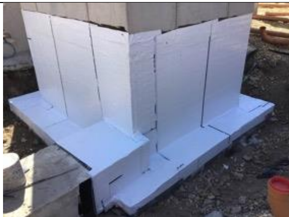
Overview of wrapped SAGM to lift pit 1.
