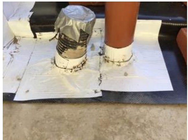
Typical pipe penetration seals using SAGM.
