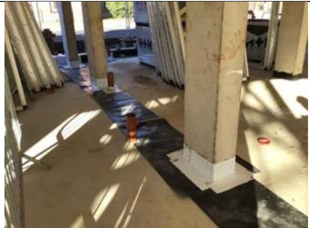
Overview of installed Juta GR DPC to the internal wall.
