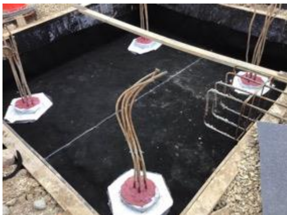
Overview of installed Juta GP Titanbond gas barrier to lift pit 1.
