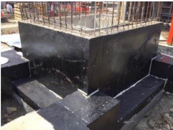
Lift pit has been coated in JUTA Bitumen Primer.
