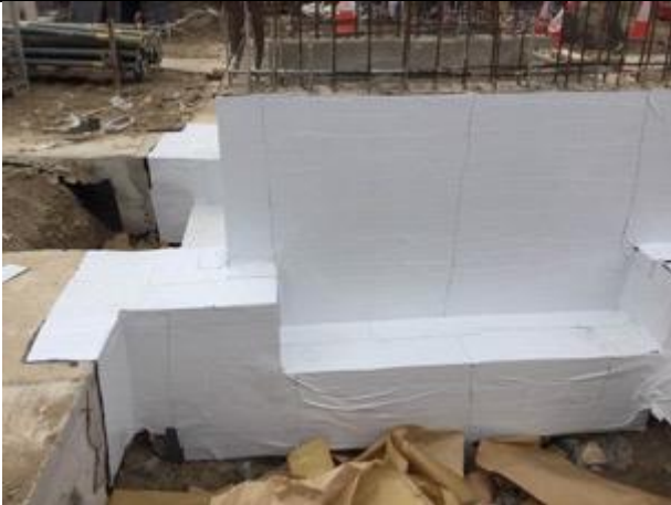
Overview showing the lit pit wrap.
