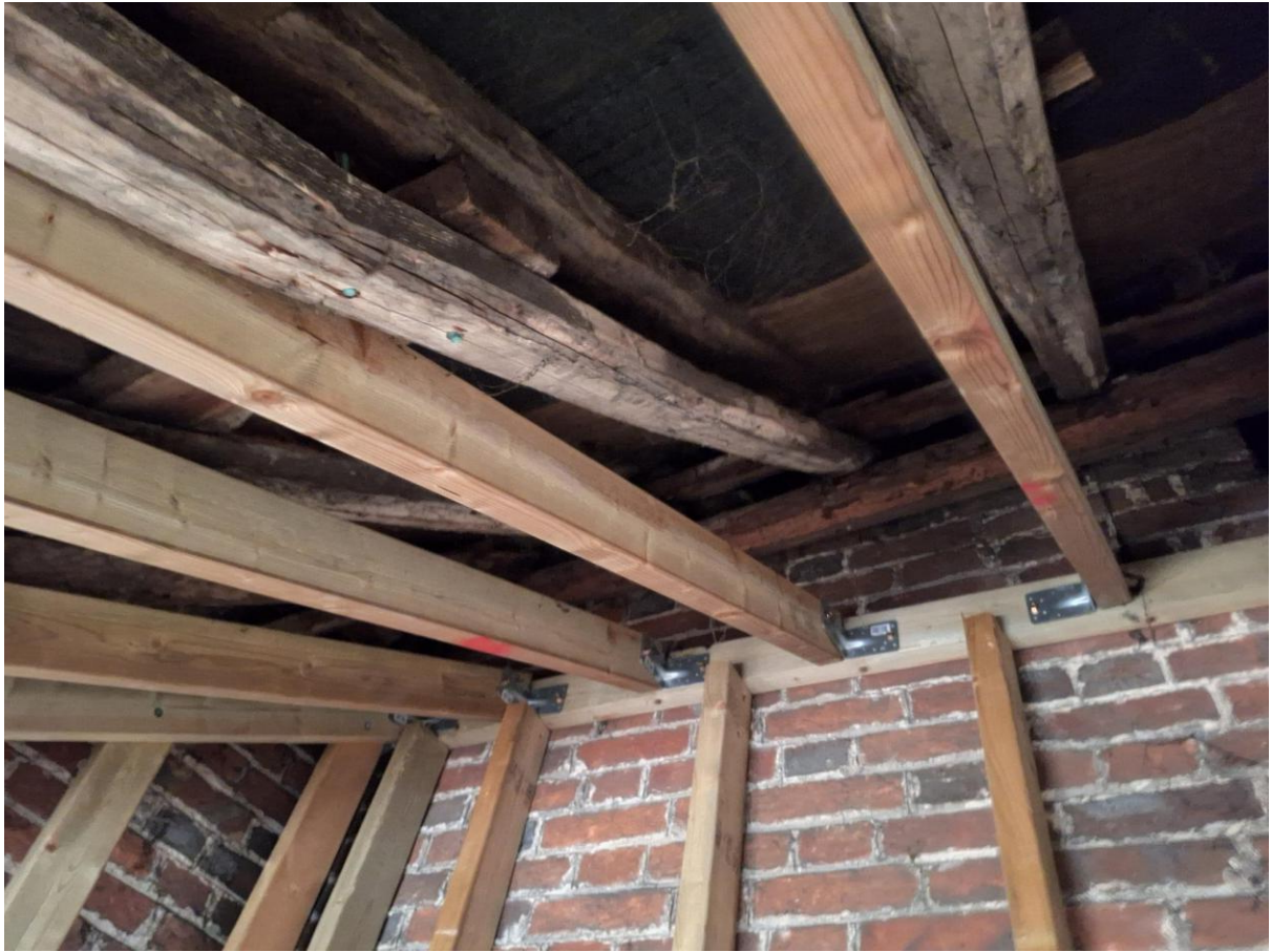
Figure 3. Image showing the existing C20 plasterboard ceiling & wall finish removed exposing the existing walls and roof rafters. The existing rafters have been inspected and are in good condition, no replacements or repairs are required.
