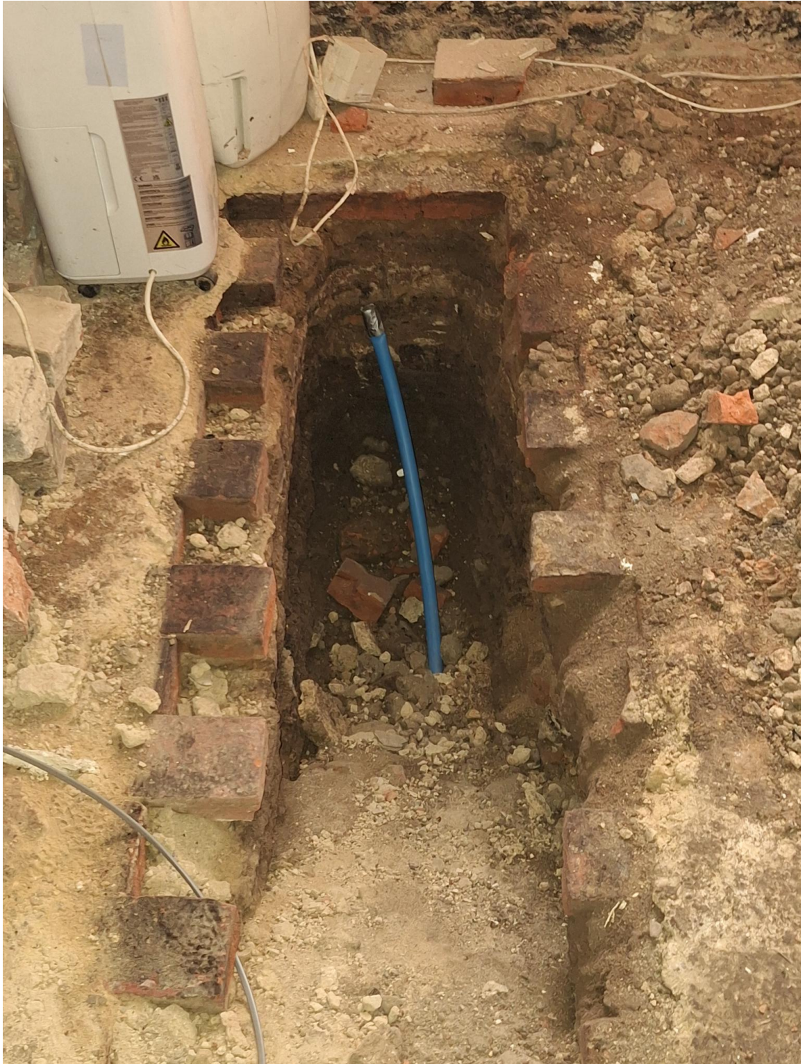
Figure 1. Image showing the installation of the 25mm diameter MDPE water supply pipe in a 457mm wide trench through the existing Dining Room floor refer to Construction Detail A.
