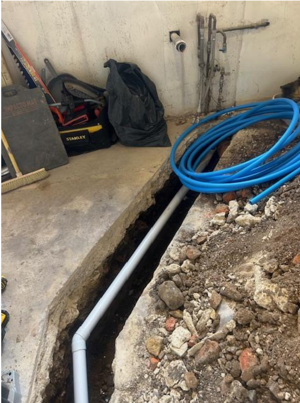
Figure 2. Image showing the installation of the 25mm diameter MDPE water supply pipe in a 225mm wide trench through the existing Kitchen floor to be connected to the existing stop cock refer to construction Detail B.
