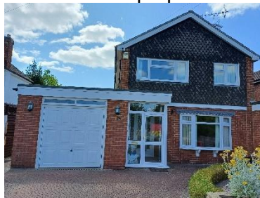
Fig 1: View from the front of the property (08/07/25)
