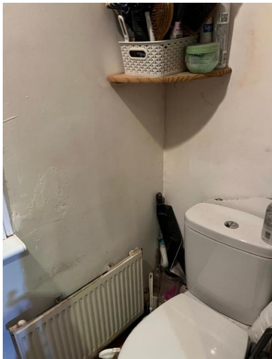
Current condition of Flat B (First Floor)
