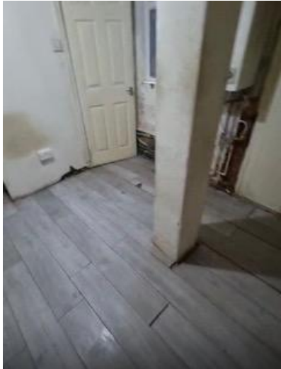
Current condition of Flat A (Basement)
