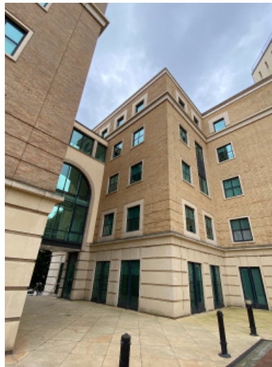
4 - South Elevation (Courtyard Side)
