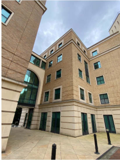
East Elevation, southern wing
