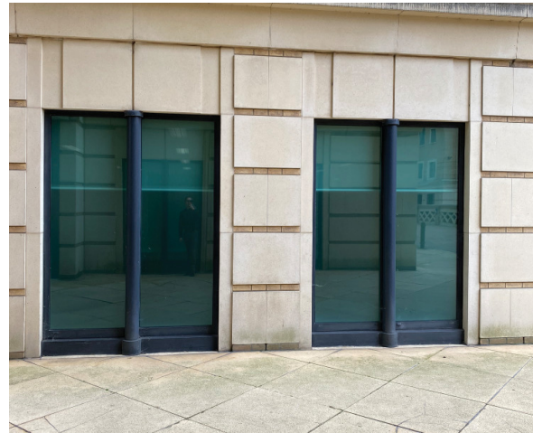
Example 1 - Typical existing ground floor fixed windows
