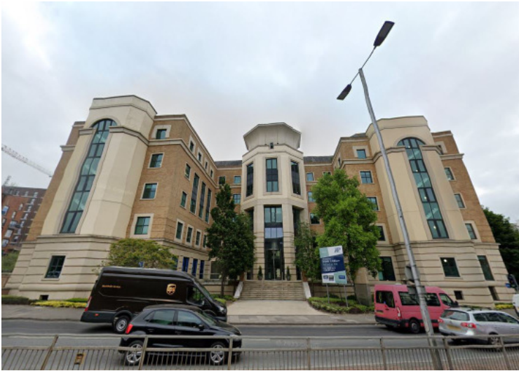
1 - Front elevation viewed from Forbury Road
