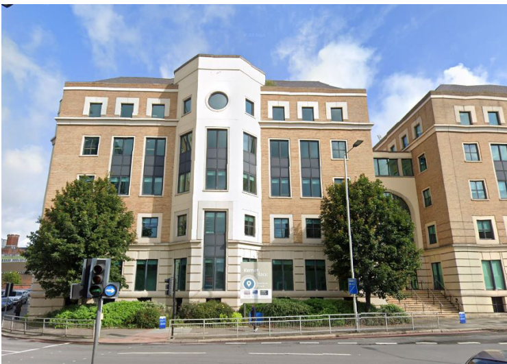
3 - South Elevation viewed from Kings Road
