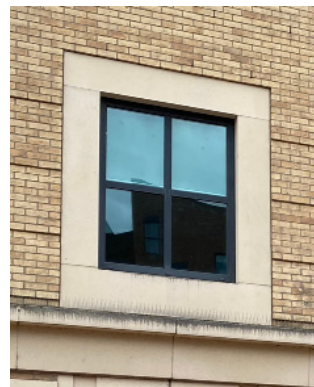
Example of existing windows to be replicated at Ground Floor
