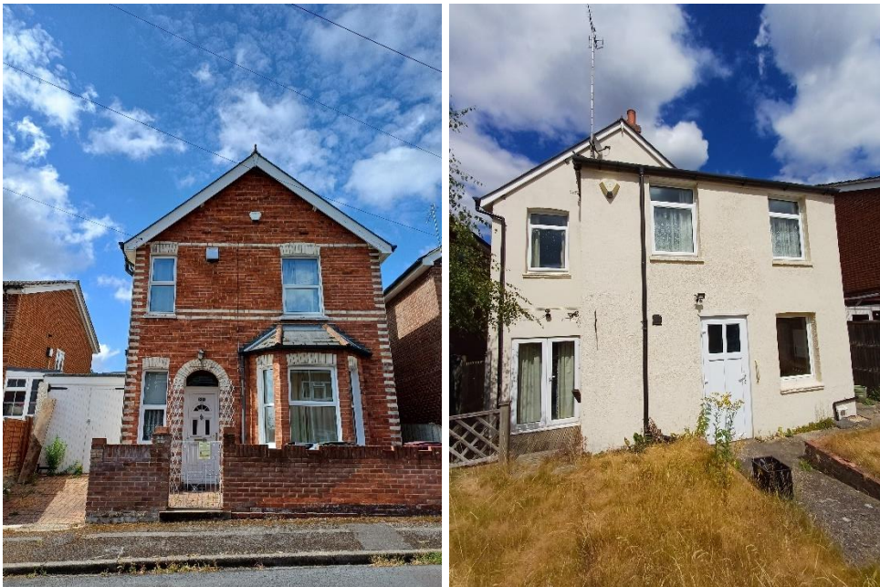
Fig 1 & 2: Views from the front and rear of the property (18/07/25)
