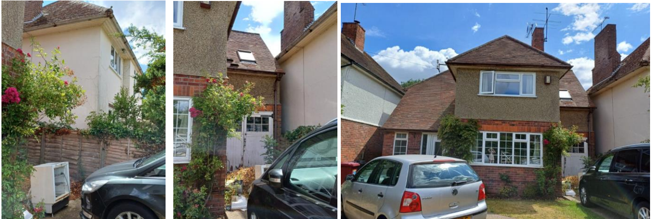
Figures 5, 6 & 7: Site photographs showing the relationship with No. 140 Westwood Road
