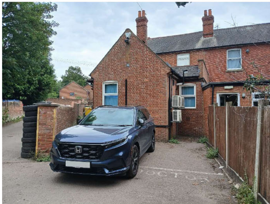
Photograph 14: The rear external wall which will have a window inserted to match the one adjacent, mirrored on the centre-line of the gable
