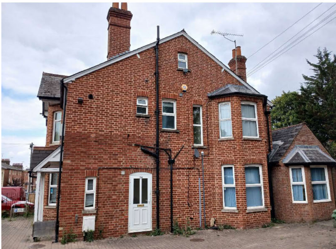
Photograph 3: The building viewed from the side (south) showing the access door into the first floor flat, known as number 79A.
