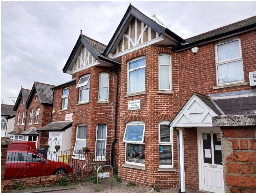
Photograph 2: The surgery and adjoining building viewed from the front (west)
