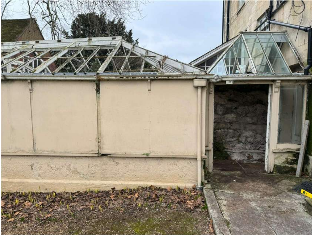
Photograph 35 – Glass wall above brick plinth protected by ply sheeting
