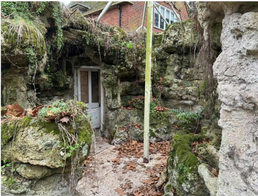
Photograph 6 – Temporary timber prop
