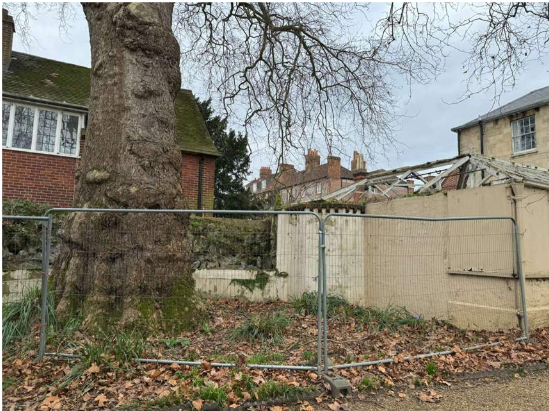
Photograph 2 – Southern wall and mature London Plane around 4.0m away.
