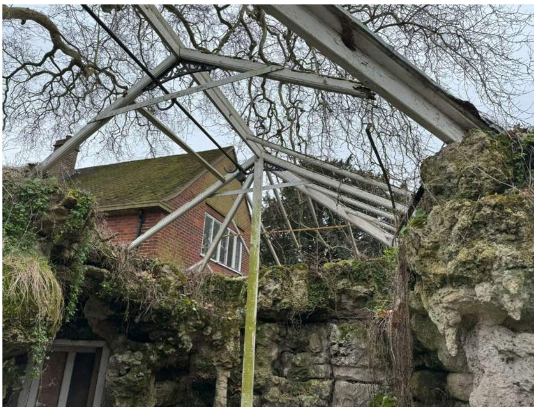
Photograph 15 – Temporary timber prop supporting end principal frame.
