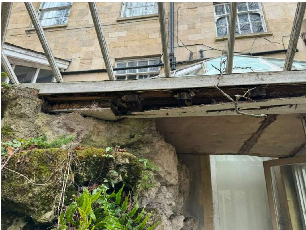
Photograph 30 – Boxed in steel beam along valley gutter
