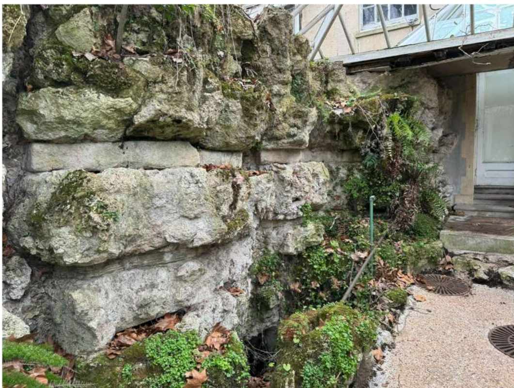
Photograph 22 – Pulhamite wall cast along western wall.
