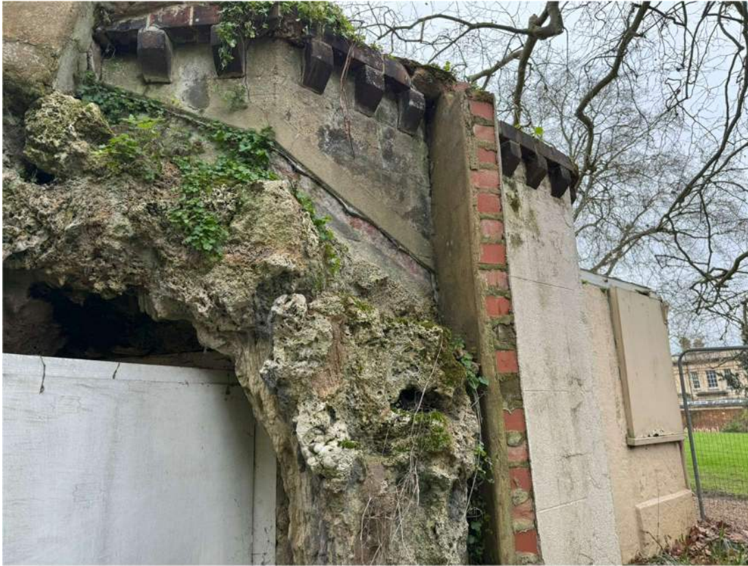
Photograph 39 – Brick cheek wall, Remnant of earlier removed glazed wall along corridor.
