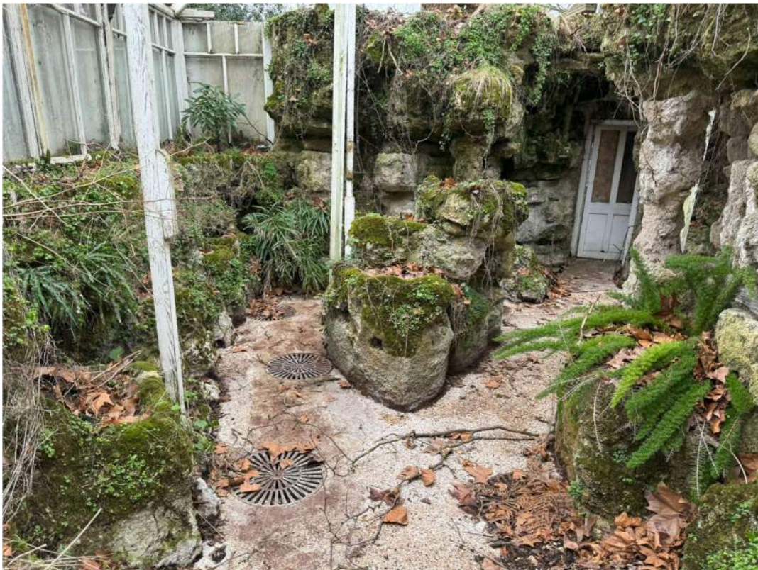
Photograph 4 – Fernery floor with cast iron duct within the terrazzo concrete slab.
