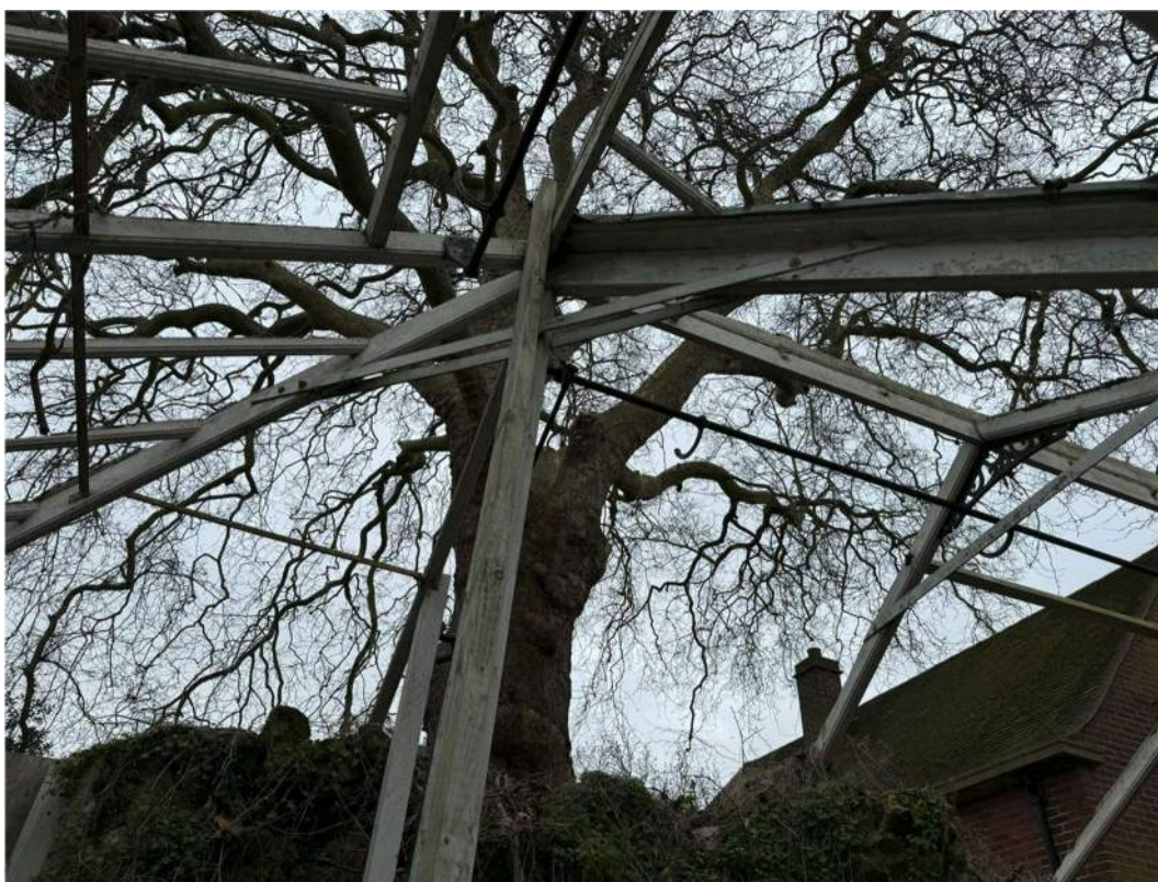
Photograph 16 – Temporary timber prop and face fixed steel straps each side of principal rafter.
