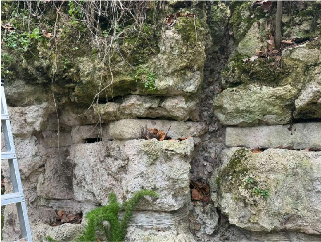
Photograph 23 – Vertical channel formed in Pulhamite wall. Potential location of high level water supply.
