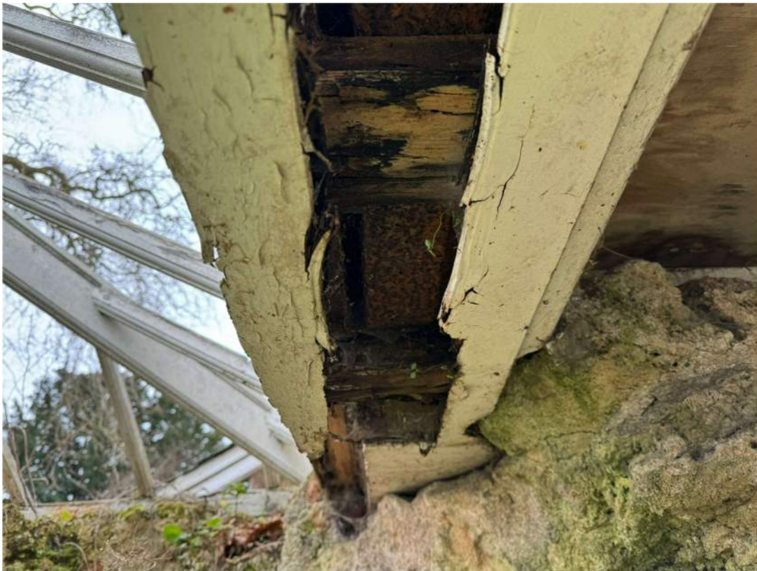
Photograph 32 – Some surface rusting to steel valley beam
