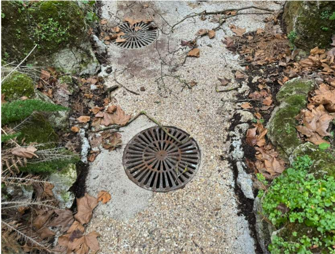
Photograph 5 – Cast iron floor duct part of the original heating and water management system.
