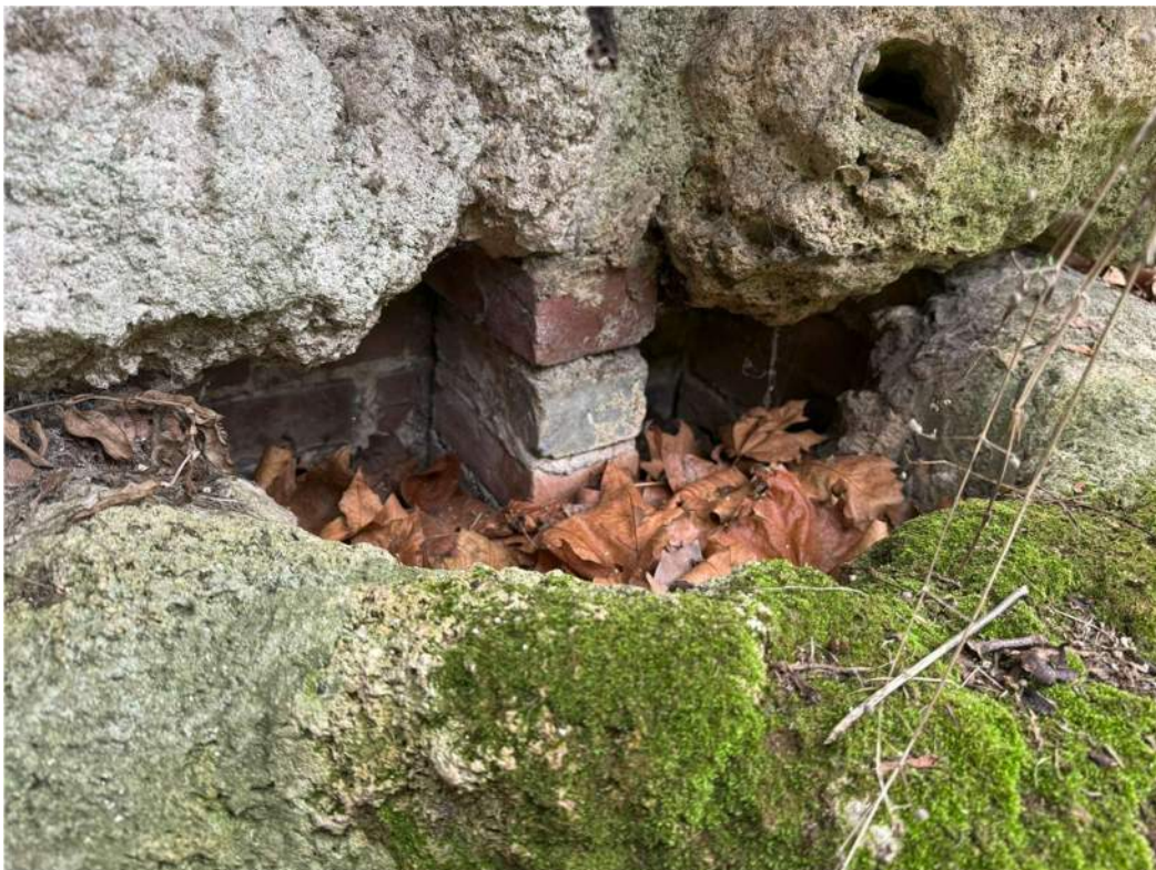
Photograph 28 – Brick supporting structure with Pulhamite and brick wall beyond.
