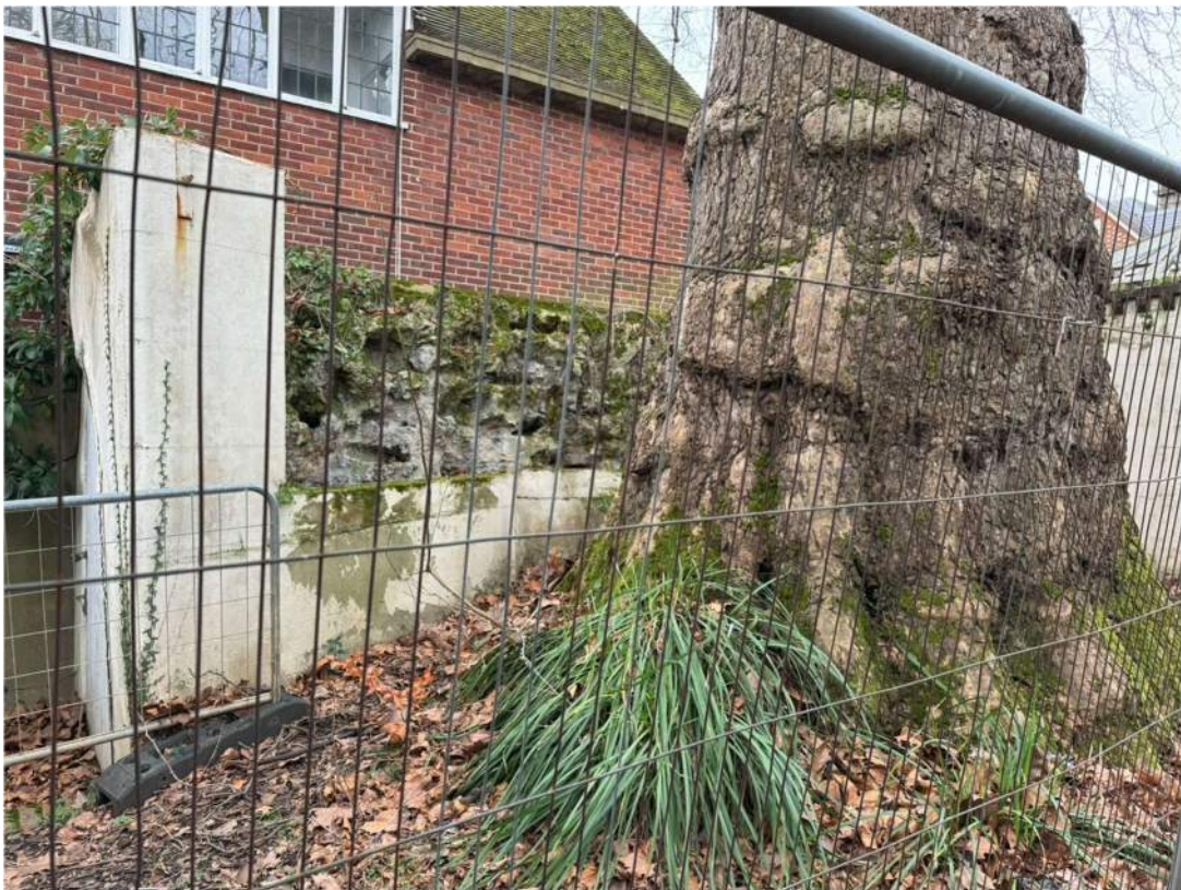
Photograph 50 – Large and mature London Plane tree very close to the corridor wall.
