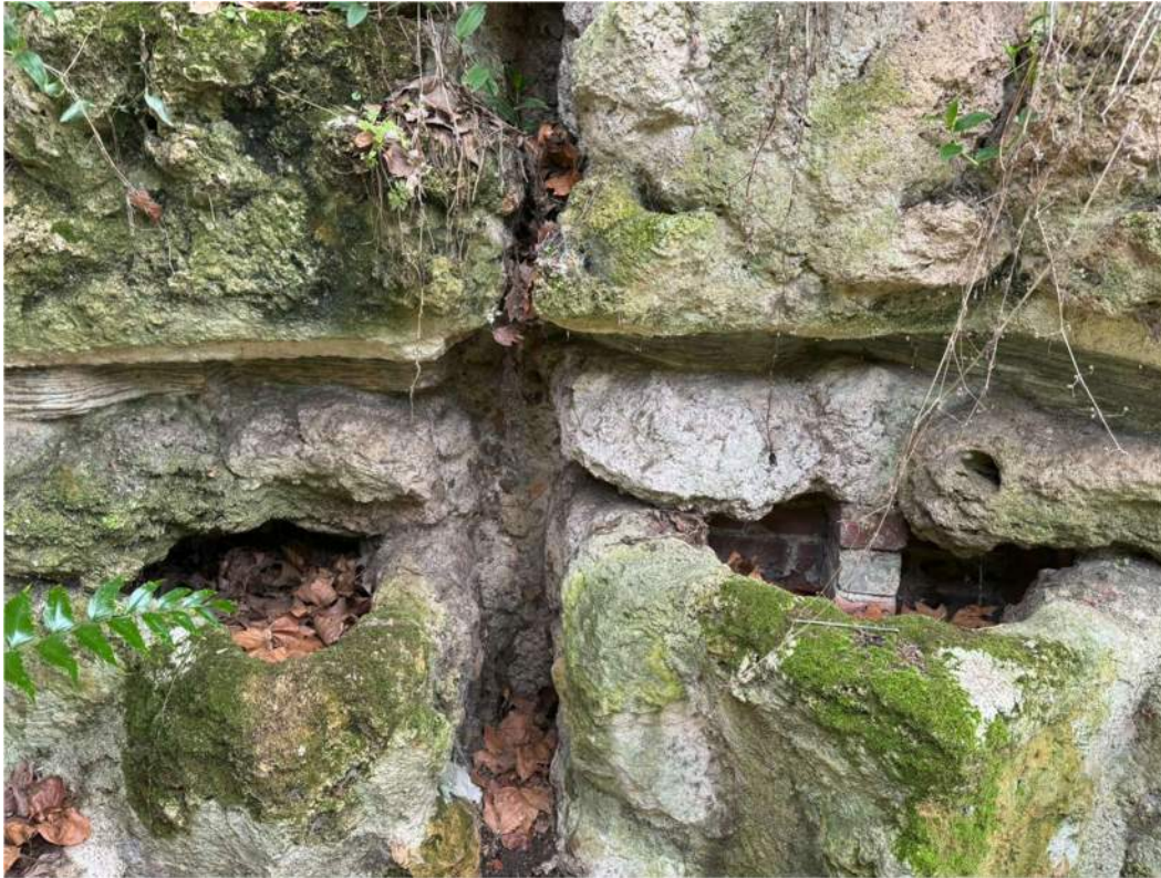
Photograph 27 – Channel for water distribution within Pulhamite and brick wall and supporting structure beyond/
