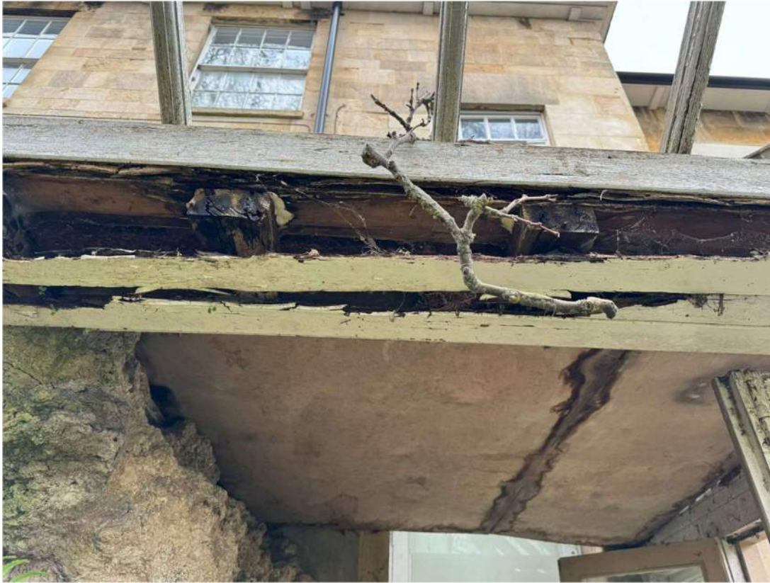
Photograph 31 – Boxed in steel beam and ply timber soffit crash deck
