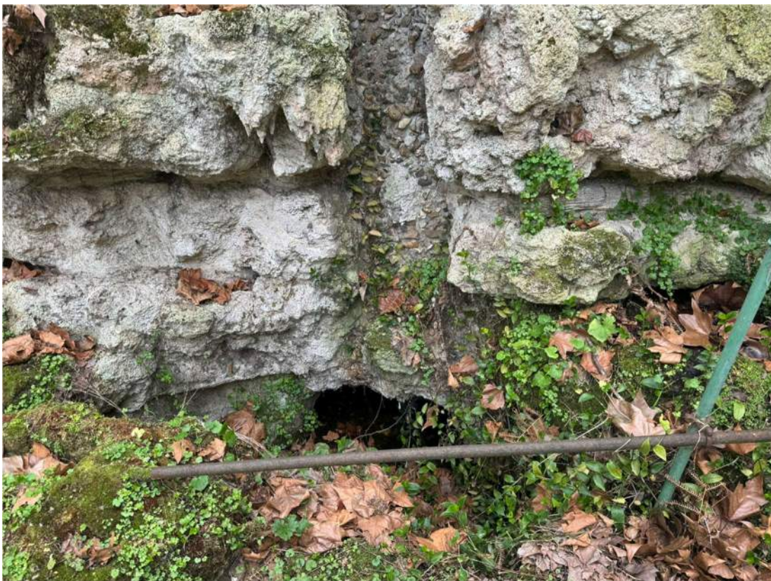
Photograph 24 – Base of vertical channel leading to water pool, part of original recirculation system.
