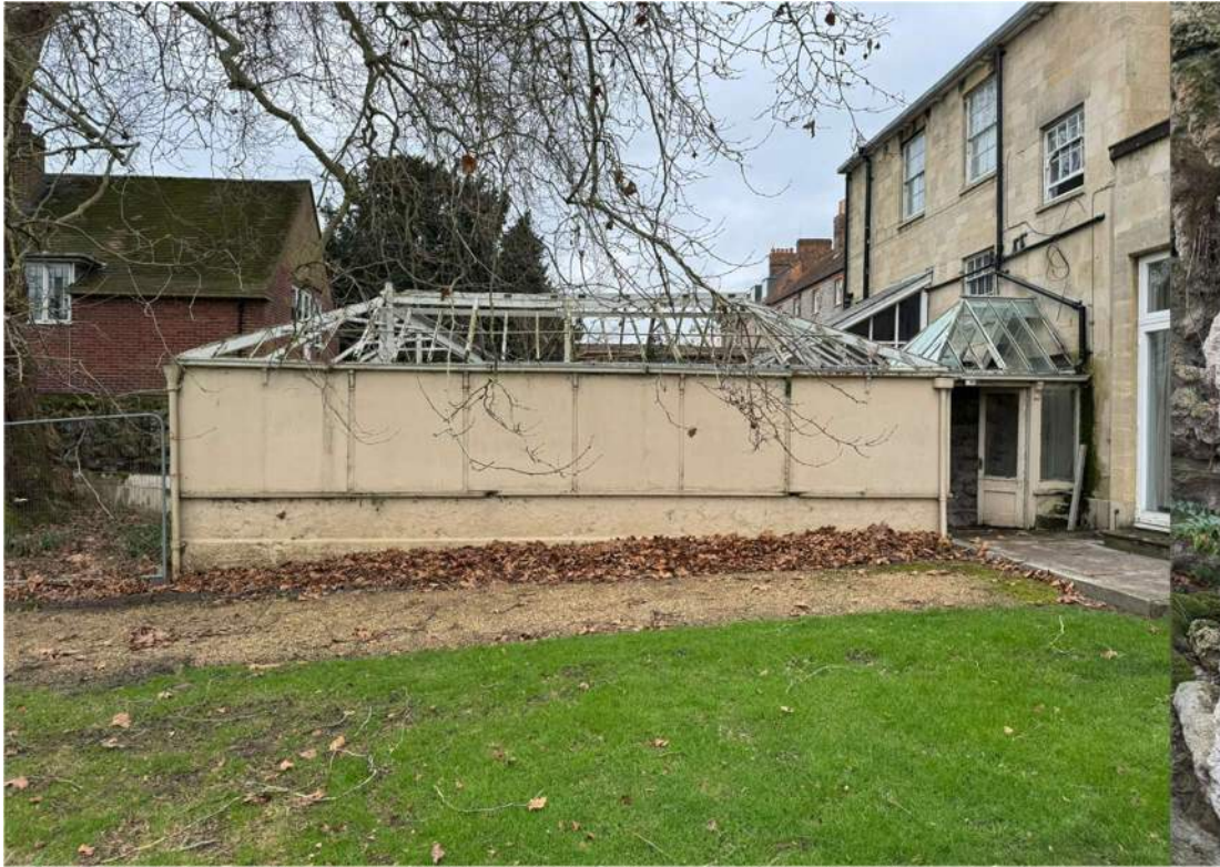
Photograph 1 – East facing wall to the Fernery. Note original glazed wall now protected with temporary boarding.
