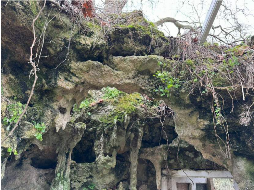
Photograph 7 – Pulhamite arch over walkway. No signs of distress.
