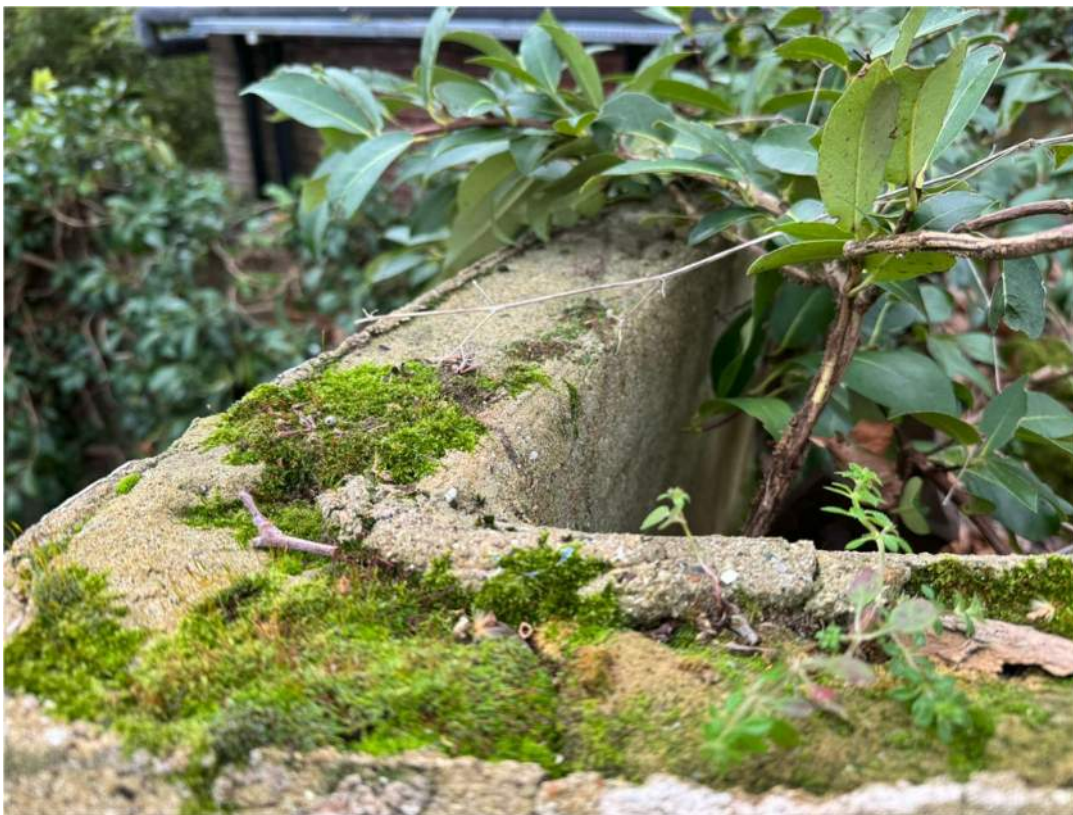
Photograph 48 – Channel for missing timber wall plate above entrance arch. Remnant of earlier glazed roof.
