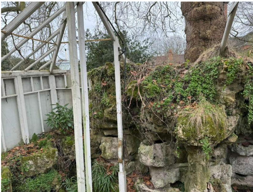
Photograph 14 – High level wall plates hidden behind Pulhamite walls.
