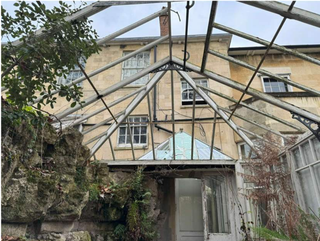
Photograph 8 – Pitched roof structure looking north towards the villa. All glazing has been removed.
