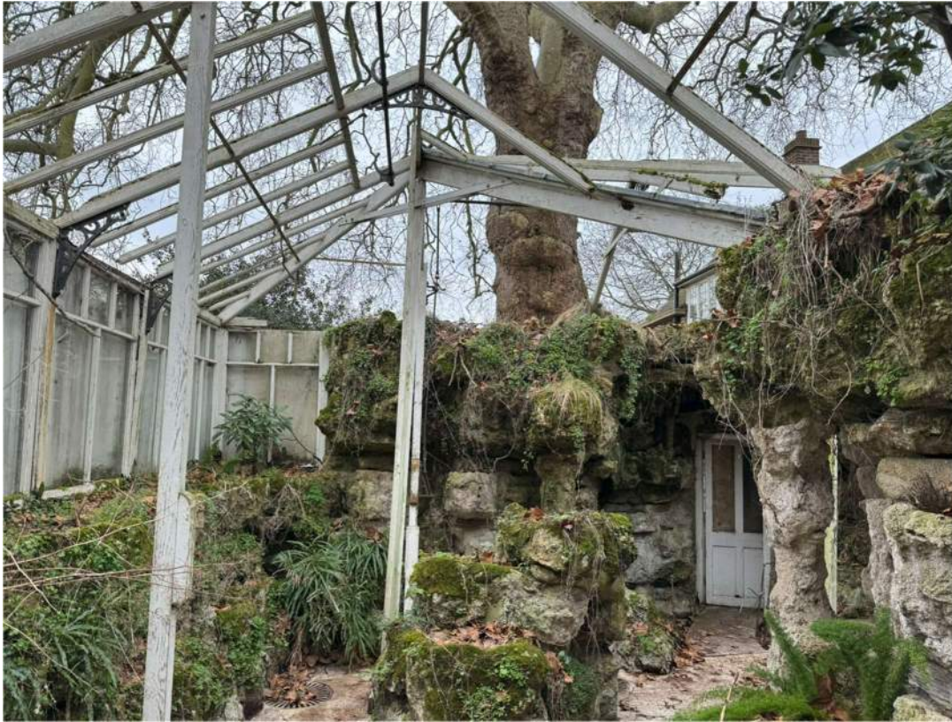
Photograph 3 – Internal view of the Fernery facing south. Note temporary central prop for hip frame.
