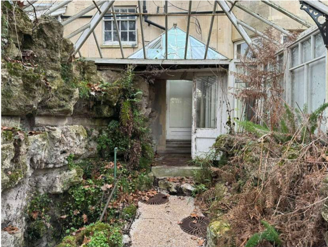
Photograph 9 – Porch structure to the north with glazing still in place but protected by plywood soffit below.
