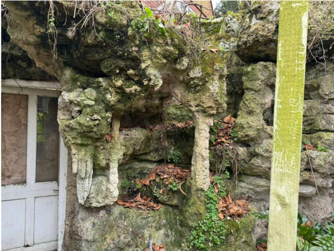
Photograph 25 – Pulamhite arch across door with hidden wall plate above
