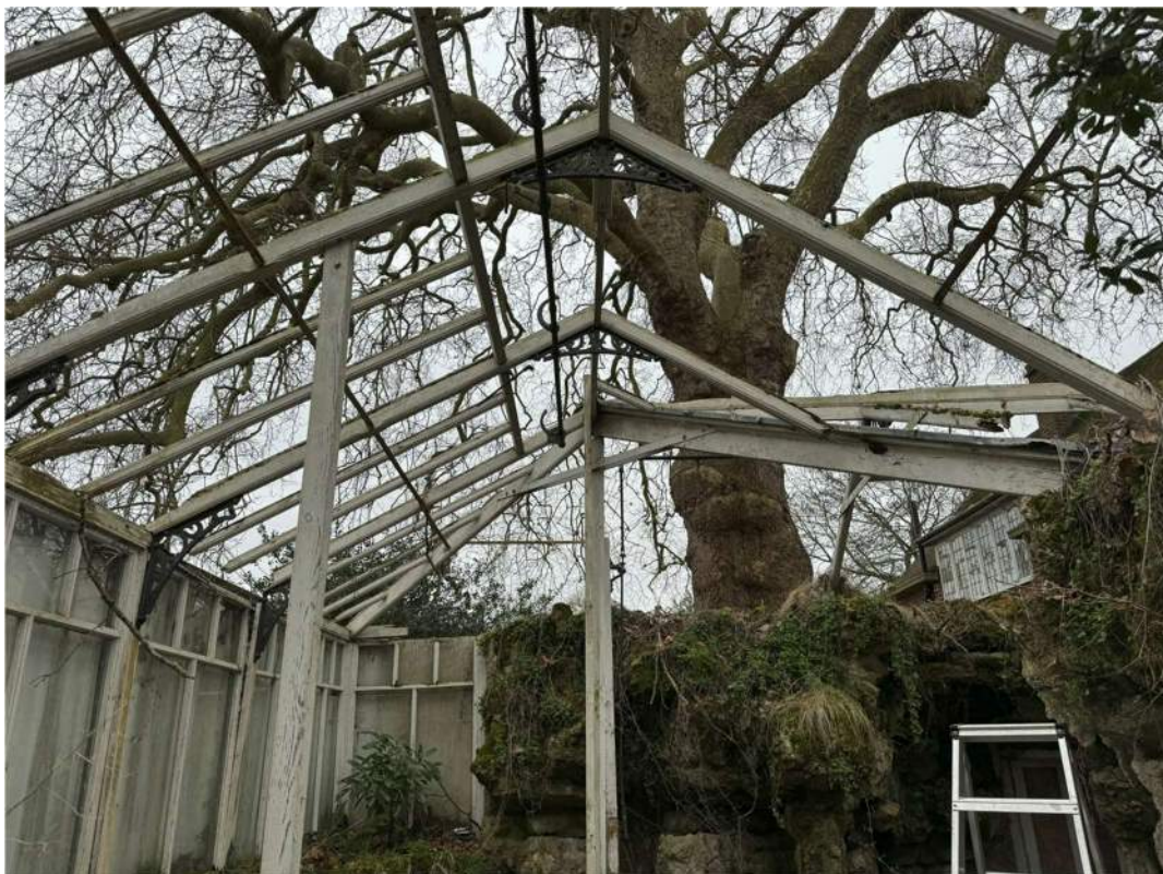
Photograph 21 – Glazing bars previously removed from western pitch
