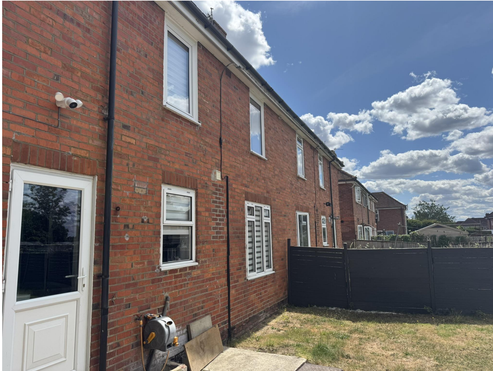
Site Visit Photos , taken on 3 rd of July 2025
