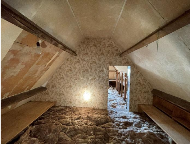
Photograph 7. The central section of the loft space. *
