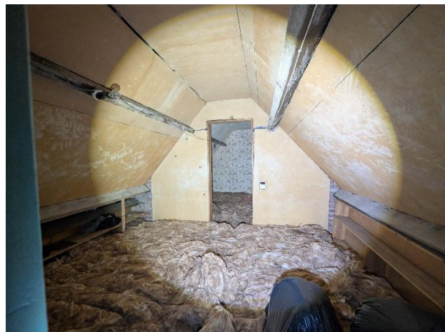
Photograph 6. The central section of the loft space.
