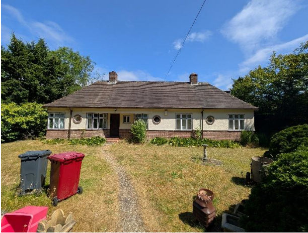
Photograph 1. The southern elevation of the dwelling.
