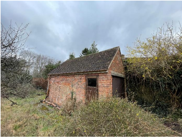
Photograph 9. Outbuilding/store viewed from the south-west. *
