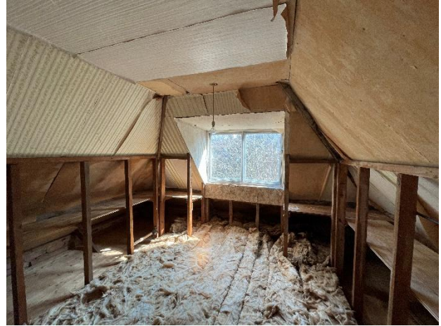
Photograph 8. The eastern section of the loft space. *
