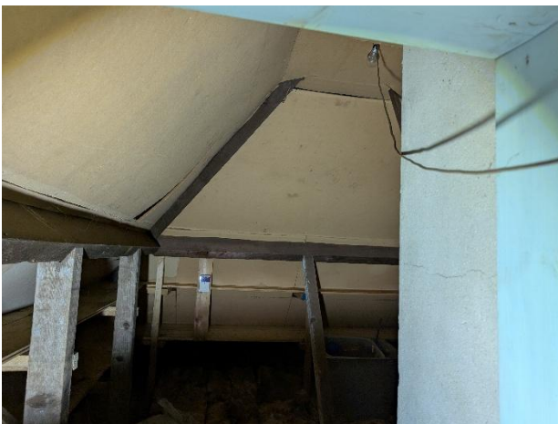
Photograph 5. The western section of the loft space.
