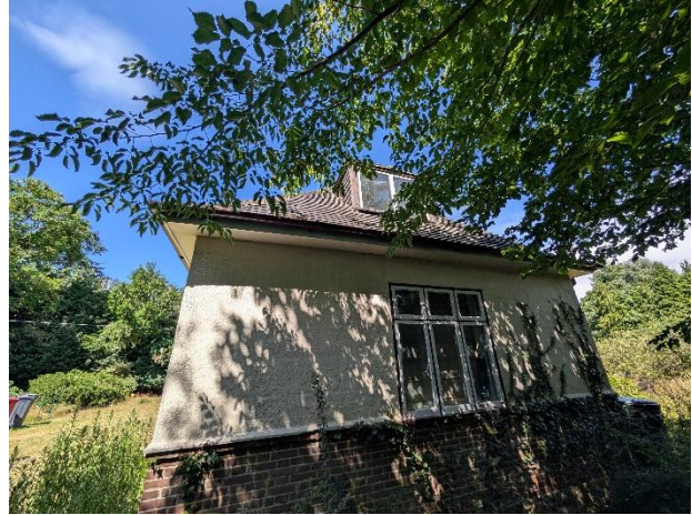
Photograph 2. The eastern elevation of the dwelling.
