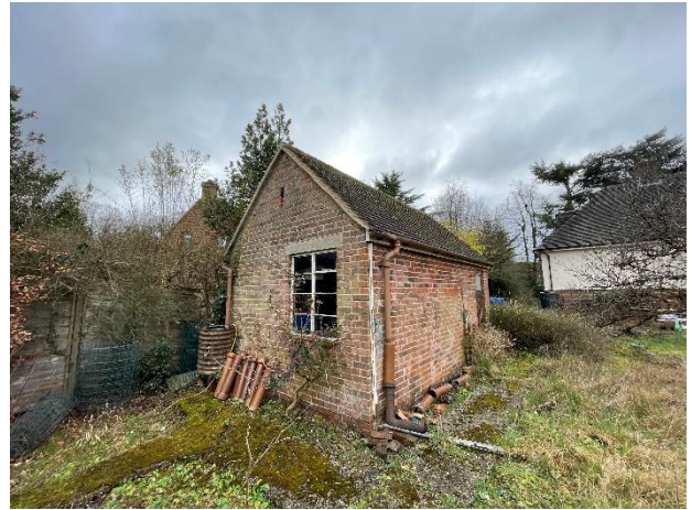
Photograph 10. Outbuilding/store viewed from the north-west. *
