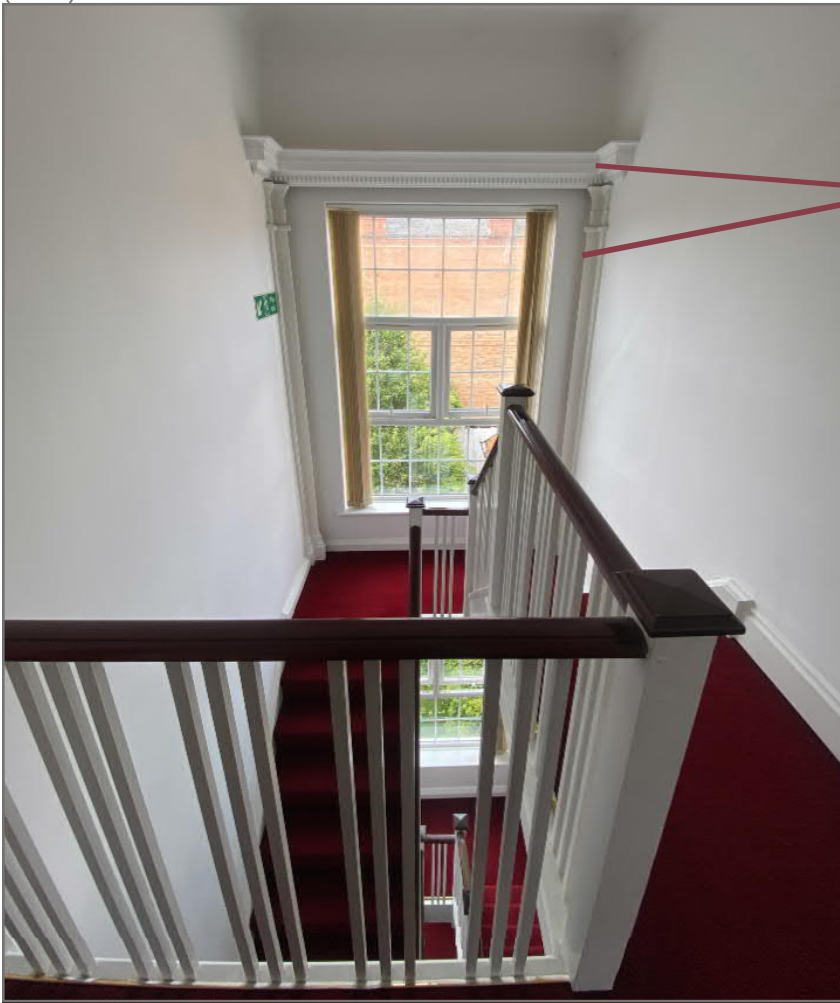
Image 39: View from Second Floor of staircase and window
