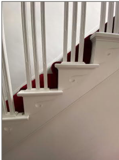
Image 25: open-string staircase: detail of treads with trio of square profile balusters with inset detail, set into a raised block
