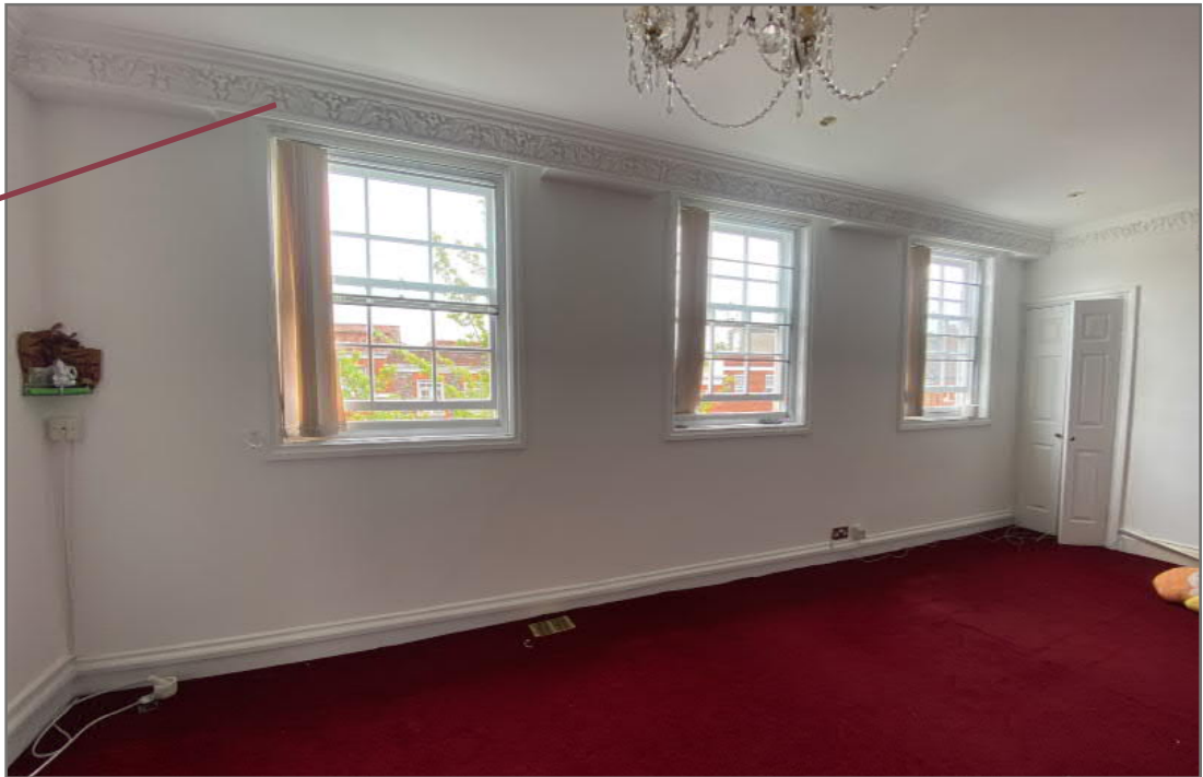
Image 41: Second Floor east room - the 'attic' floor, is likely to have originally been three rooms and would not have had a decorative cornice - reserved only for the most important reception room
