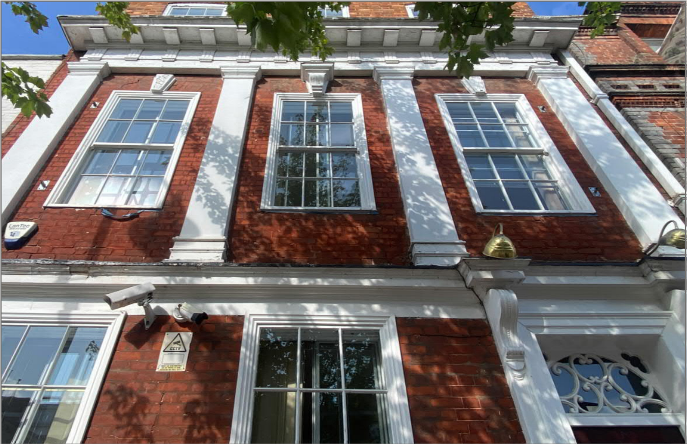
Image 18: First Floor detail of east elevation
