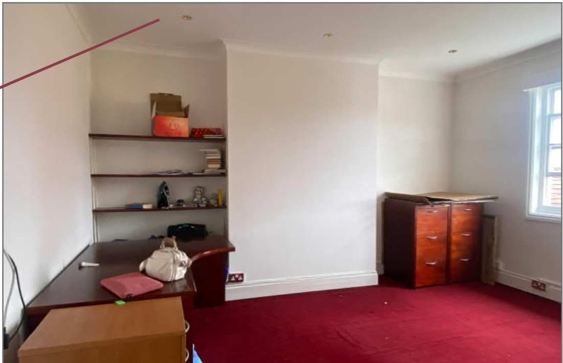
Image 42: Second Floor west room - the chimney breast and sash windows remain
