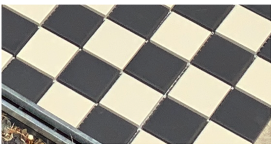
TILES TO FRONT ENTRANCE
