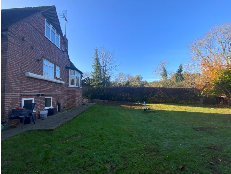
View from side boundary towards the dwelling
