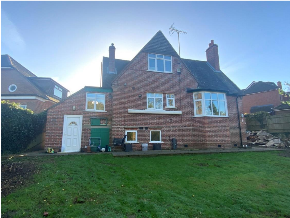
View from garden towards the dwelling
