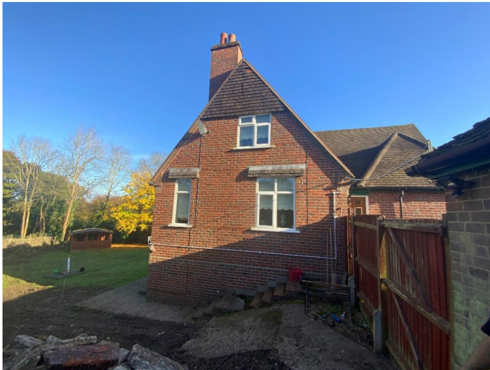
View from side boundary towards the dwelling
