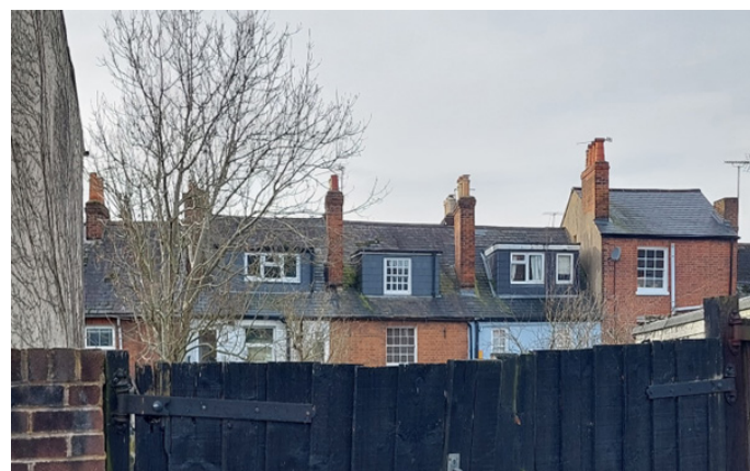
Figure 5: View from Princes Street towards existing dormer lofts at rear of properties along Watlington Street
