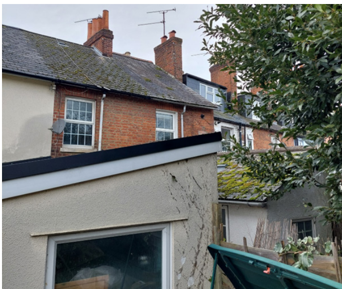
Figure 4: View from 85 back courtyard garden: existing dormer lofts north along Watlington Street
