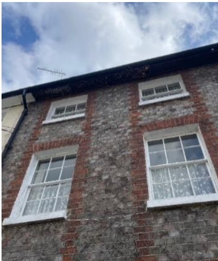
Figure 14: Example of six over six window as proposed
