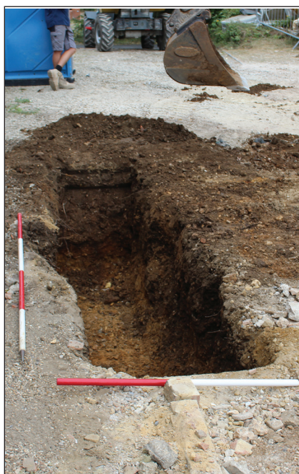
Plate 3. Northern east-west trench footing, looking East, Scales: 2m and 1m
