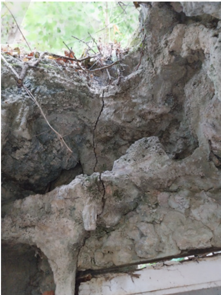
Crack in Pulhamite at south end of Fernery
