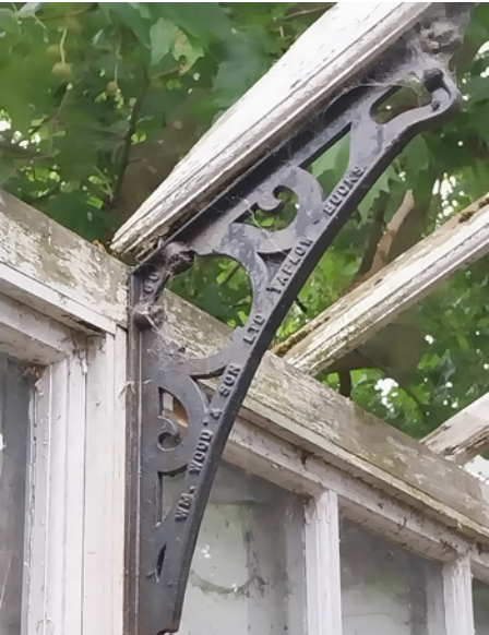
Cast iron bracket at eaves level
