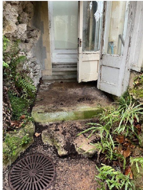
Entrance porch and door into the Acacias.
