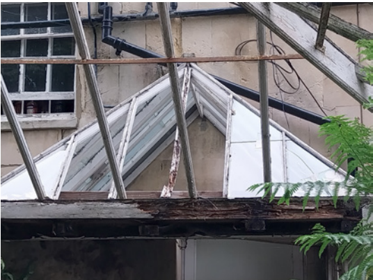
Junction of Fernery roof with porch roof
