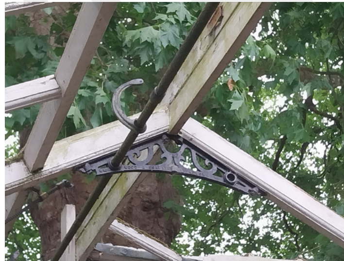
Mechanism for opening roof light
