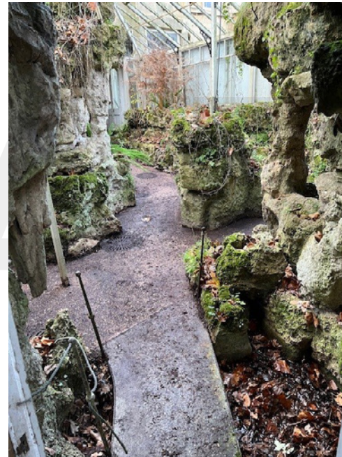
South end of the main section of the building.
