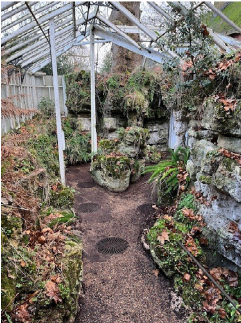
Interior of the main section of the building.
