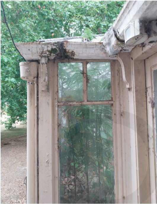
Return bay on east side of Fernery
