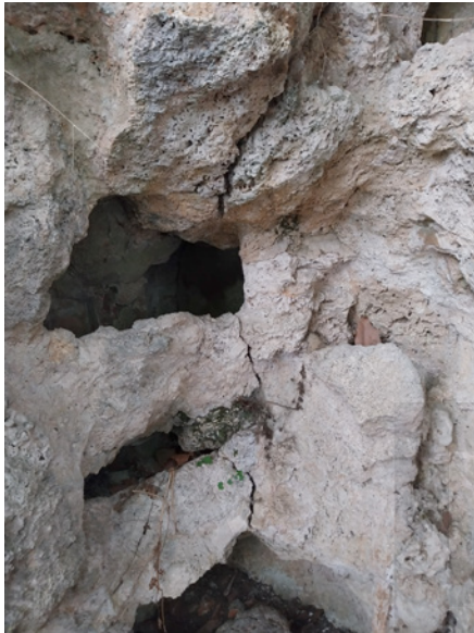
Crack in Pulhamite at south end of Fernery
