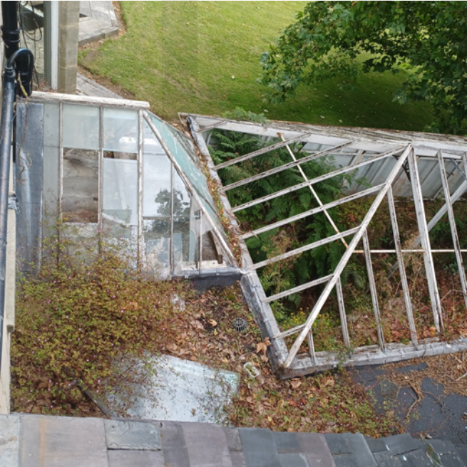
Roof seen from rear of the Acacias
