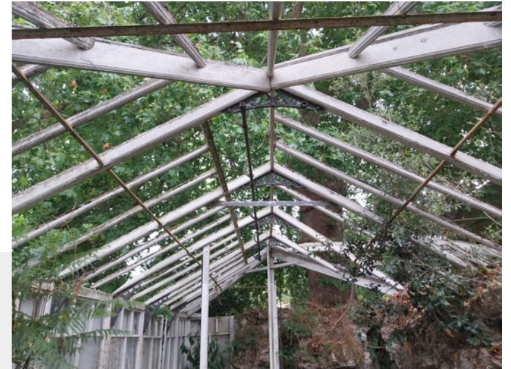
Ridge line of the roof
