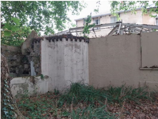
Exterior of south end of Fernery
