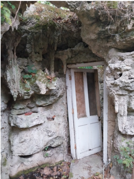
Pulhamite rockwork at south end of Fernery
