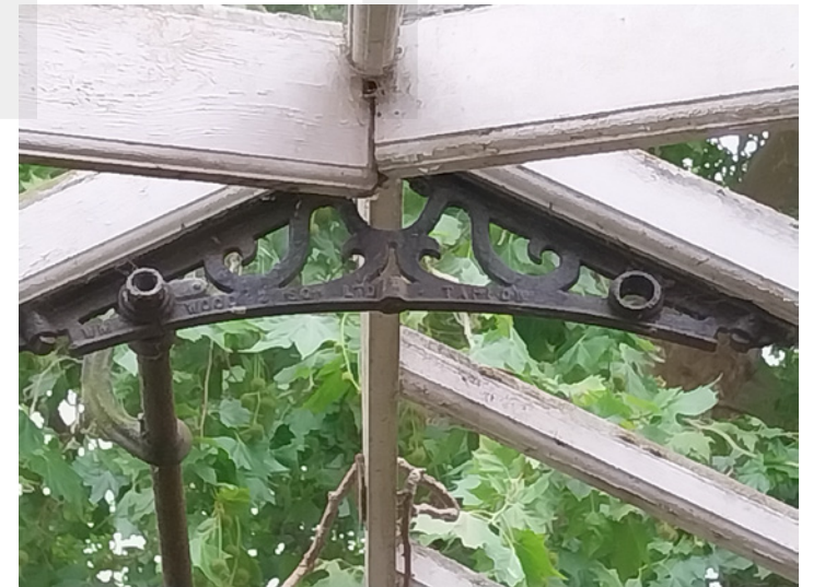
Cast iron bracket below the ridge
