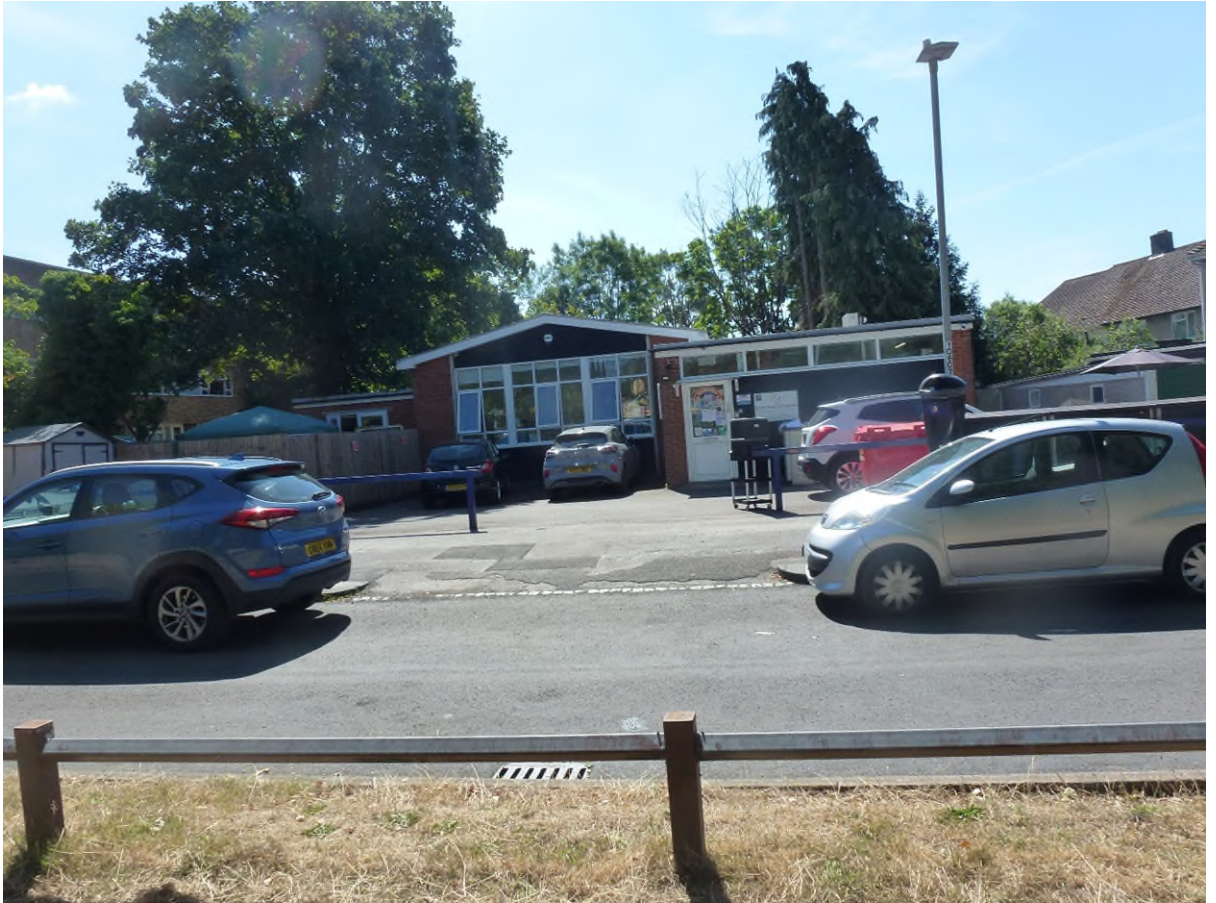
Photograph 2 The Existing Nursery on Grove Road (Service Road)
