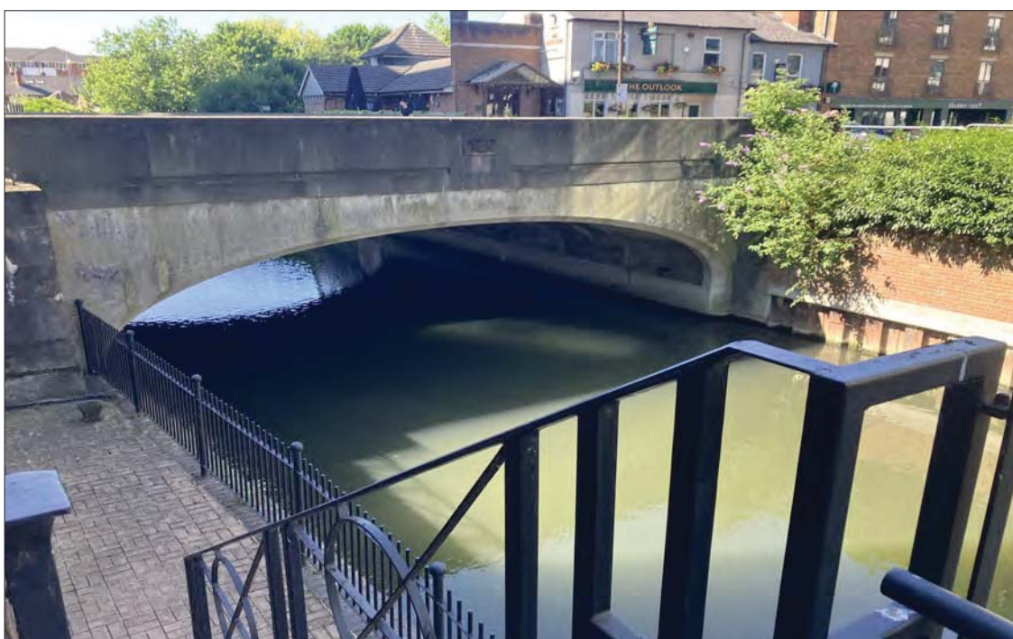
Photo facing south showing river tunnel beneath Kings Road to the southwest of the site
