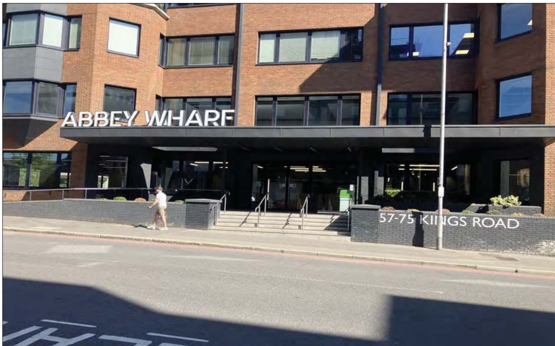
Photo facing north showing entrance to the existing building
