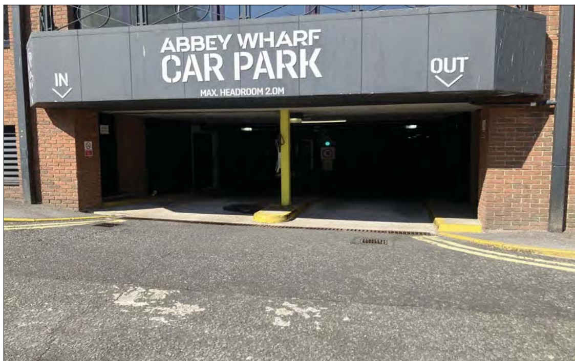
Photo facing west showing basement carpark access on east of the site
