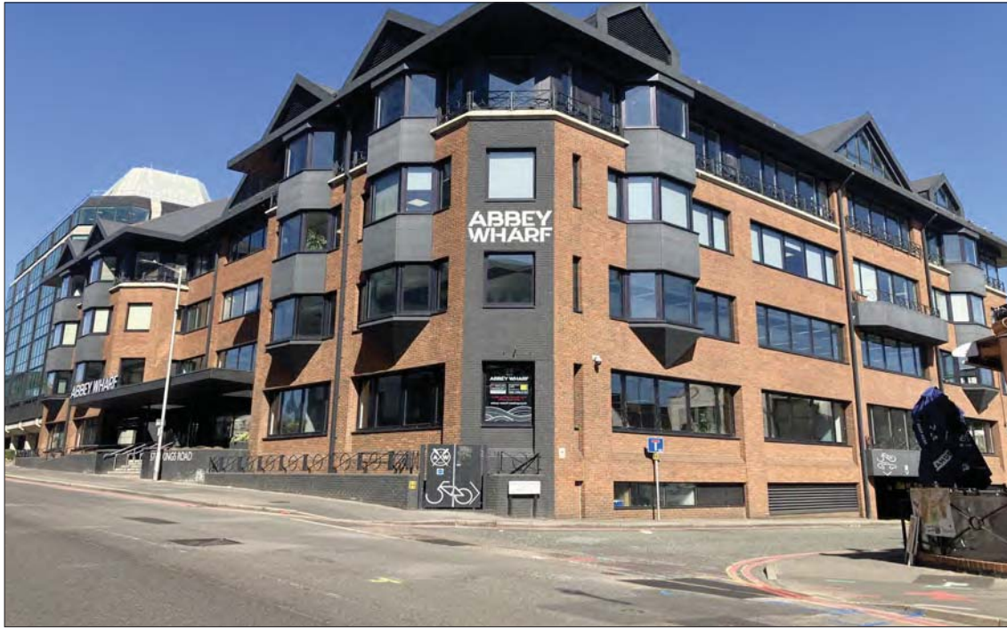
Photo facing northwest showing existing five storey building
