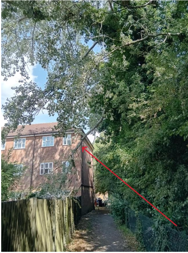
Figure 2 - T11 broken limb resting on the fence
