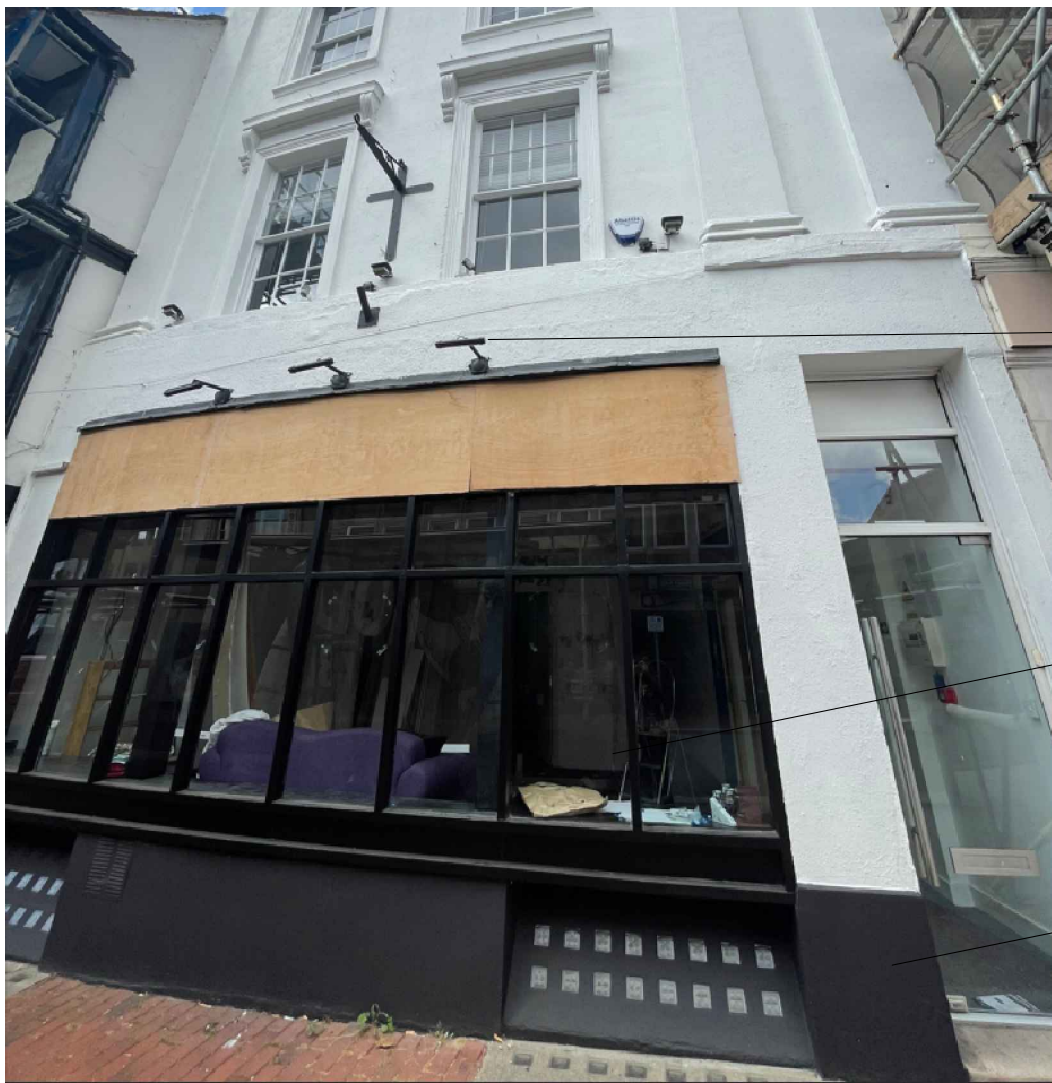
Current view of Front Elevation
