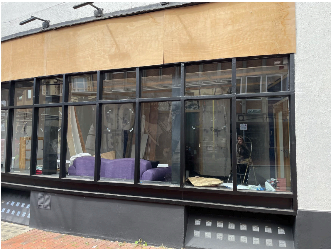
Image 06 Front shop window frame and plinth below have been painted black matt. The existing signage lights will remain. A new sign board and window film will be applied for under a separate Advertisement consent application.
