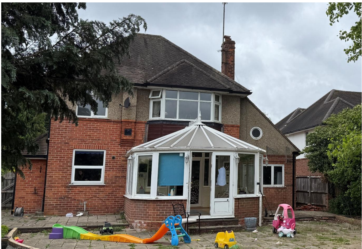
Existing Rear Extension
