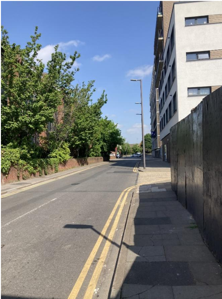
Figure 3 Existing Highway Conditions on Eaton Place
