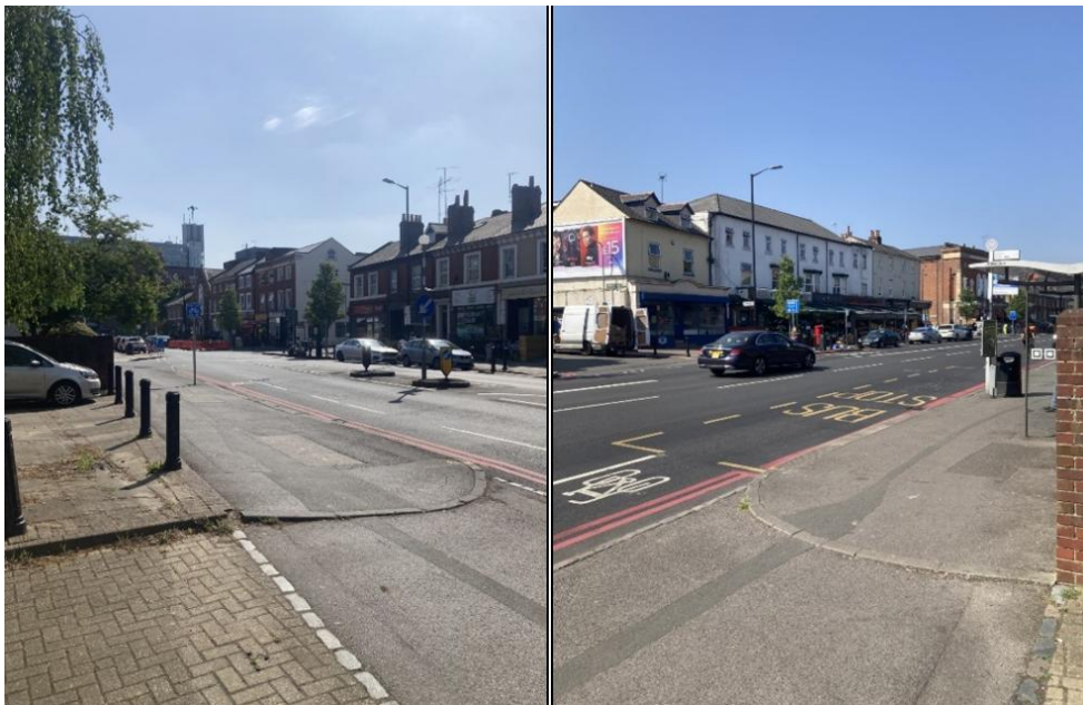
Figure 2 Existing Highway Conditions on Oxford Road
