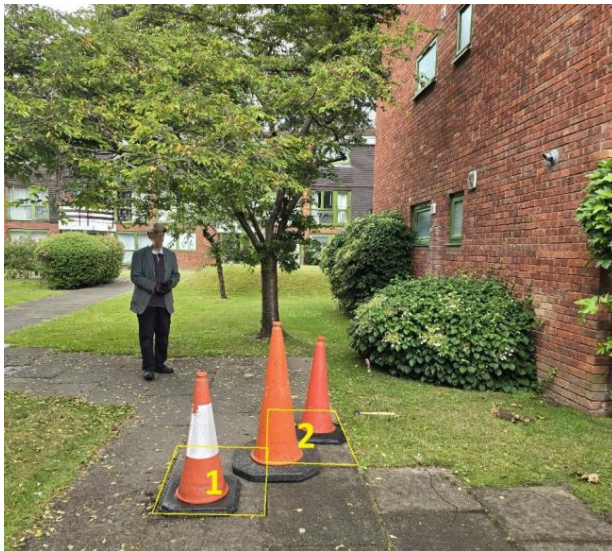
Figure 1 - Paving Slab 1 and Paving Slab 2
