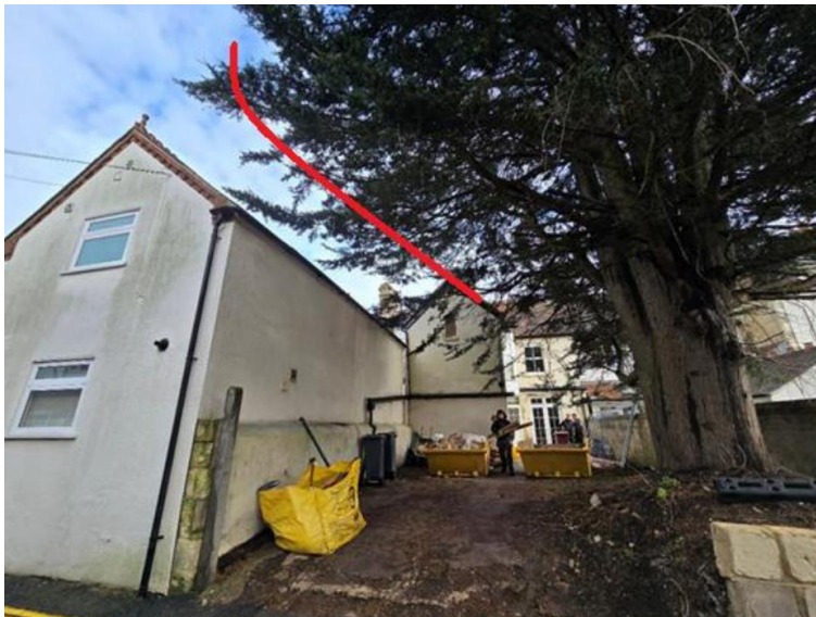
Figure 1 - North Canopy Selective Branch Reduction
