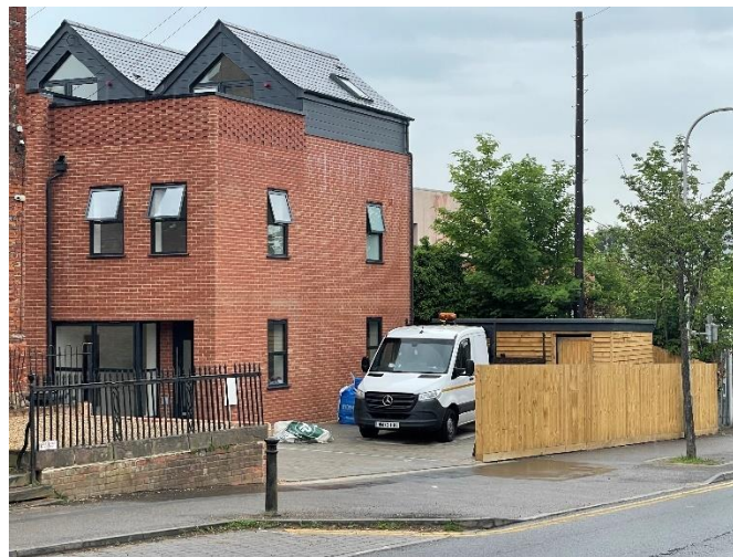
Figure 2 - Site as at 21 May 2025
