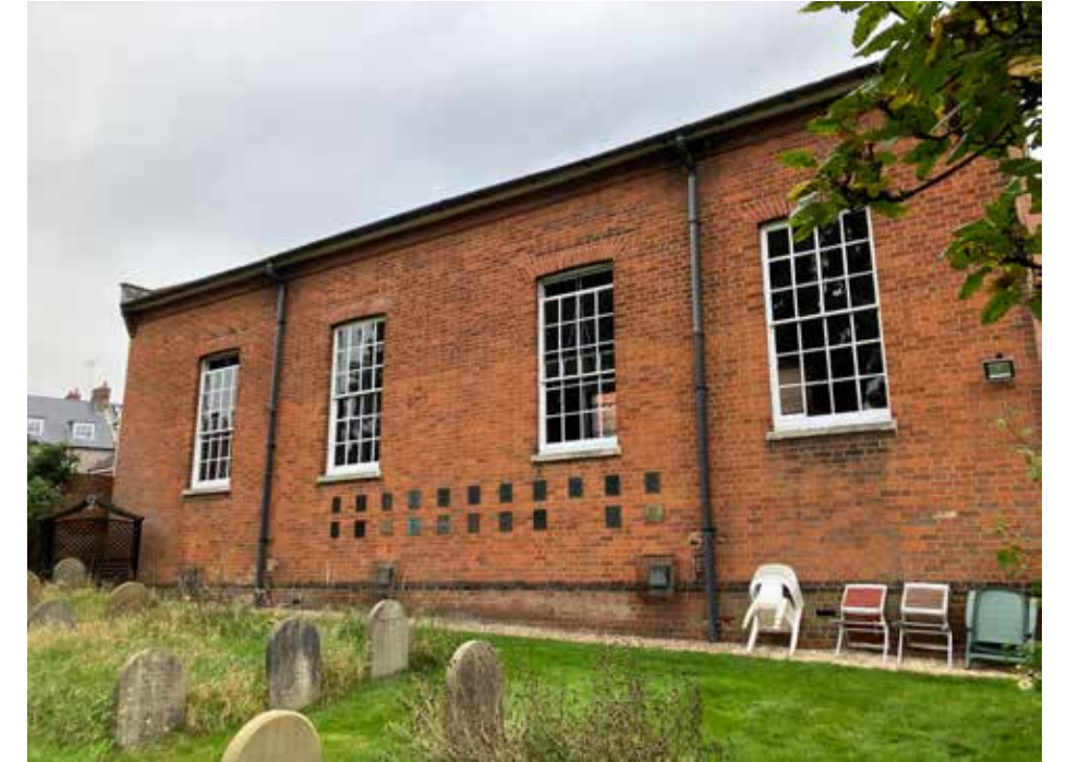
Figure 5.7 Rear elevation of the Quakers Meeting House
