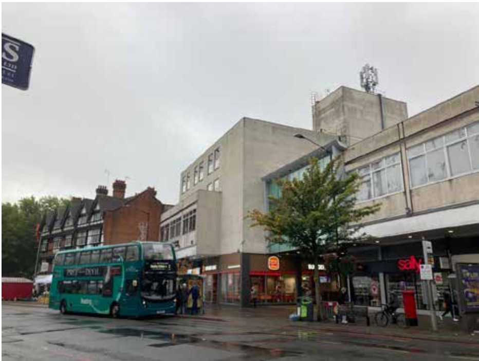
Figure 6.9 Broad Street Mall within Reading town centre
