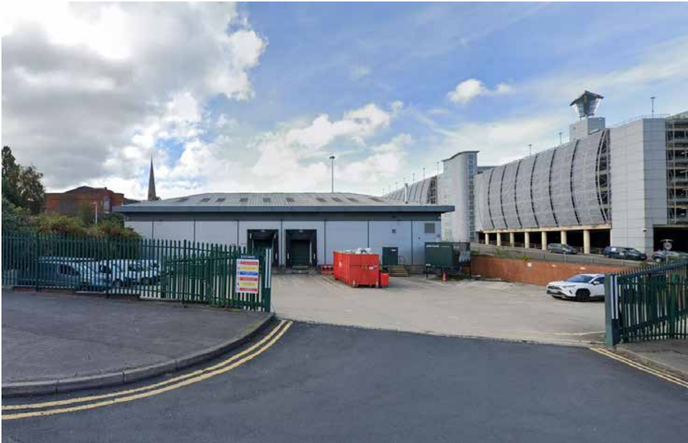
Figure 1.3 Current building on Site. Source: Google Street View October 2020.
