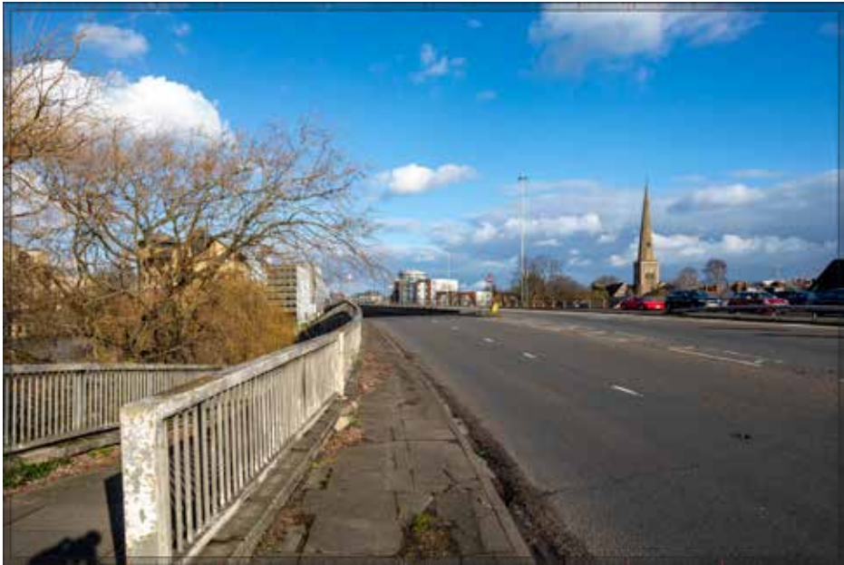
Figure 7.8 View 9: Bridge Street/A329 looking east. Source: Cityscape
