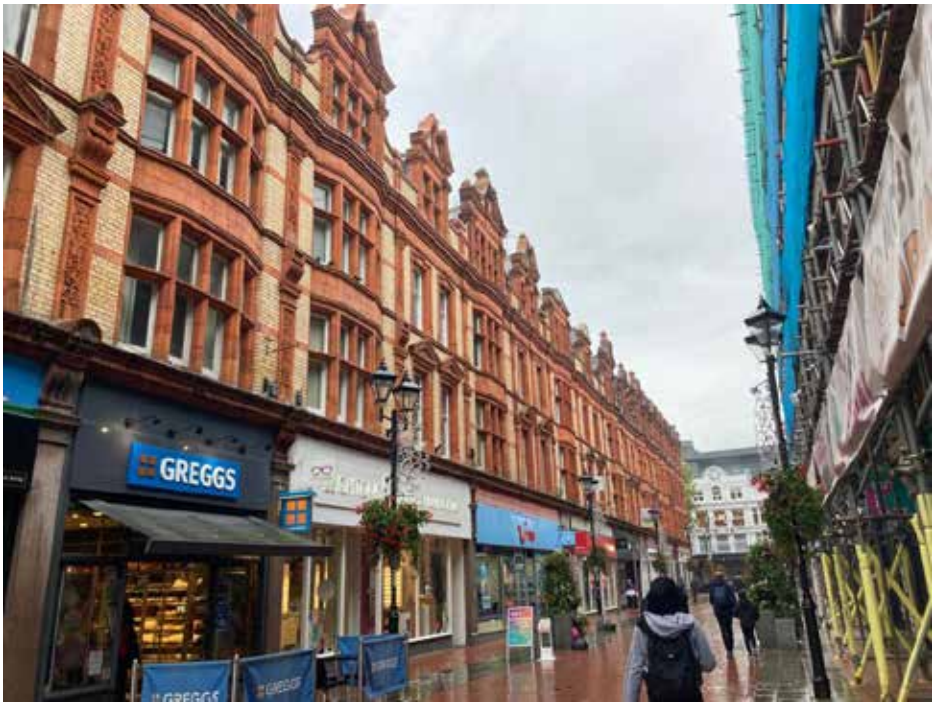
Figure 6.8 Historic buildings within Reading town centre
