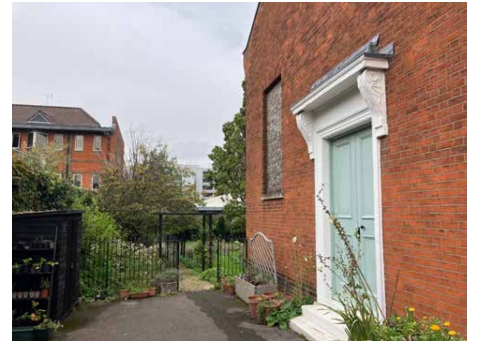
Figure 5.8 Main entrance to Quakers Meeting House and relationship with the burial ground to the north
