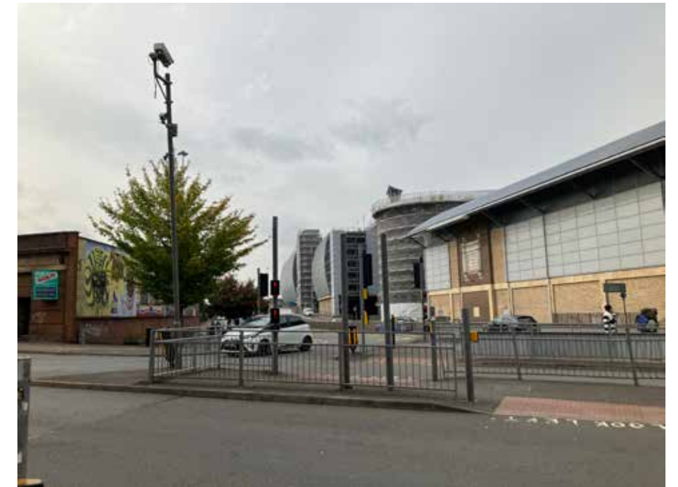
Figure 6.3 The Oracle Shopping Centre and associated multi-storey car park on the northern side of the IDR.
