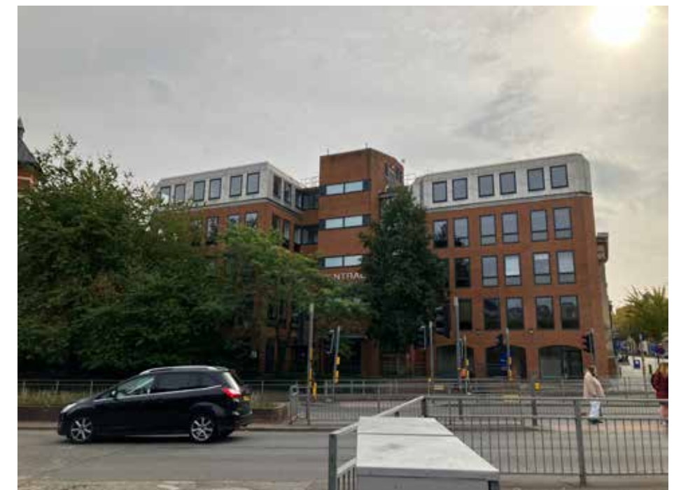
Figure 6.4 Commercial development on the southern side of the IDR.
