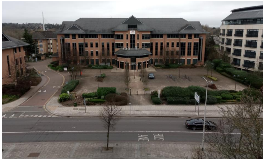
Site photograph looking north from the multi-storey car park roof to the south (20/02/2024)
