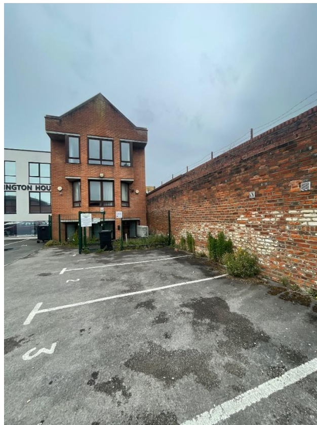
Figure 3: Application Building – Rear Elevation
