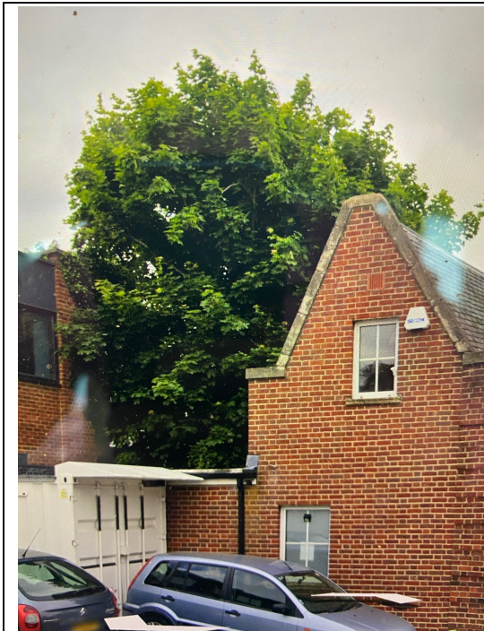
Fig. 3. Image of T1 courtesy of Google Street View
