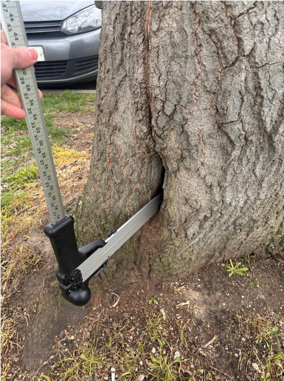
Figure 3 Cavity at base of T5.
