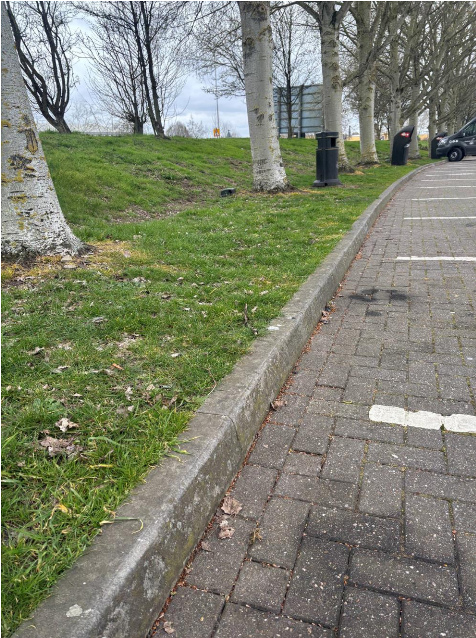
Figure 2 T1 through to T6. No evidence of root deflection on curb or hardstanding.
