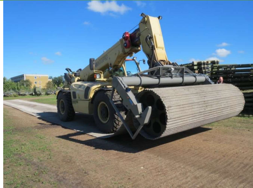
Fig.3: Examples of track board ground protection systems – specification will be dependent on the loading to which it will be subject.
