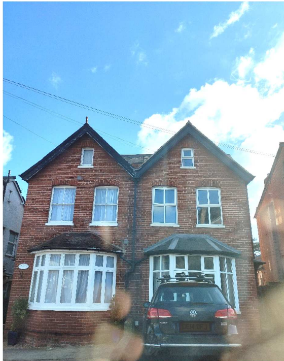
Street facing elevation (east)
