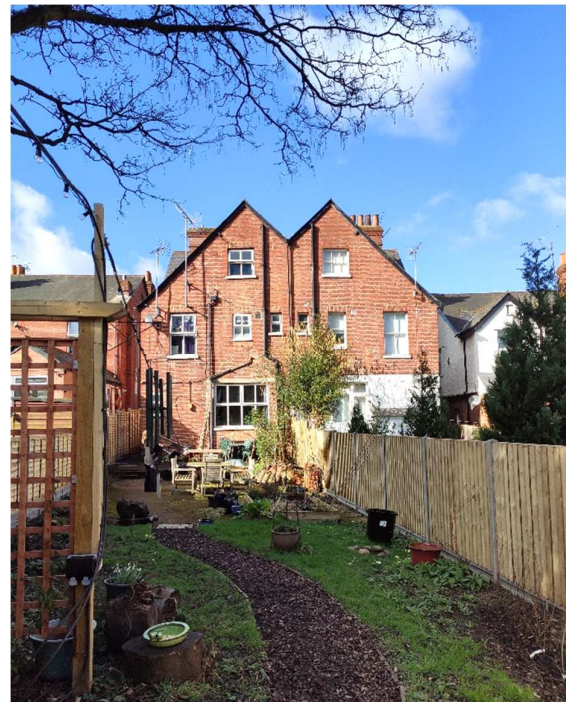
Rear elevation view from back garden (west)
