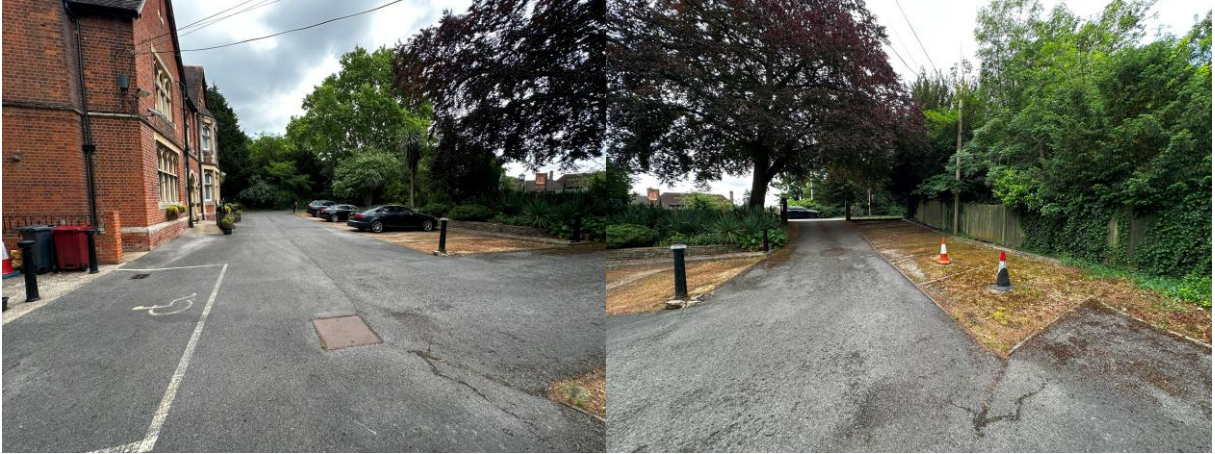
Figure 3 – Existing Car Parking
