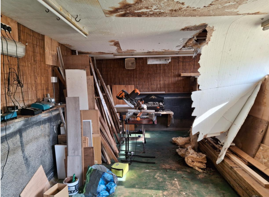
Figure 6: The internal of B2, as seen from the front (west) facing east
