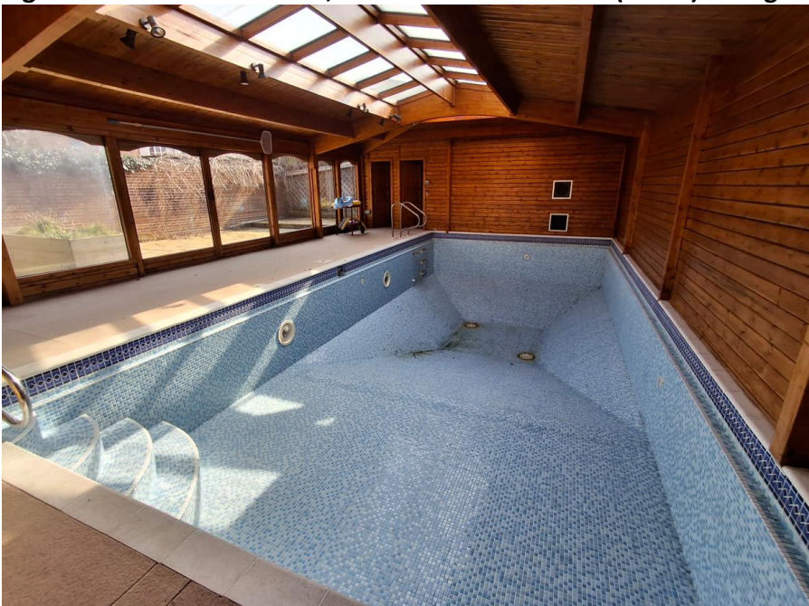
Figure 4: The internal of B1, as seen from the front (north) facing south
