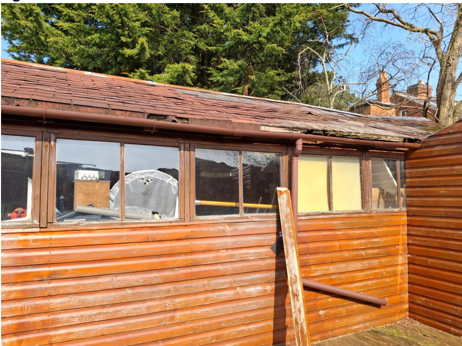
Figure 5: The south elevation of B2
