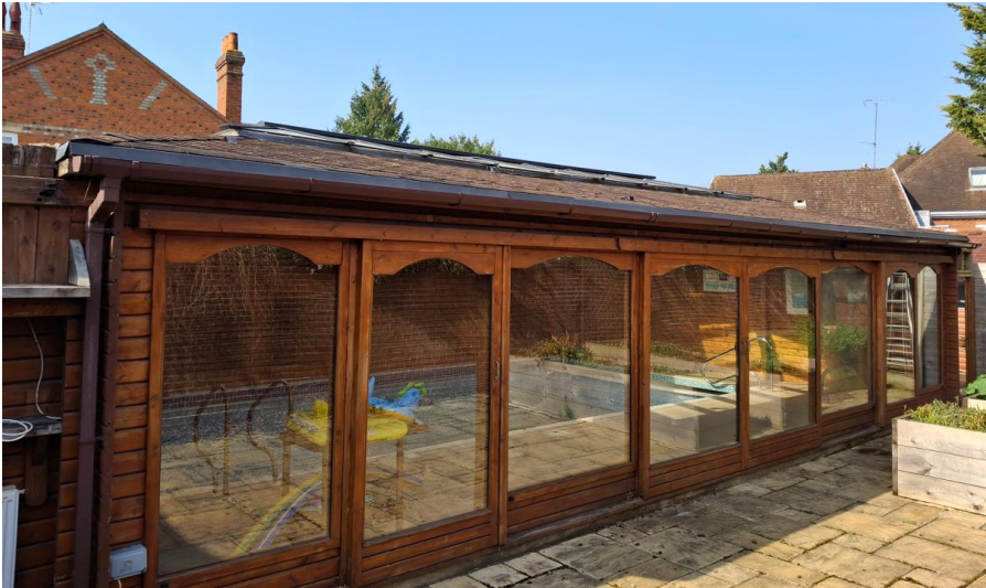
Figure 3: The east elevation of B1
