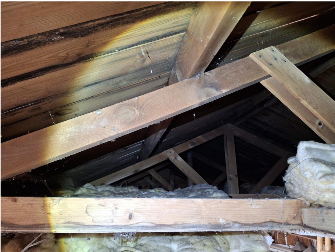
B2: loft, facing north
