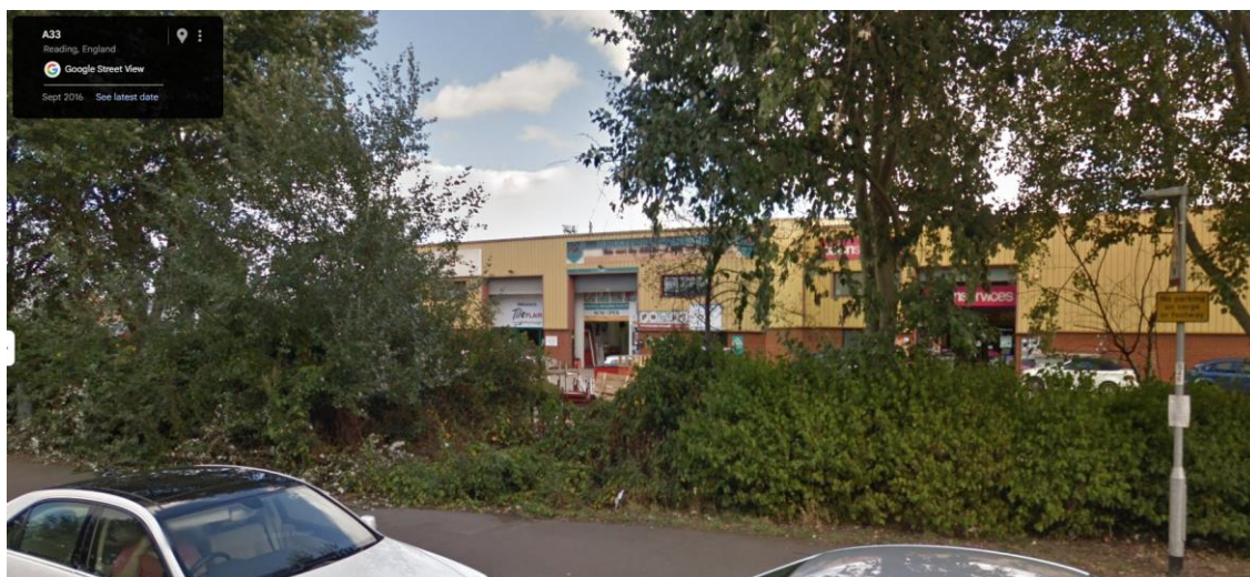
Figure 4: Unit 1b Mayfield Trade Centre - Google Street View taken in September 2016 (Source: Google Maps )
