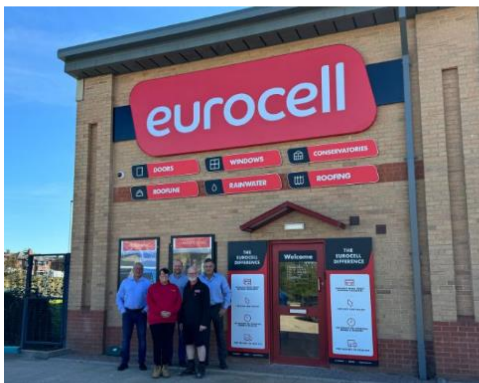
Figure 17: Customer entrance (Dewsbury). Source: Eurocell Relocates to Bigger and Better Branch
