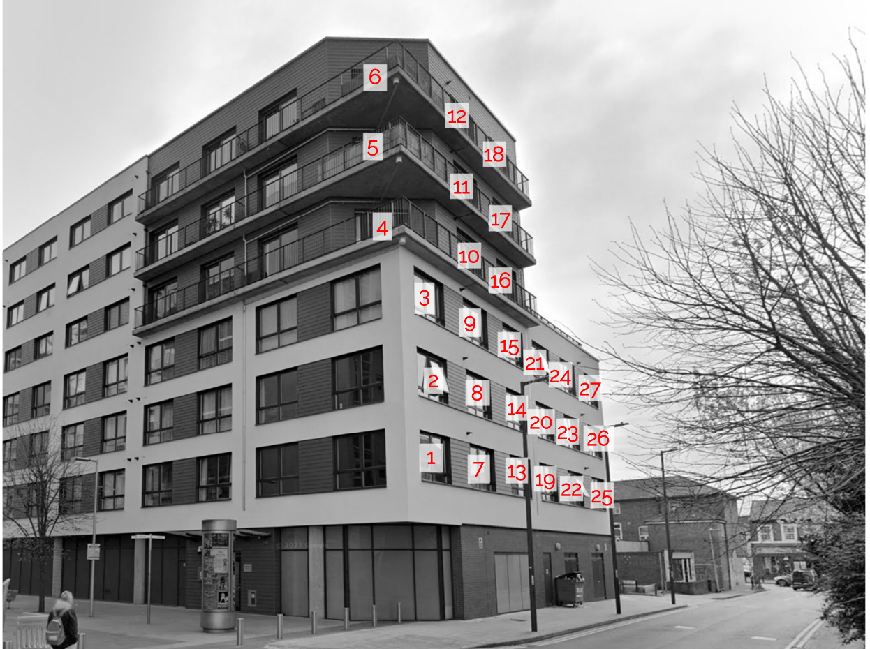
Mayer House – West Elevation
