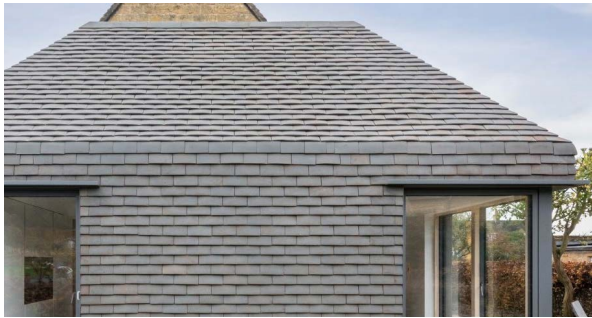
Precedent - slate mansard roof to wall transition.
