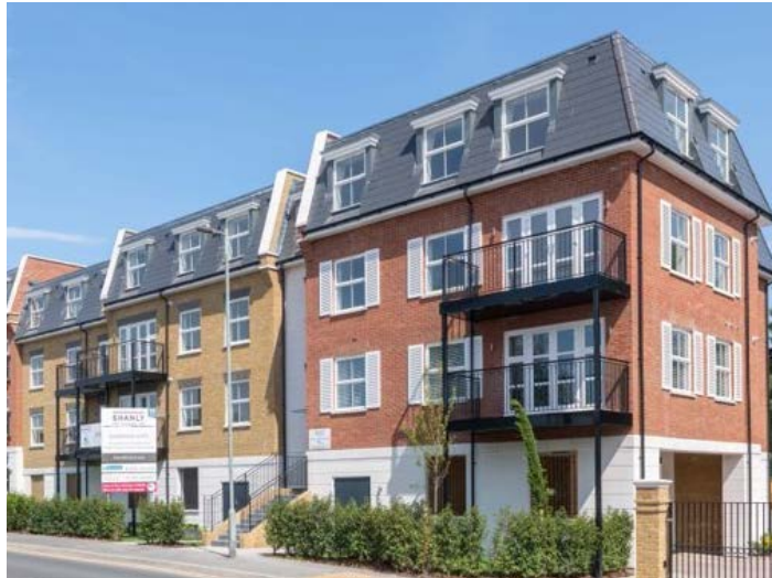
Elmwood Gate, Oldfield Road, Maidenhead
