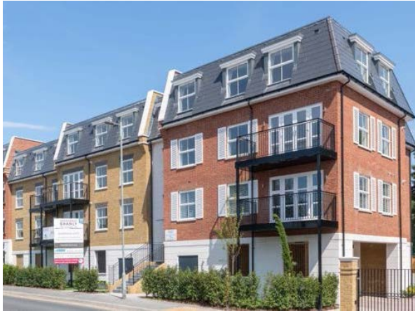
Sorbon Estate - Elmwood Gate with traditional mansard roof.
